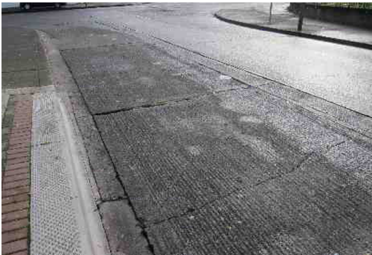
Rating 6: Transverse linear cracks of narrow width ( \leq 12\text{mm} ) and poor joint seal with grass growth
