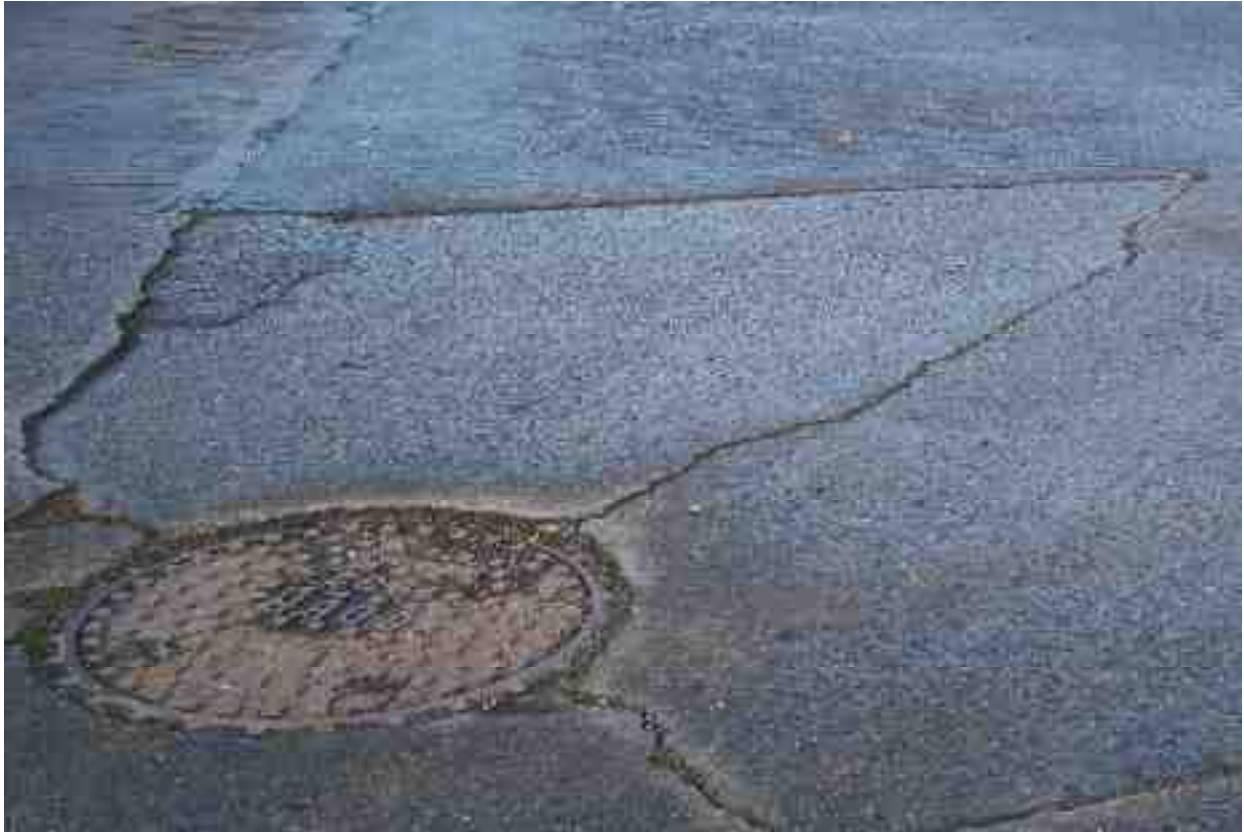
Cracking in vicinity of Manhole
