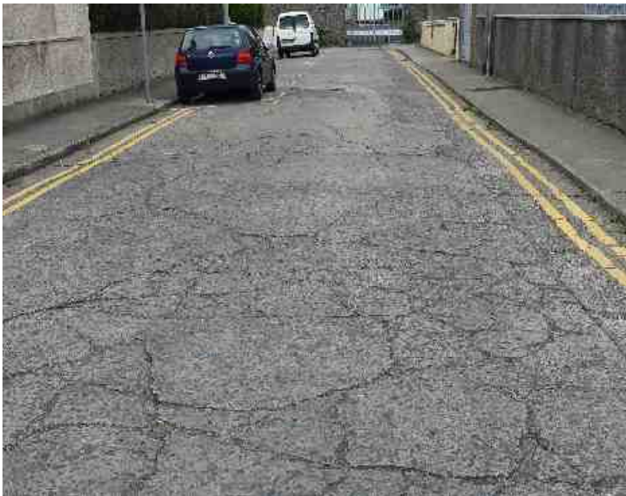
Rating 1: Failed slab with extensive cracking
