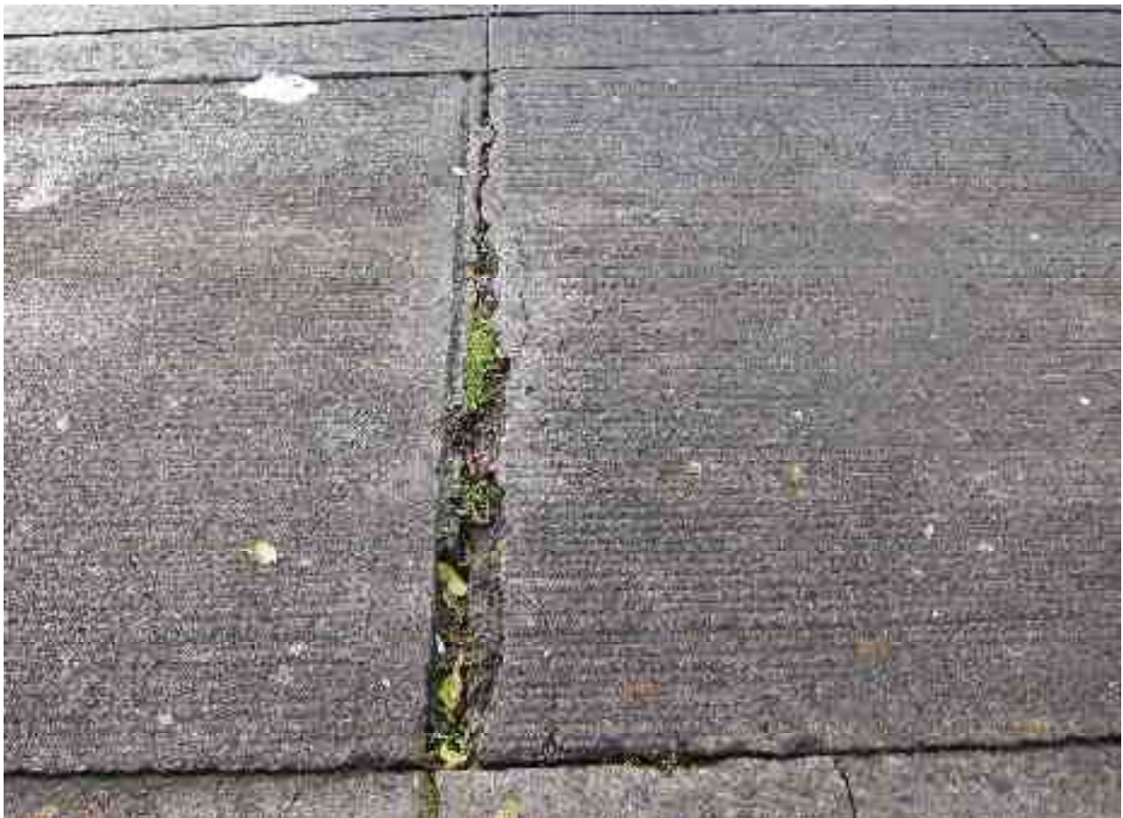
Severe Joint seal damage with joint eroded causing cracking and spalling
