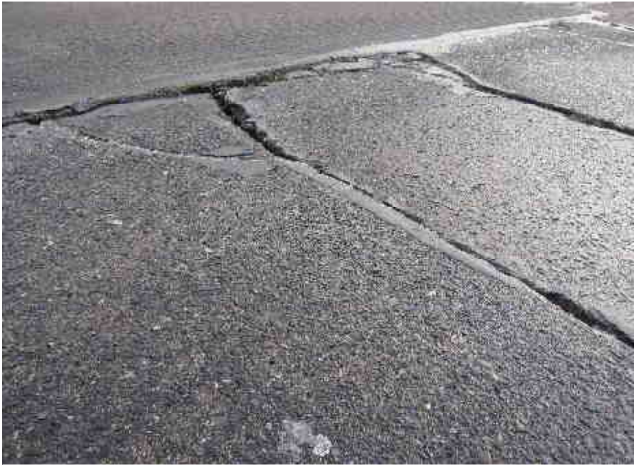
Wearing and polishing of aggregate over the surface, corner break and joint damage also evident
