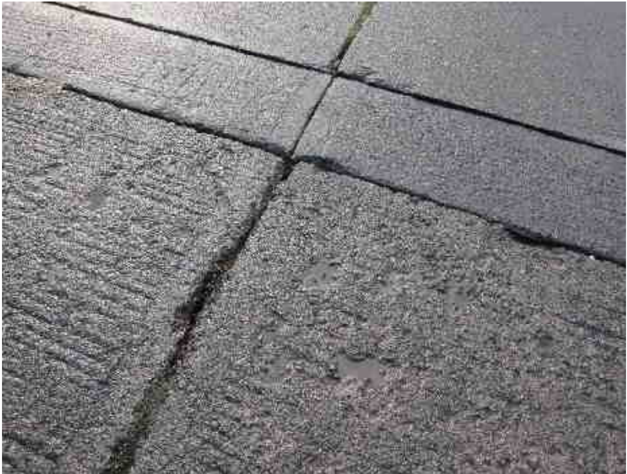
Scaling on concrete slab resulting in loss of surface, joint seal damage also evident
