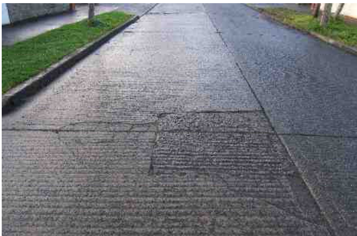
Rating 5: Multiple Corner breaks with broken pieces, crack width is narrow ( \leq 12 mm)
