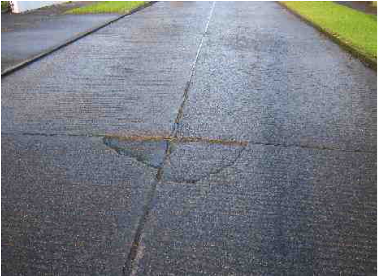
Corner Breaks on adjoining concrete slabs
