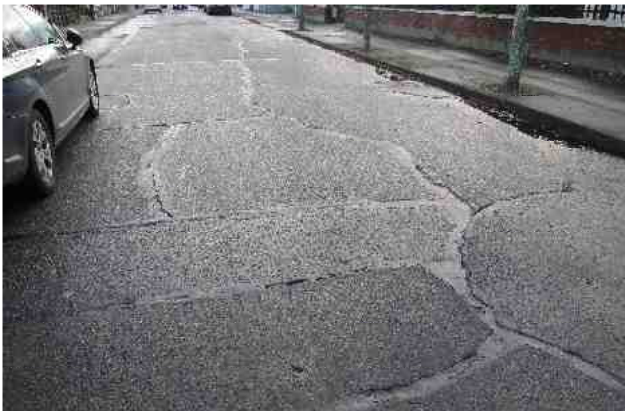
Rating 2: Extensive wide interconnecting cracking with poor sealant
