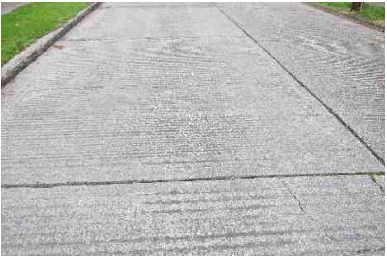
Rating 7: Good condition overall, a few isolated linear cracks (tight) present, partial joint seal damage
