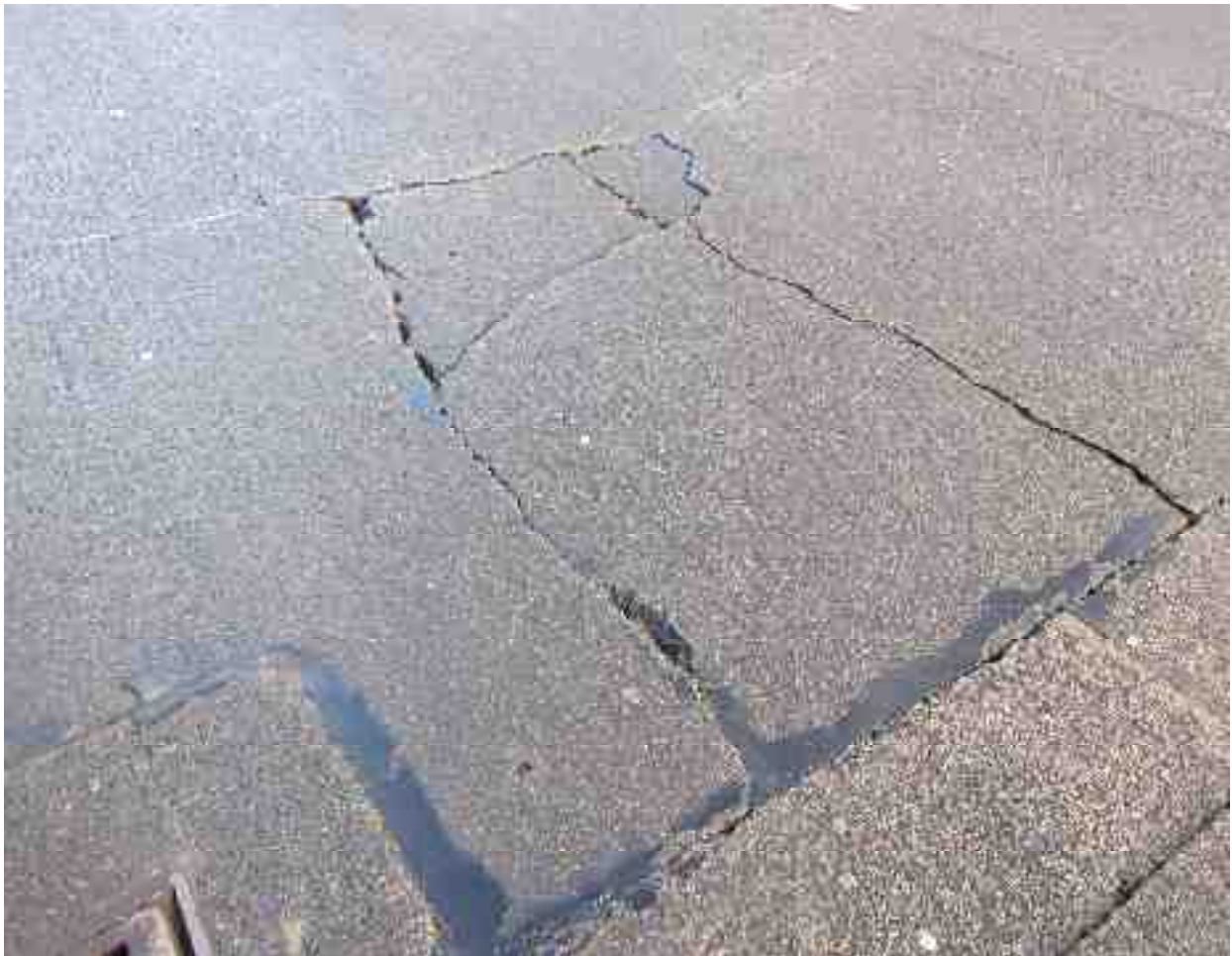
Shattered slab with movement and severe Faulting resulting in failed road surface
