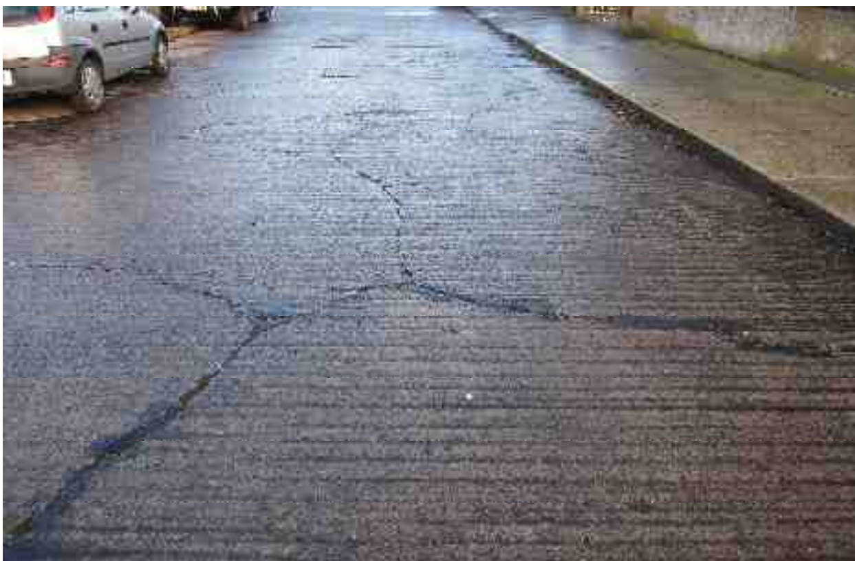
Rating 3: Shattered slab, wide cracks (>12mm) with very poor crack sealing
