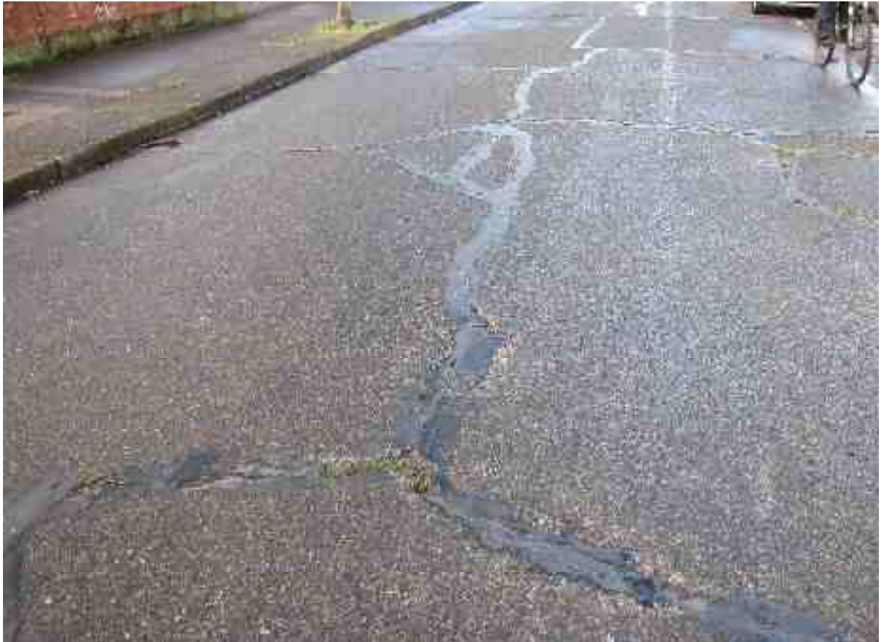
Wide and Poorly sealed cracks showing severe deterioration
