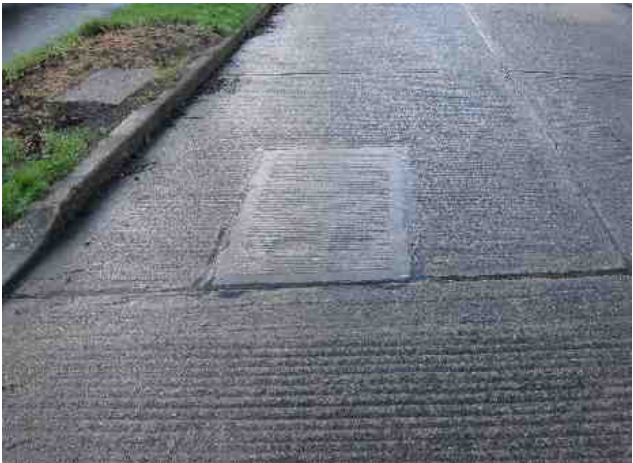
New Patch in very good condition with good sealant
