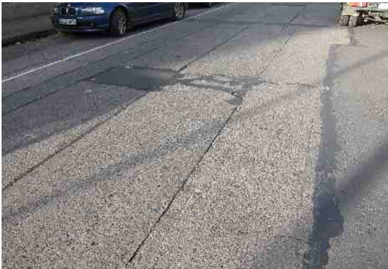
Rating 6: Transverse linear cracks (tight) with good patching and some wear
