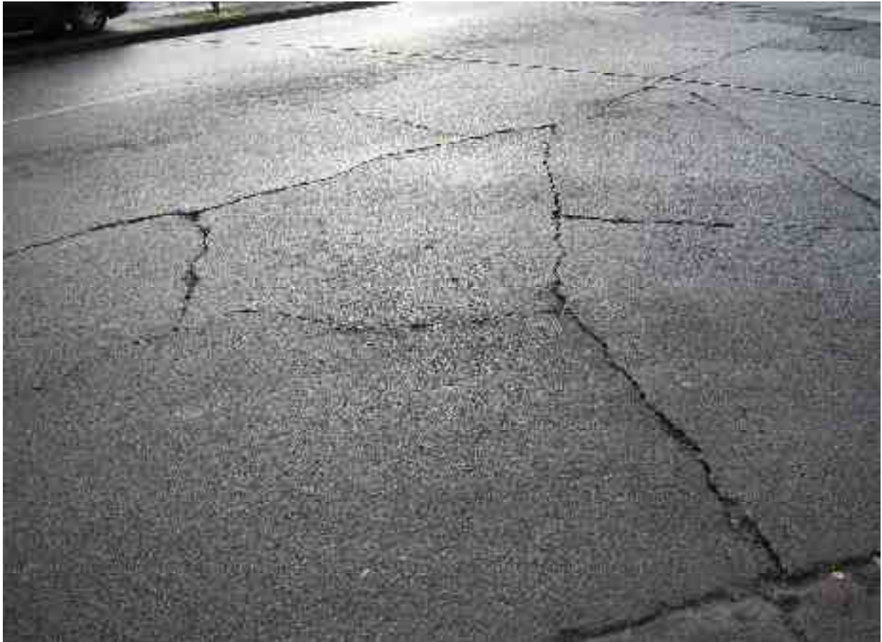
Shattered slab over large area
