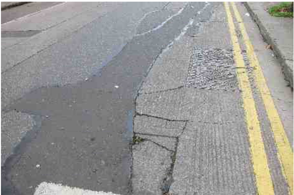
Cracking in vicinity of Manhole with asphalt utility patching
