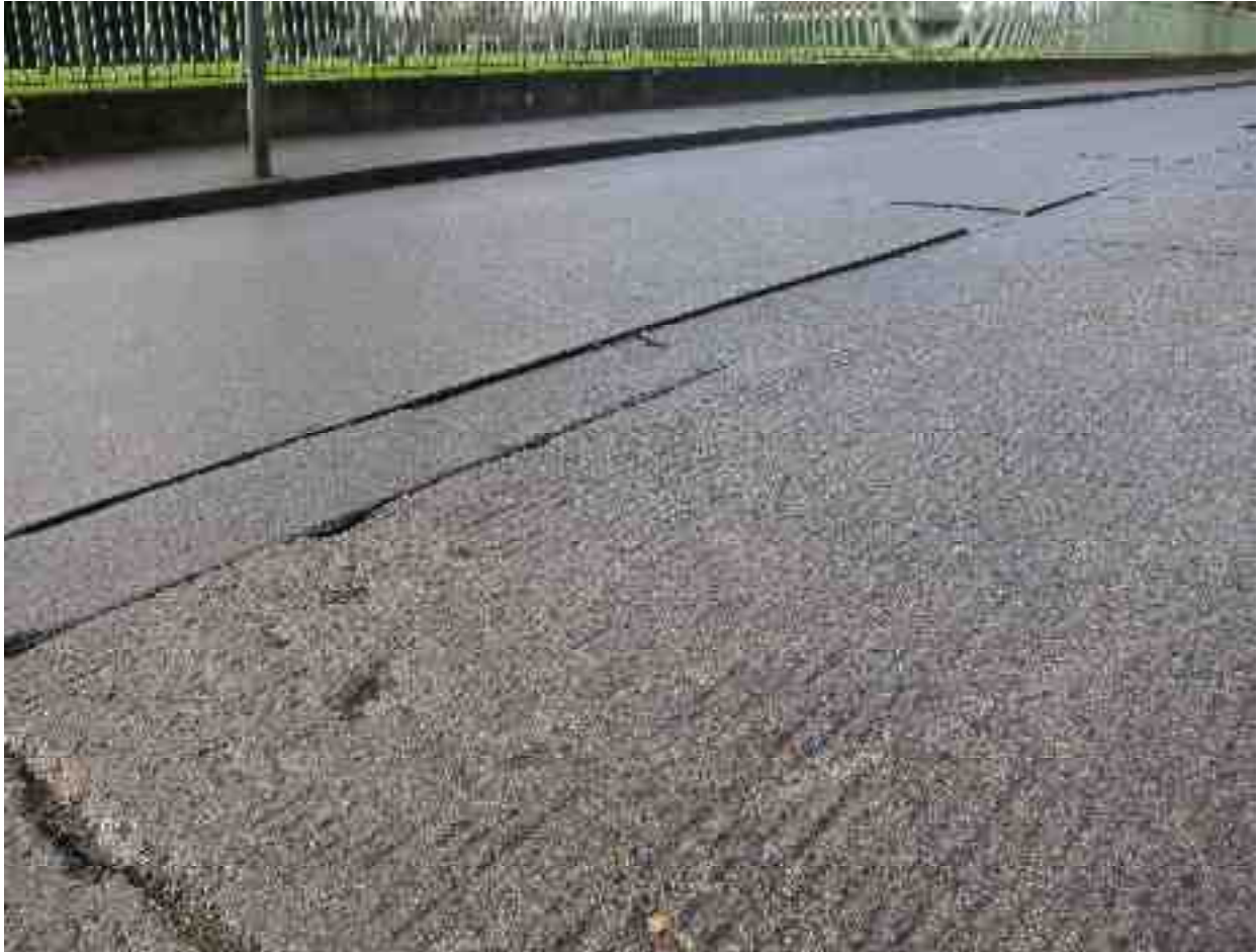
Faulting of slabs
