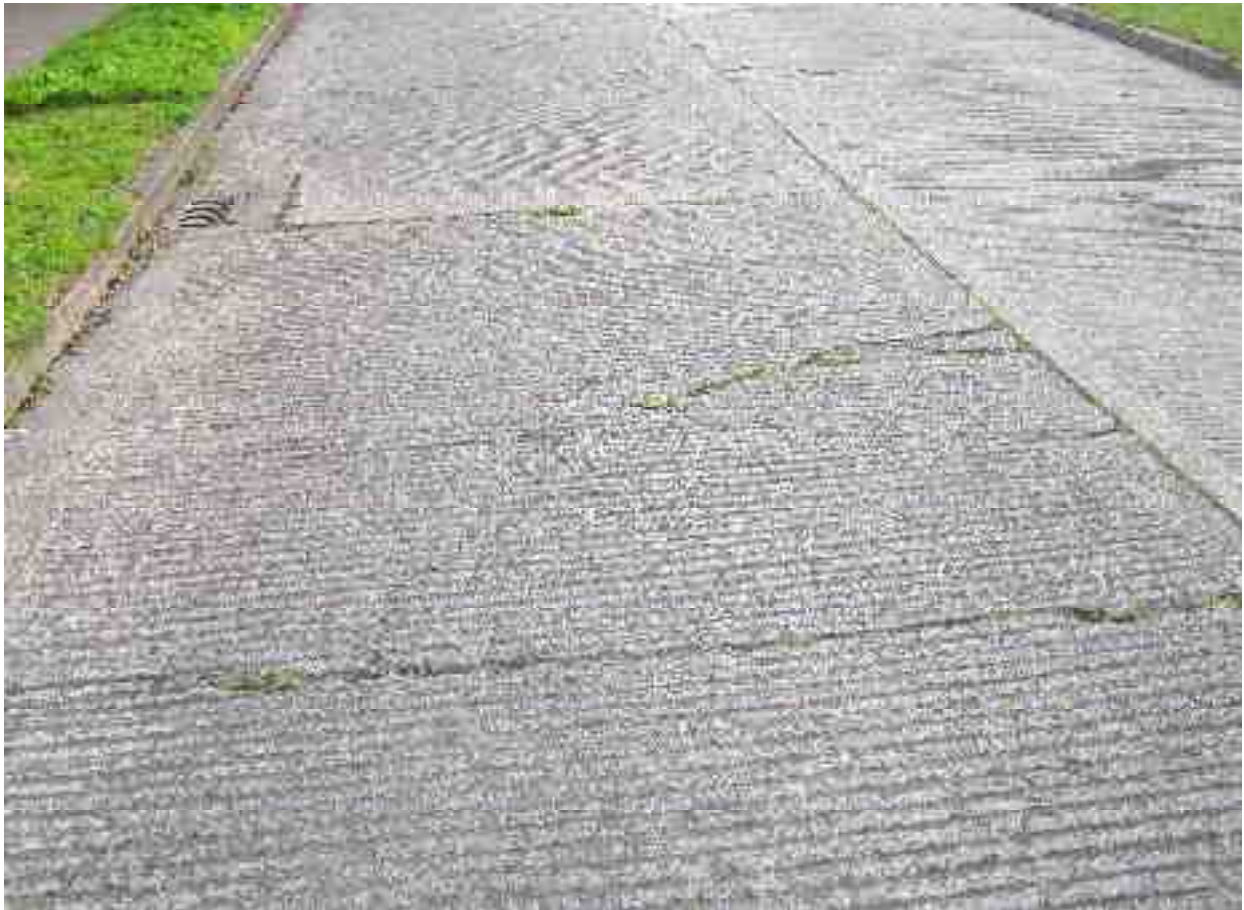
Longitudinal and Transverse cracks
