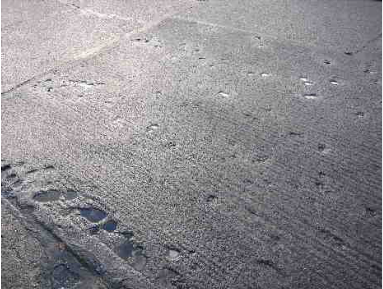
Pop-outs on concrete slab
