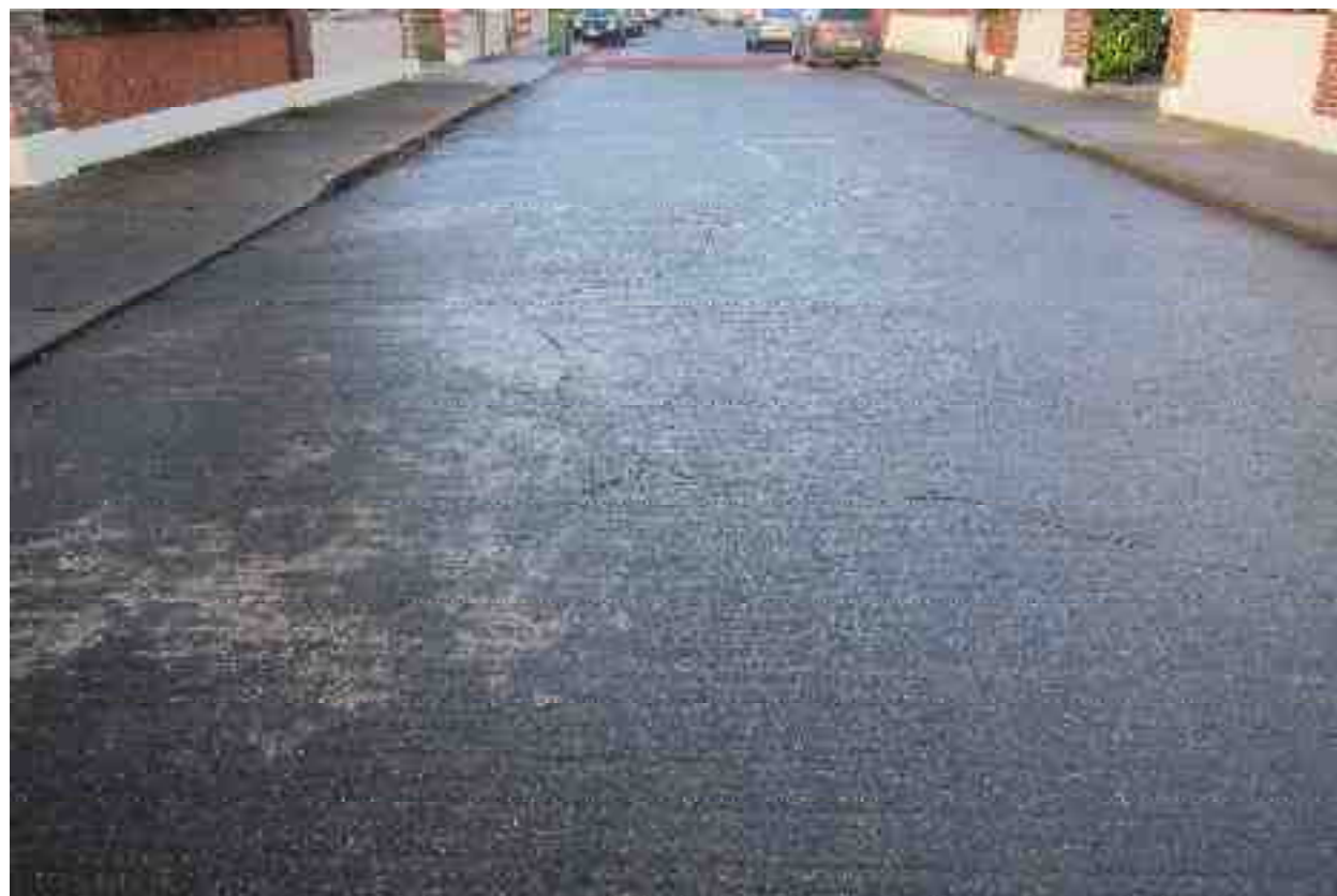
Rating 4: Extensive interconnecting linear cracking
