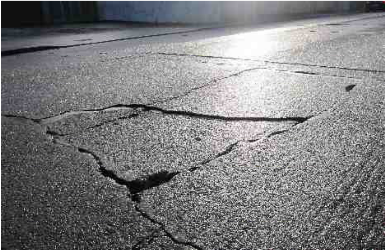
Rating 1: Extensive very wide cracks, severely shattered slab with severe faulting (>25mm) and spalling
