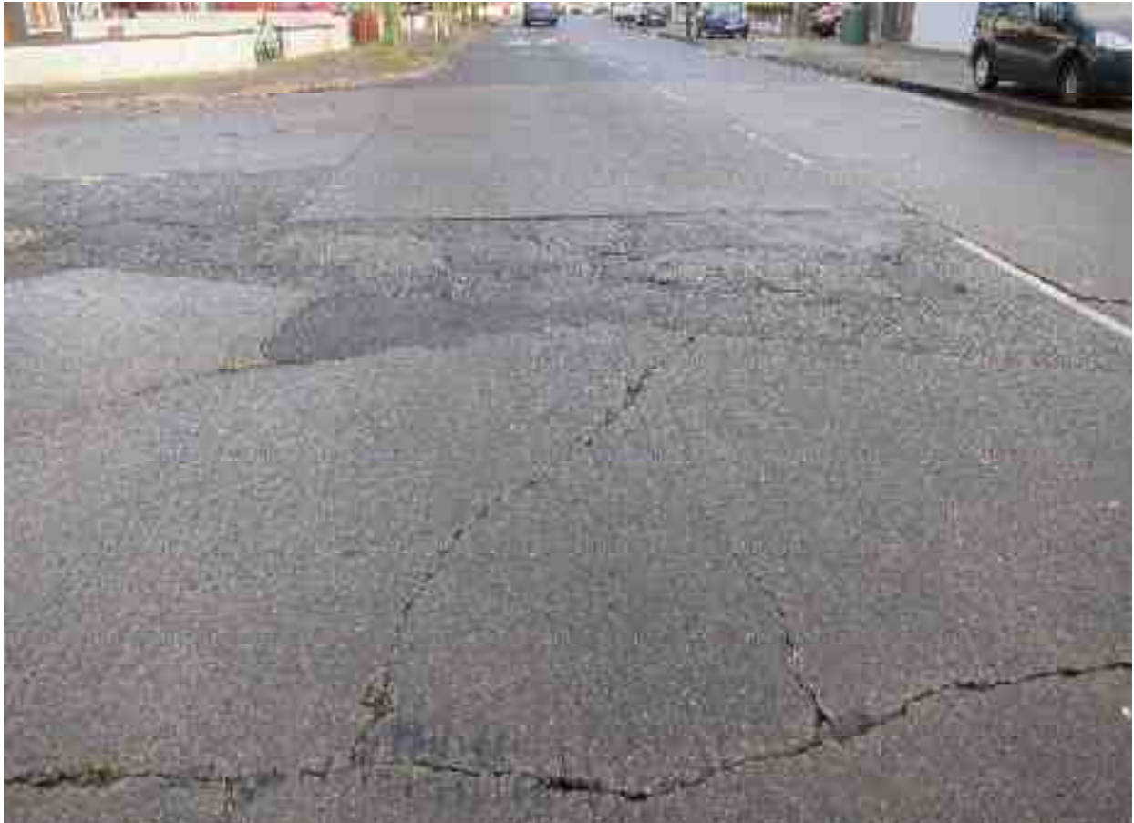
Poor patching in area of shattered slab
