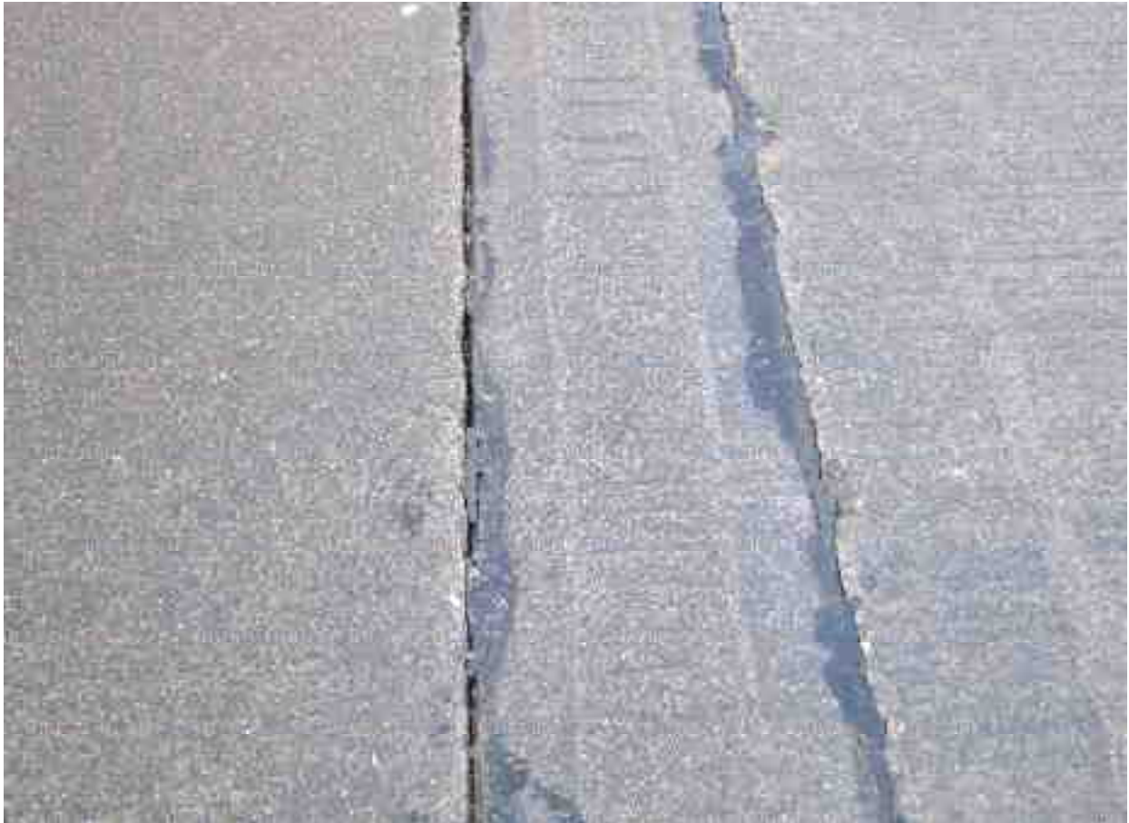
Joint seal damage with sealant almost completely removed
