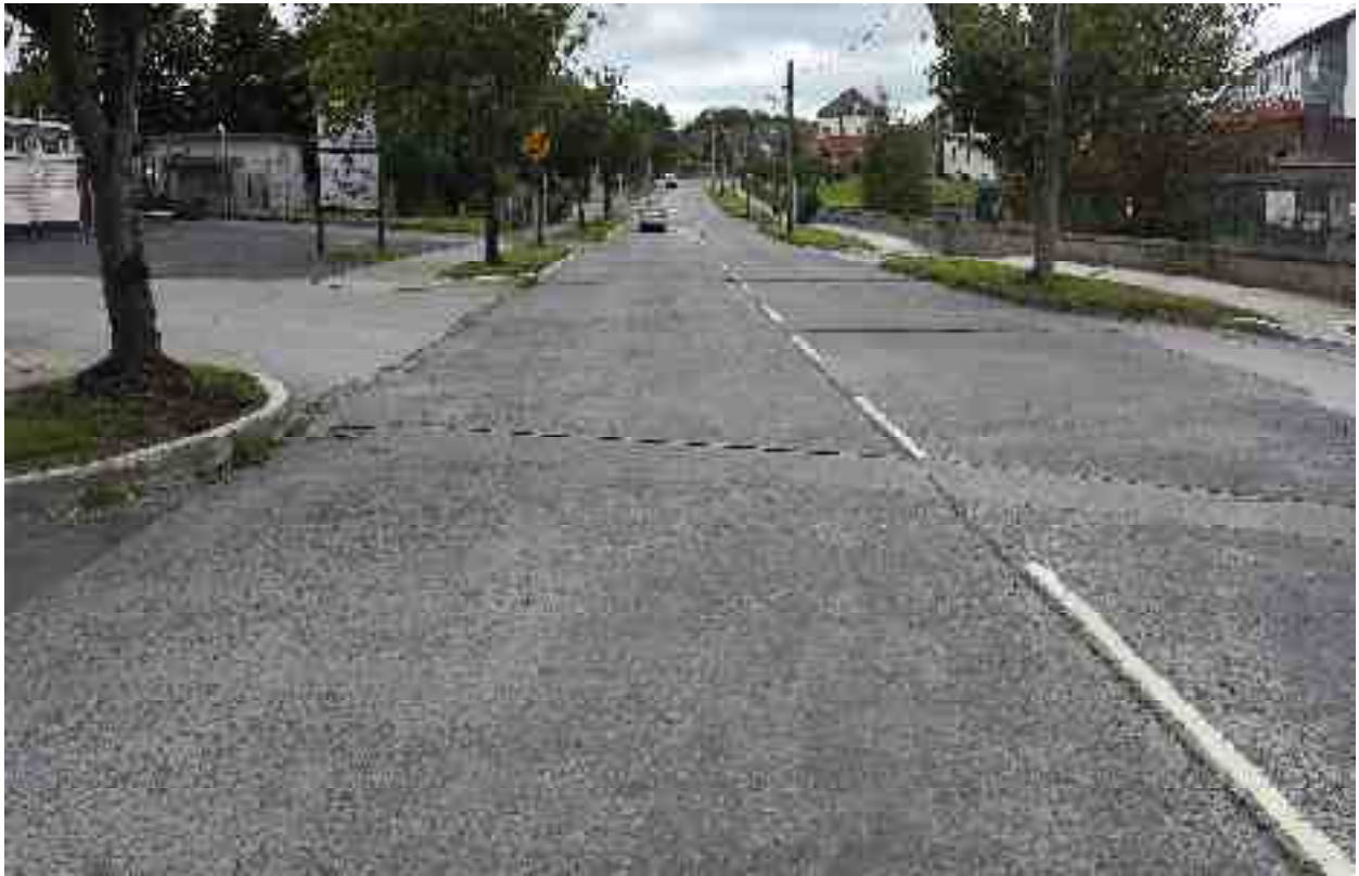
Rating 7: Greater than 30% Wear and Polishing present. Isolated utility cut in good condition
