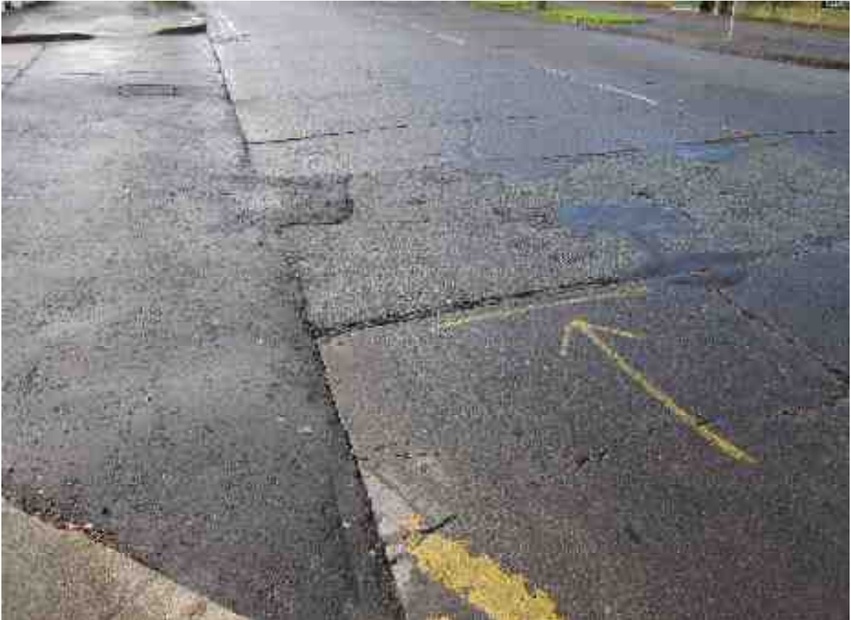
Deteriorated asphalt patching in poor condition on concrete surface
