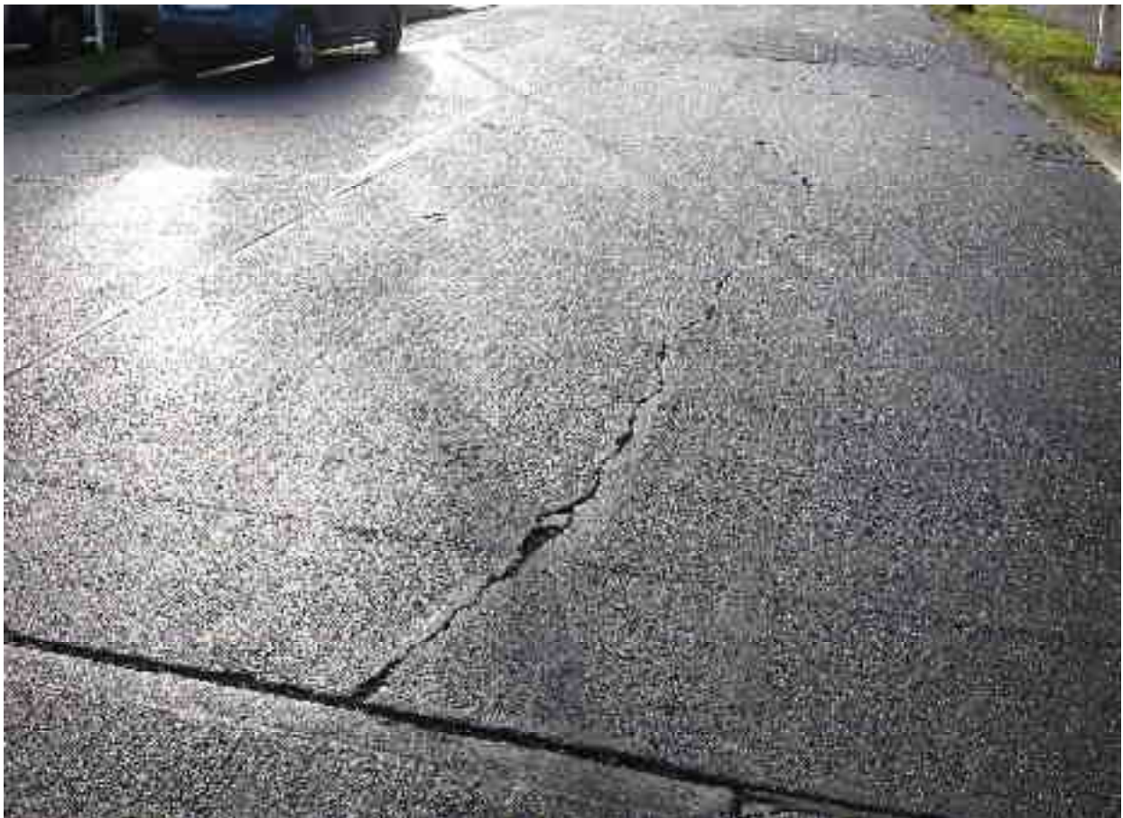
Longitudinal open crack along concrete slab with no sealant
