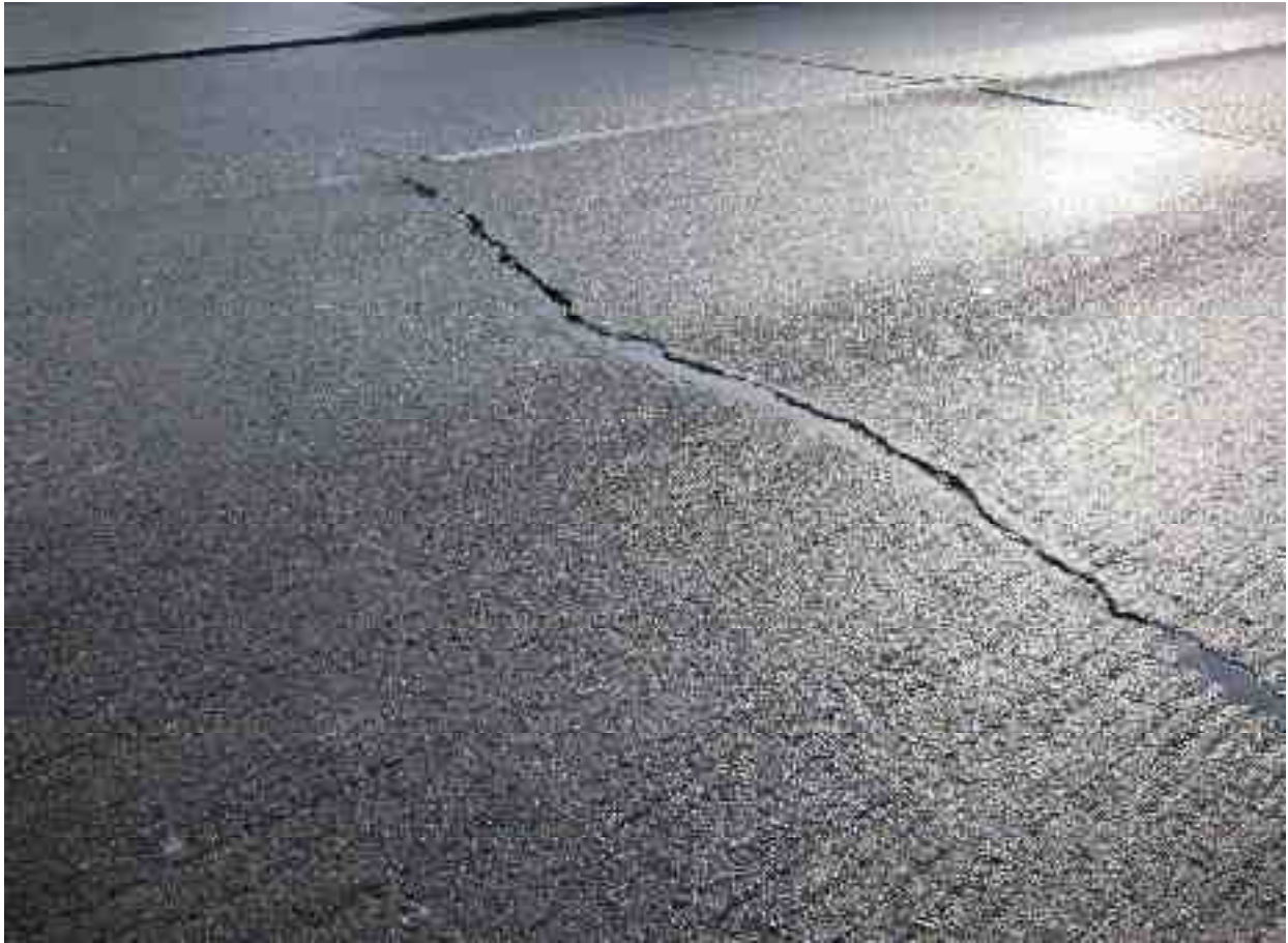
Transverse cracks across carriageway open > 12mm and with poor sealant
