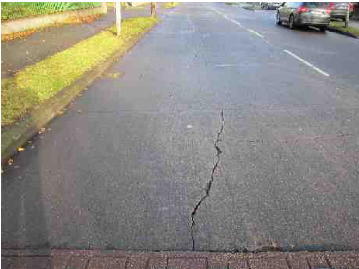
Rating 4: Severe unsealed cracks greater than 12mm wide with spalling present
