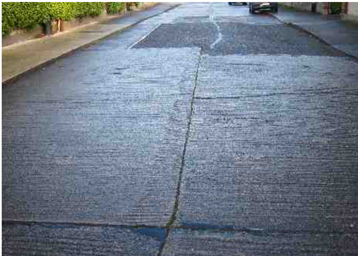
Rating 5: Large Patching in fair condition and linear narrow cracks present
