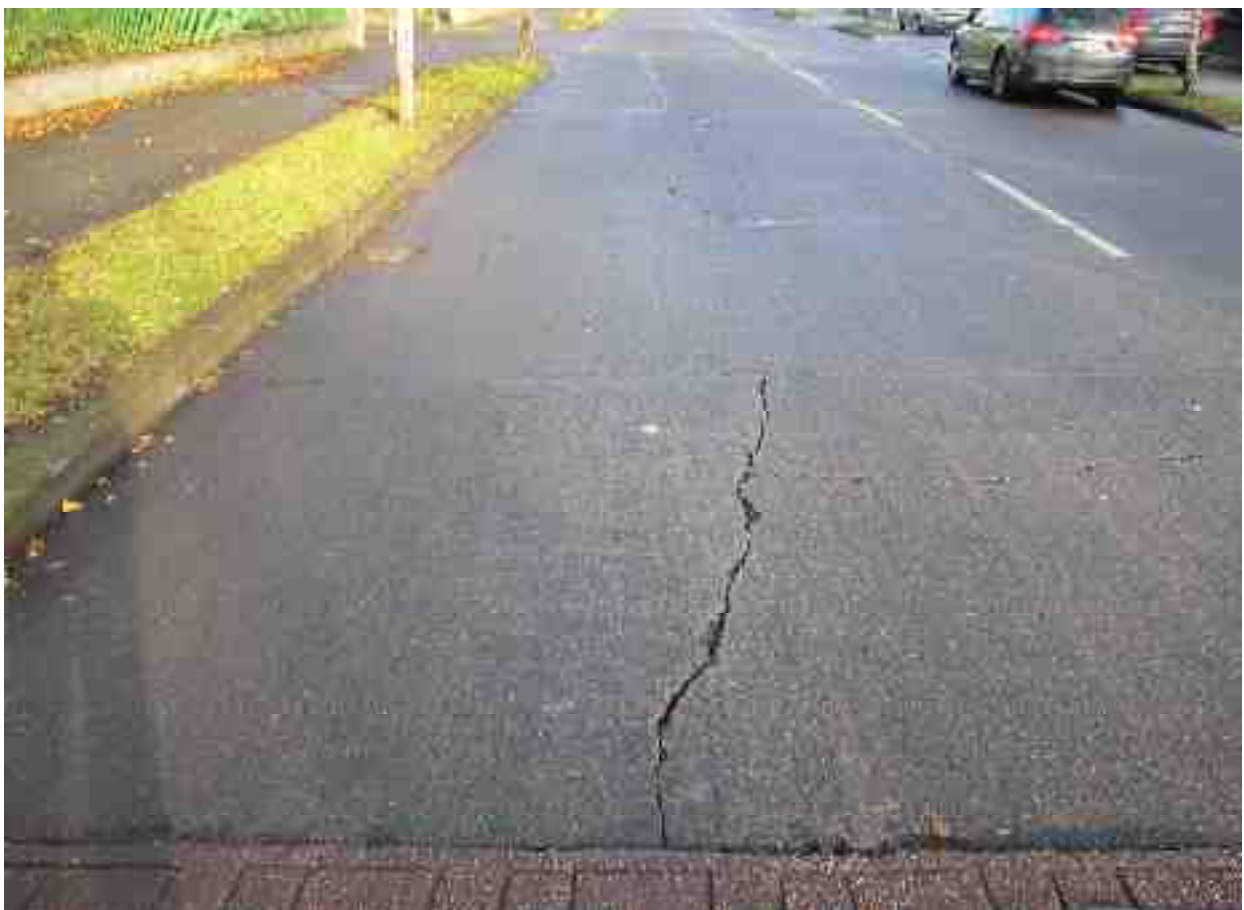
Longitudinal and Transverse wide open cracks
