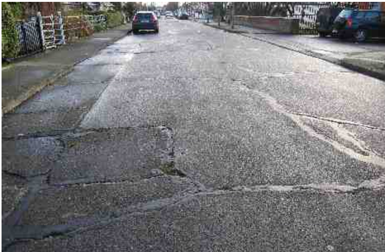
Rating 2: Large quantities of wide and open cracking with very poor sealant
