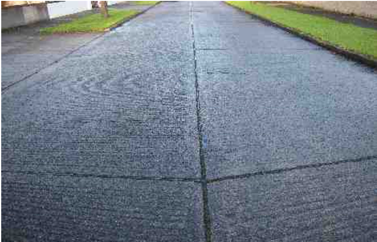
Rating 8: Good condition, First isolated tight Linear crack evident, partial joint seal damage
