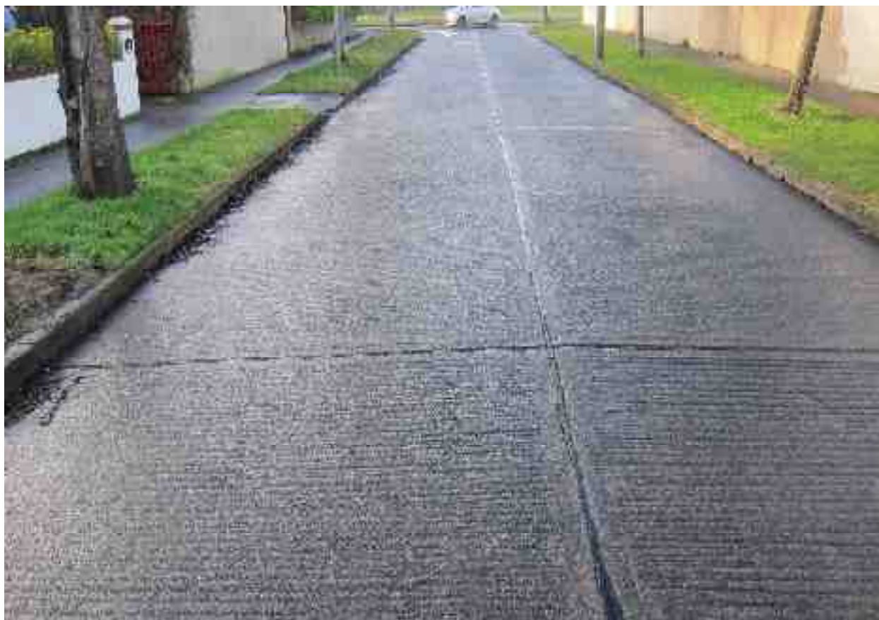
Rating 10: New Pavement, no visible defects
