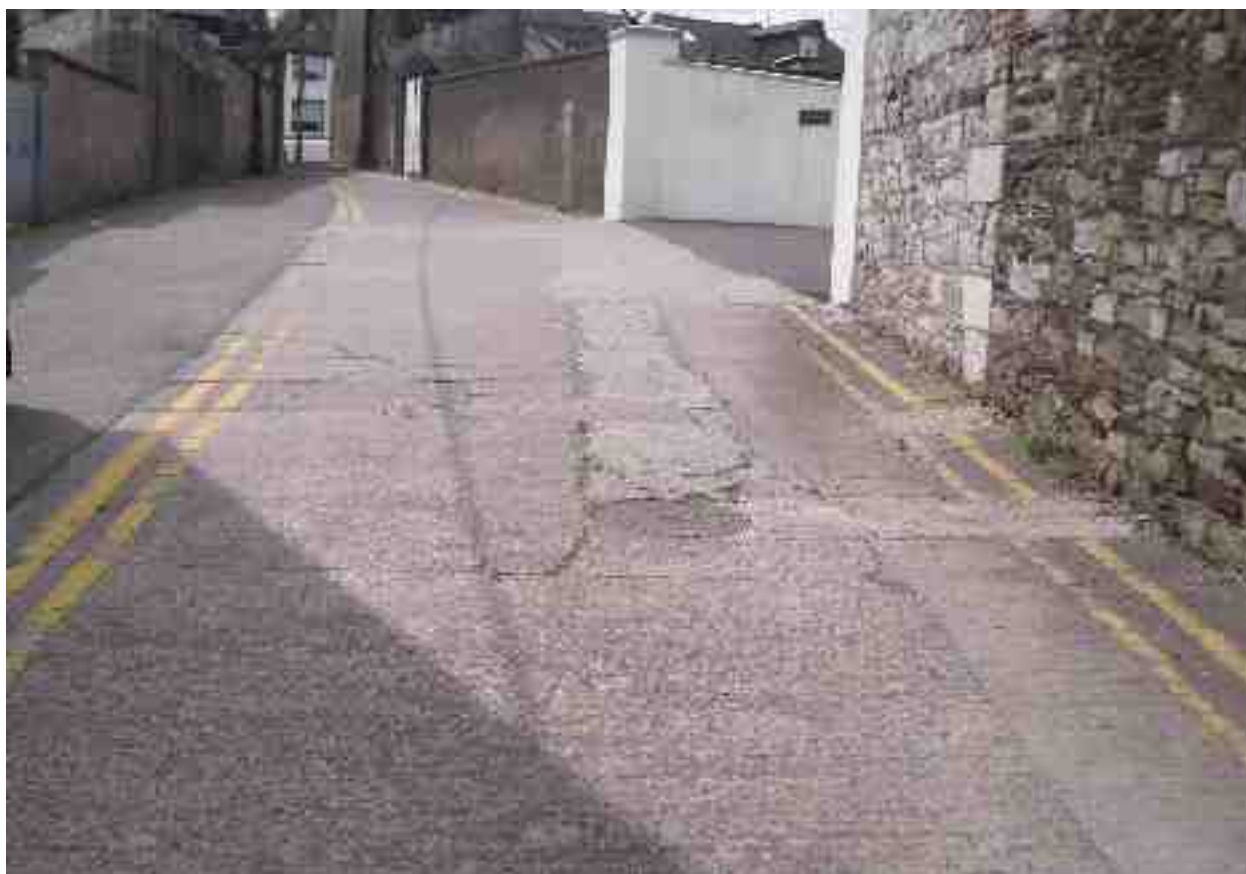
Rating 5: Fair patching, more frequent linear cracks and utility cracks (all narrow)
