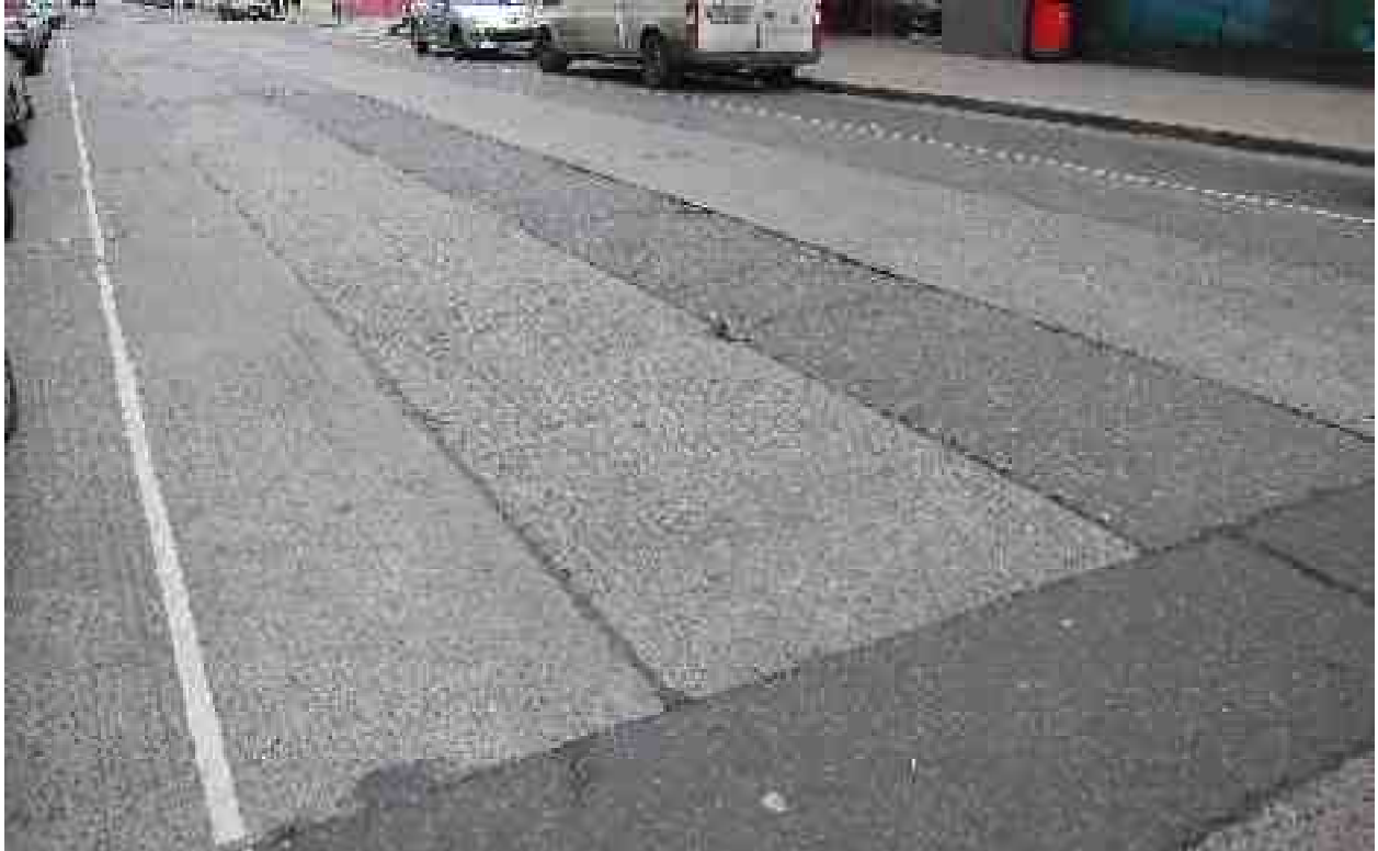
Rating 6: Utility cut patching generally in good condition, some wear and polishing
