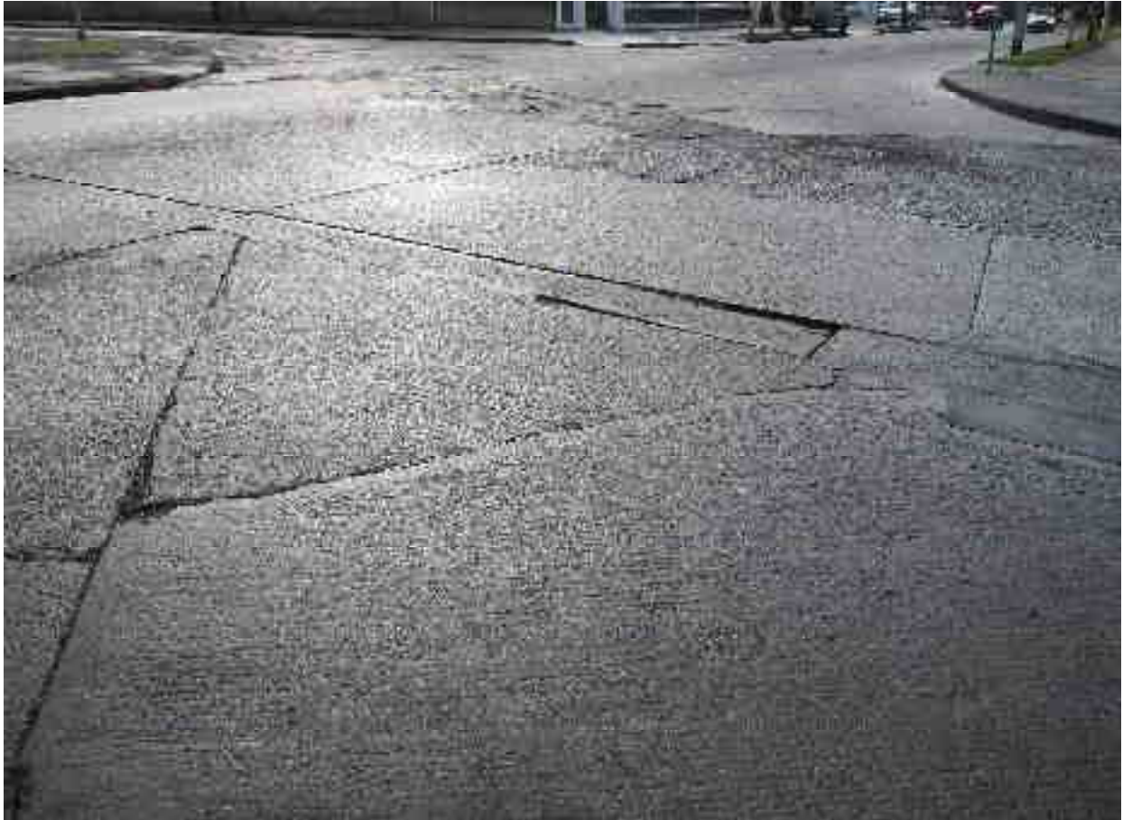
Faulting resulting in lip protruding from road surface
