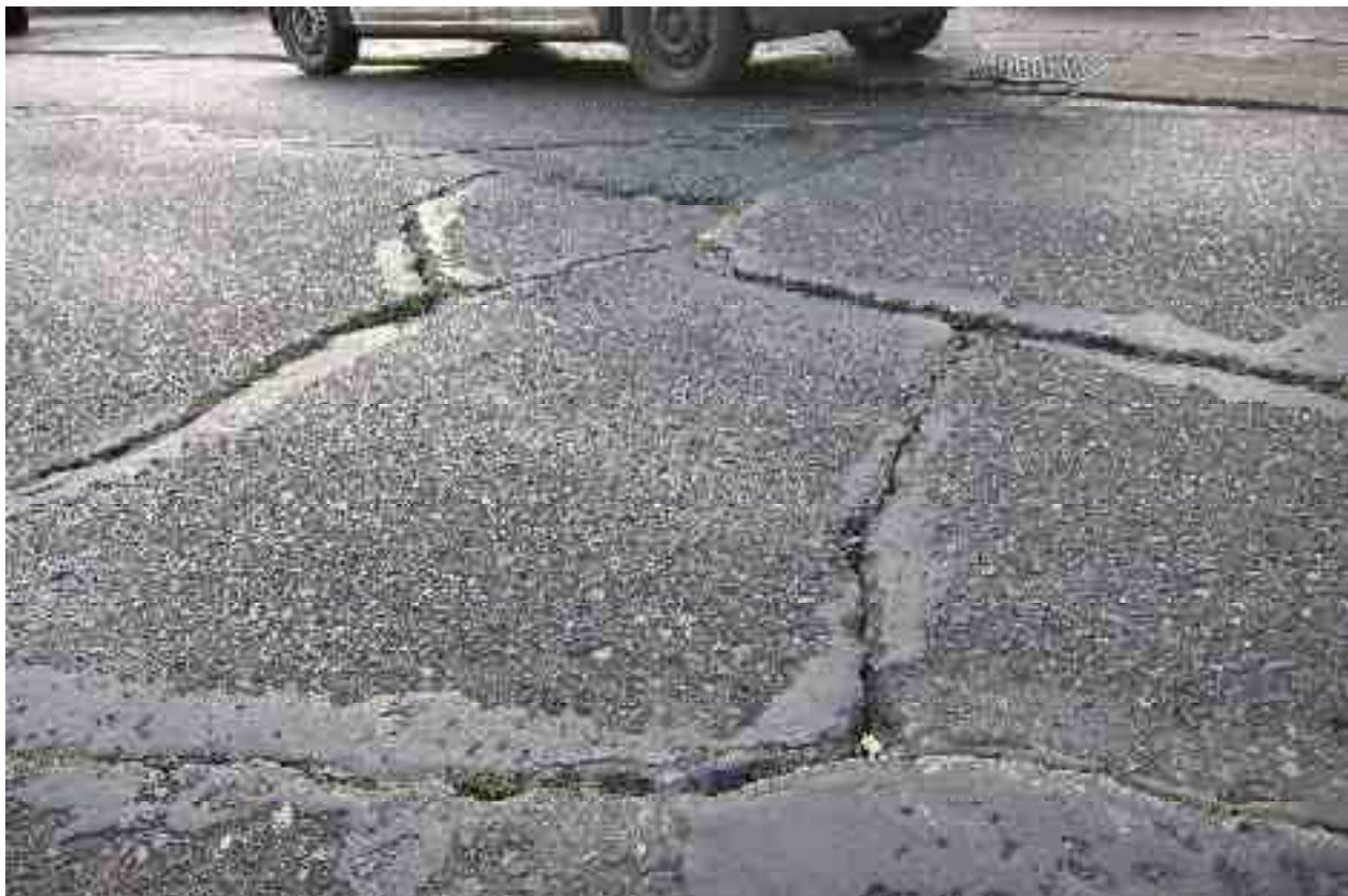
Rating 1: Shattered slab with spalling and grass growth, very wide cracks and very poor crack sealing
