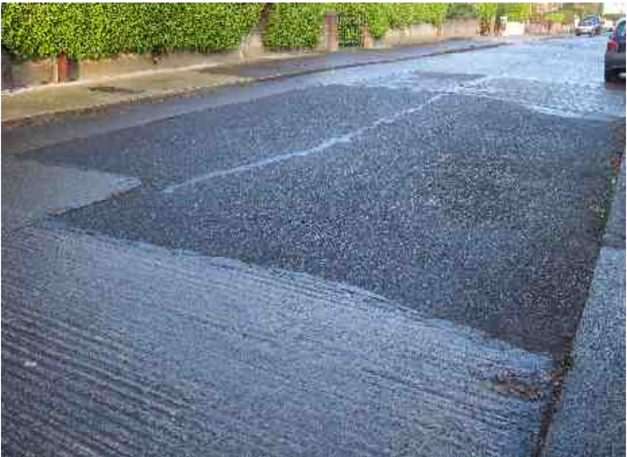
Moderately deteriorated asphalt patching in fair condition on concrete surface
