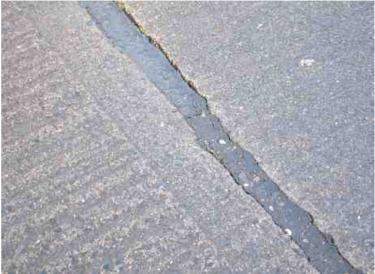
Wide Longitudinal joint with deteriorated joint sealing
