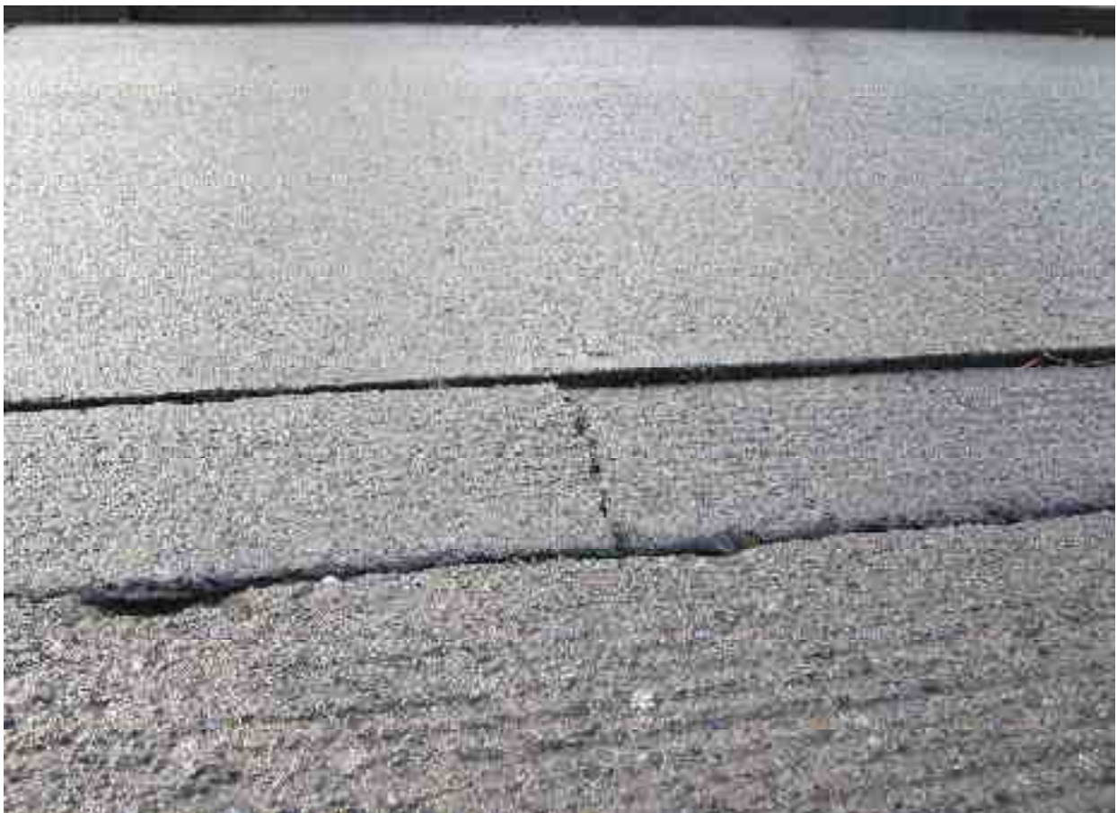
Severe Faulting (> 25mm) along joint
