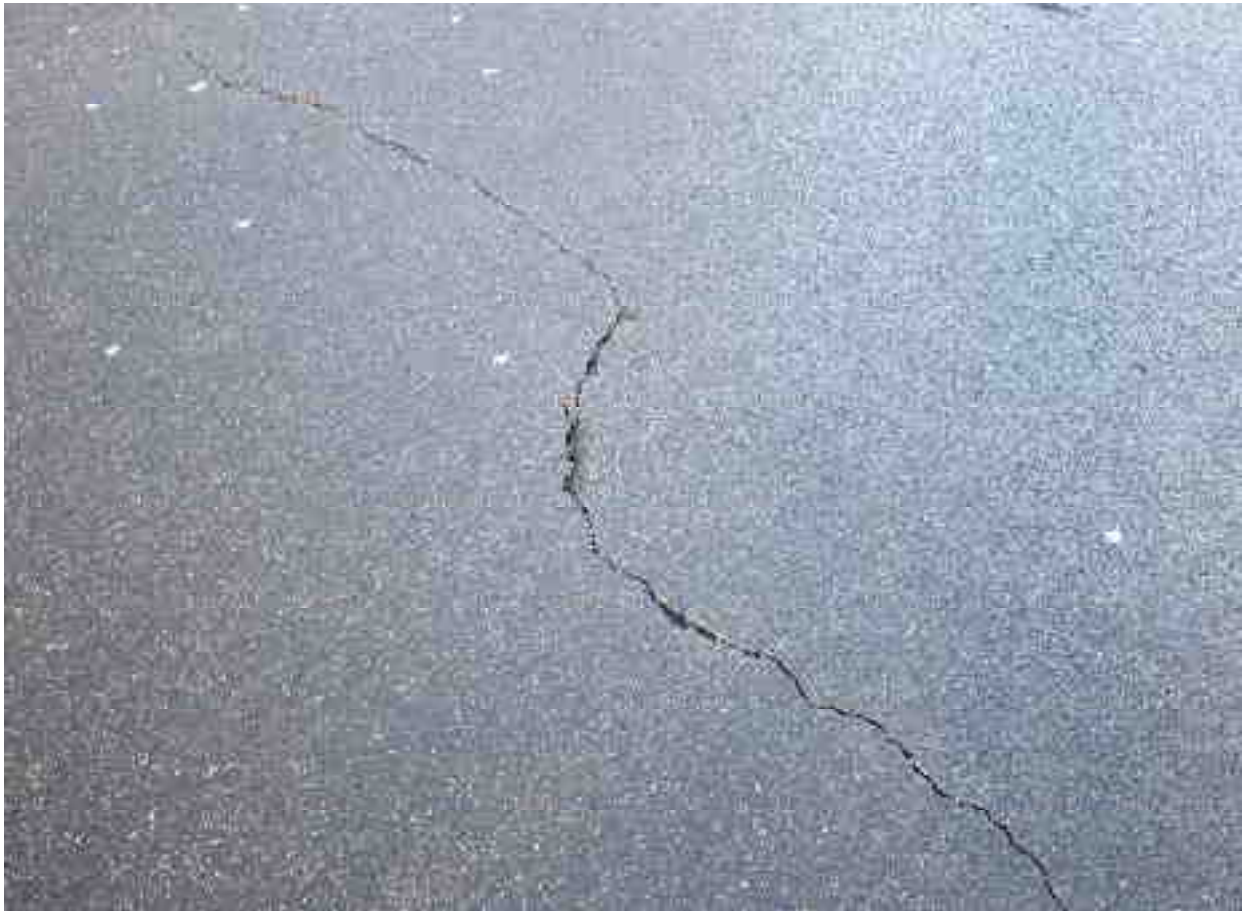
Meander crack, open and with no sealant, and with spalling evident
