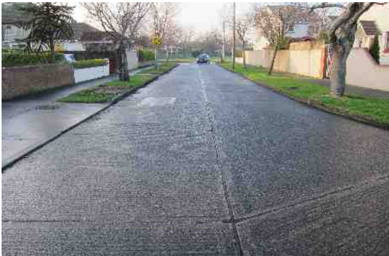
Rating 9: Small Patch in good condition, a few isolated tight Linear cracks present
