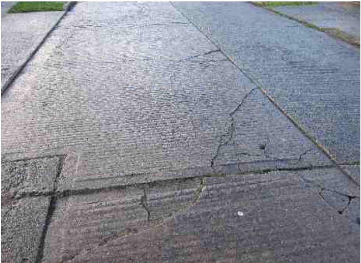
Extensive Corner Breaks
