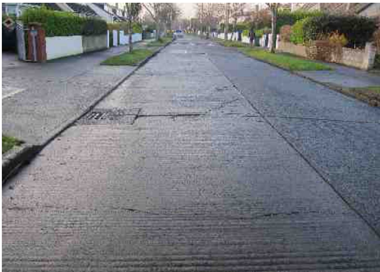
Rating 5: Several slabs with Corner breaks, Linear cracking (non-filled \leq 12\text{mm} ) and some spalling evident
