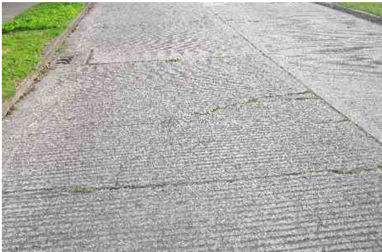
Rating 5: Corner breaks with minor faulting and spalling present, cracks are \leq 12 mm wide
