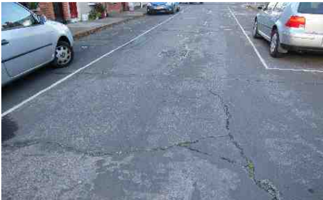
Rating 3: Extensive wide cracking (> 12mm) with spalling and very poor joint sealant
