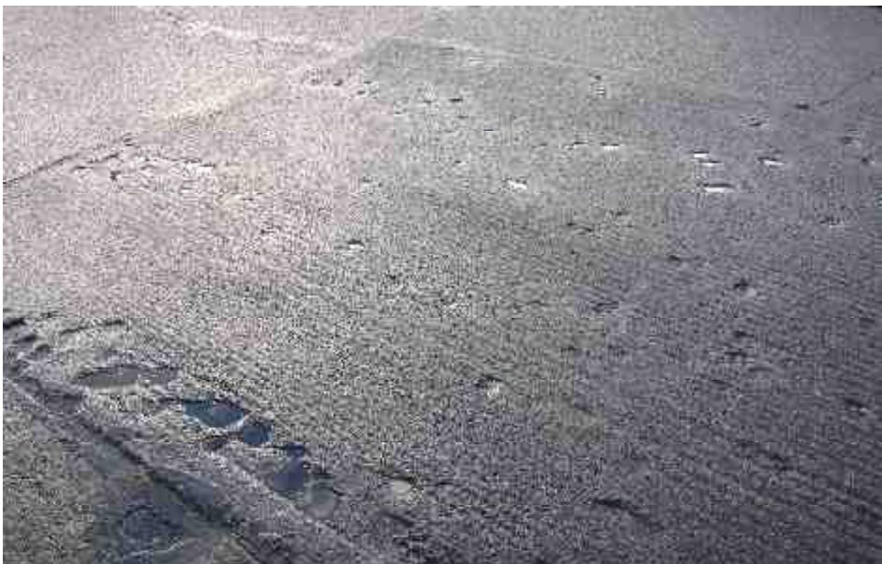
Rating 8: Surface defects - Pop-outs over 10 to 30% of area
