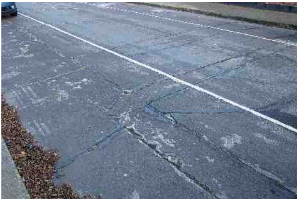
Rating 4: Multiple interconnecting linear cracks present with sealant in poor condition.
