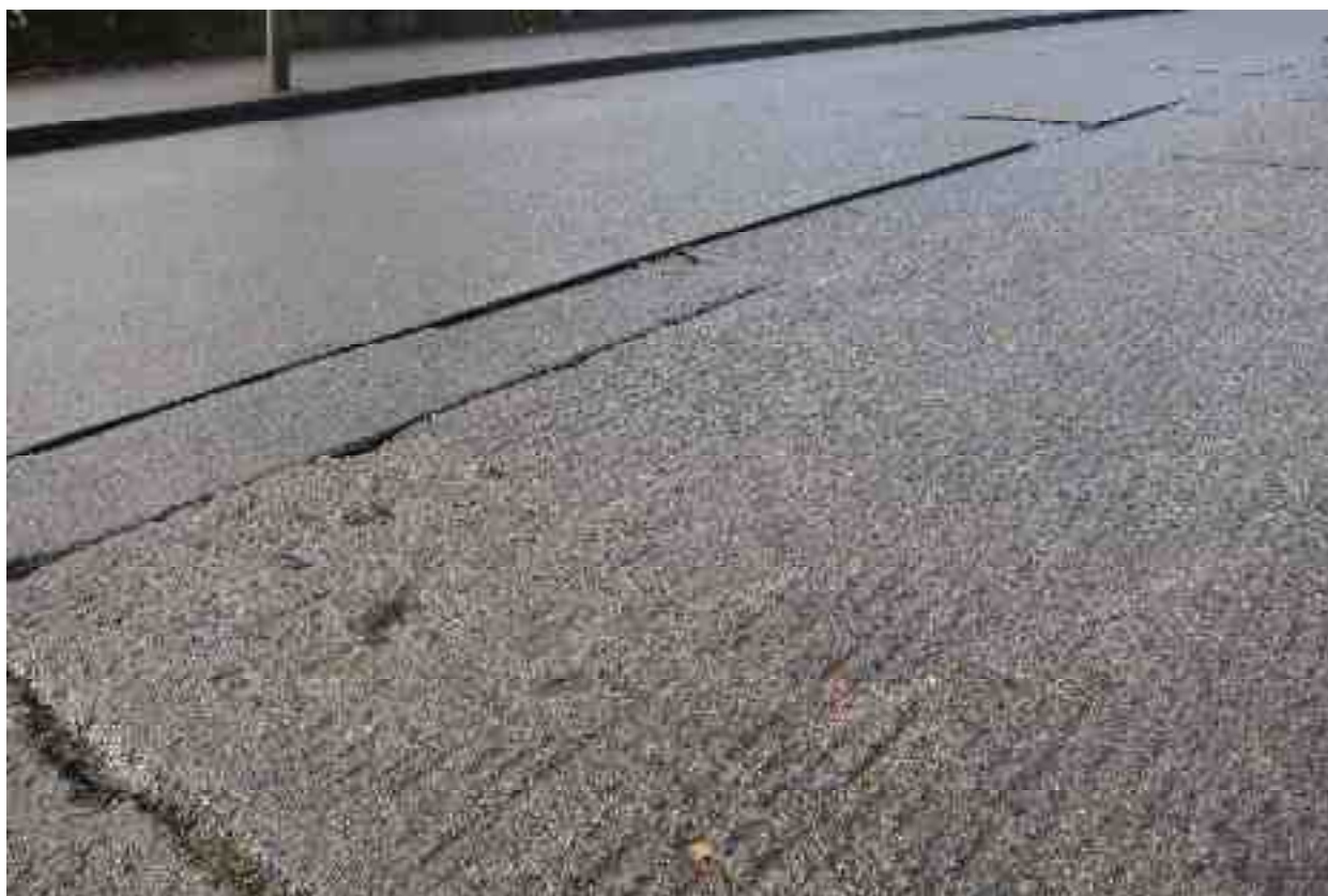
Rating 3: Severe faulting and surface deterioration present, very poor joints
