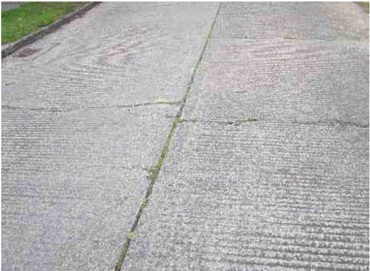
Wide Longitudinal joint with deteriorated joint sealing
