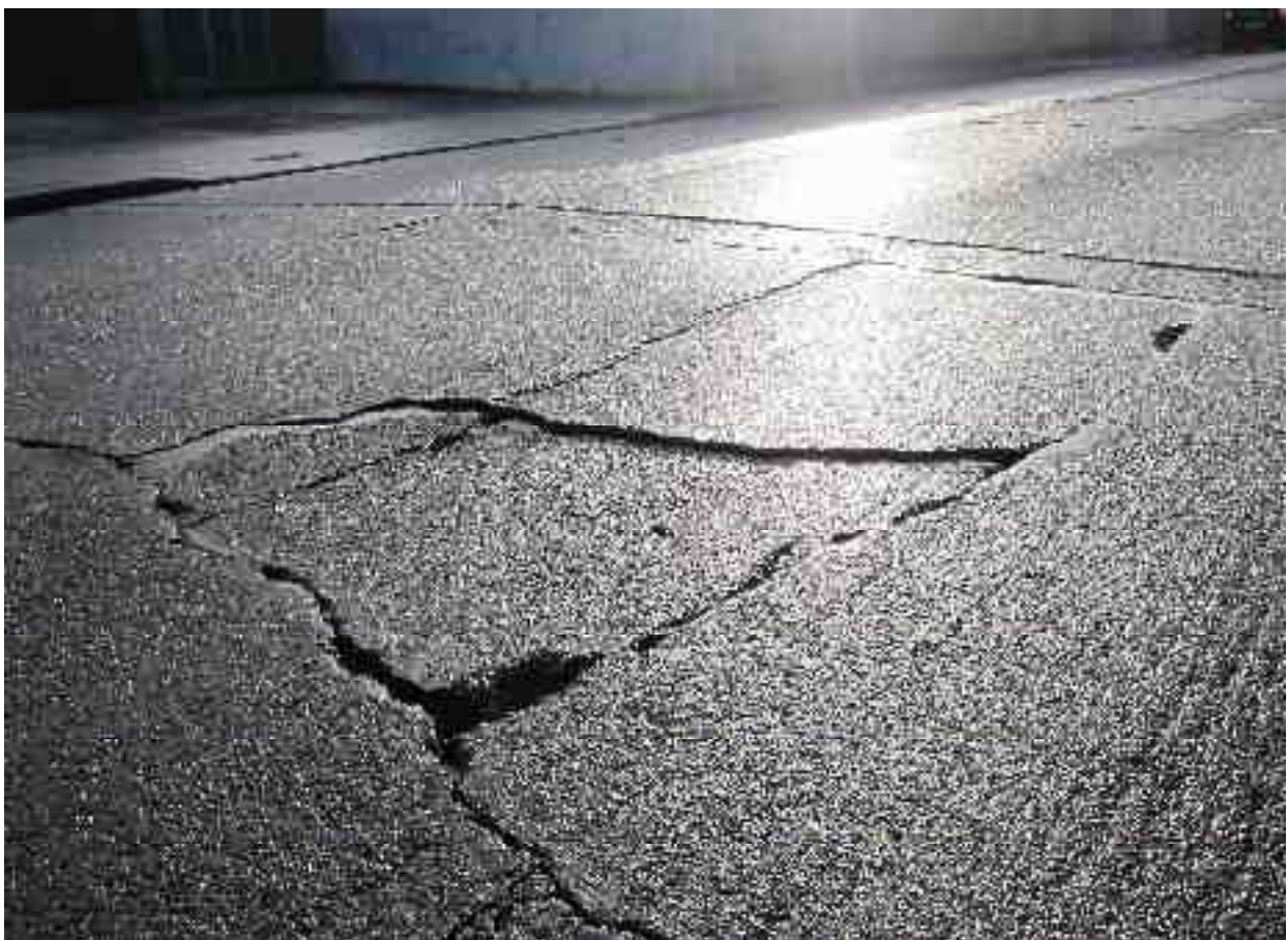
Failed Pavement: Severely Shattered Slab with severe Spalling and Faulting (> 25mm)
