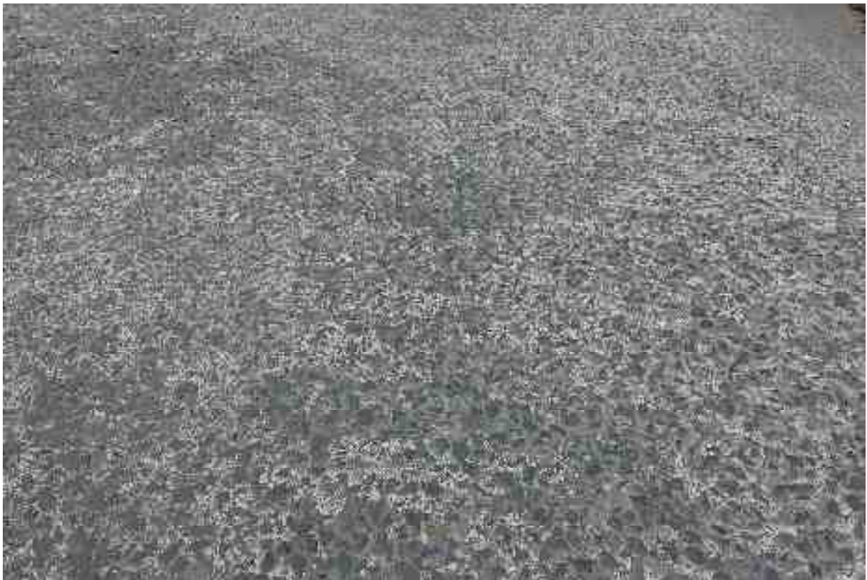
Wearing and polishing of aggregate evident over surface of concrete slab
