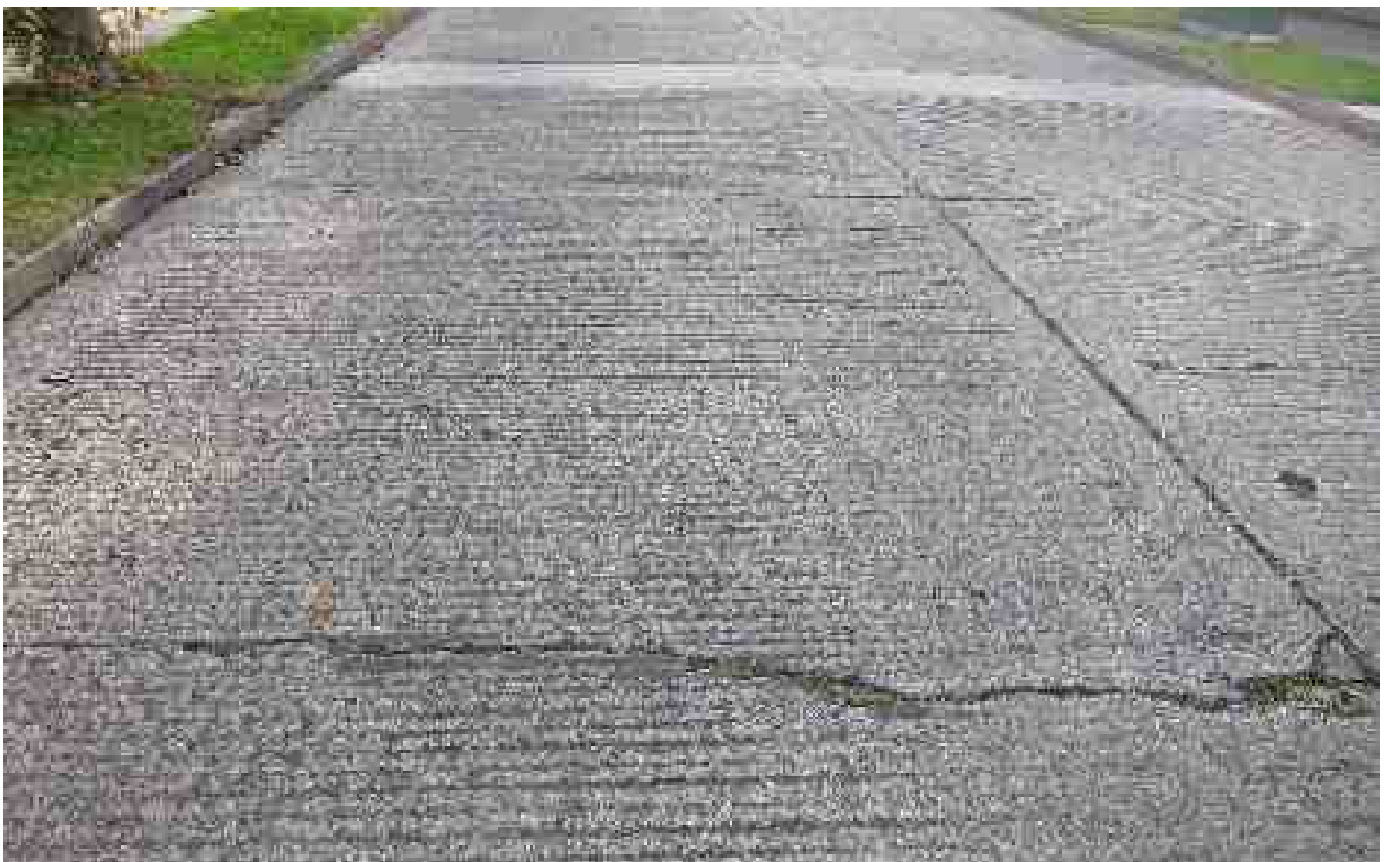
Rating 6: Open Linear cracks and Corner breaks present, Patching and utility cut repairs in good condition
