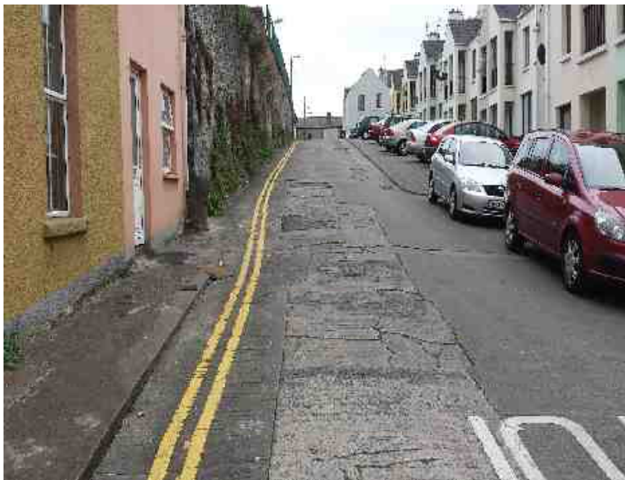
Rating 2: Extensive Shattered slab with no sealant present
