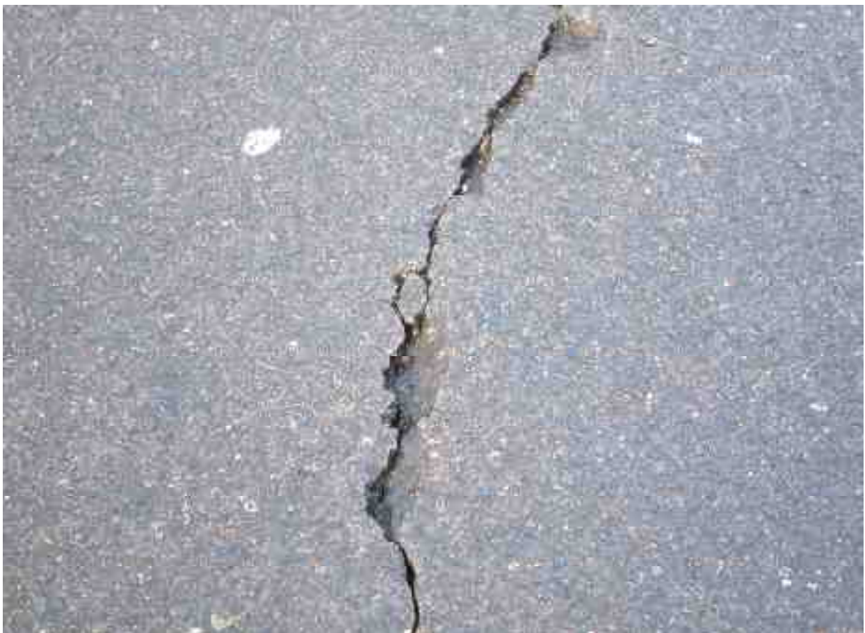
Spalling along edge of wide crack resulting in loss of large pieces of concrete
