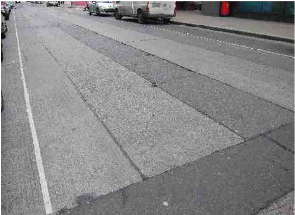
Asphalt Utility patching in centre of concrete pavement
