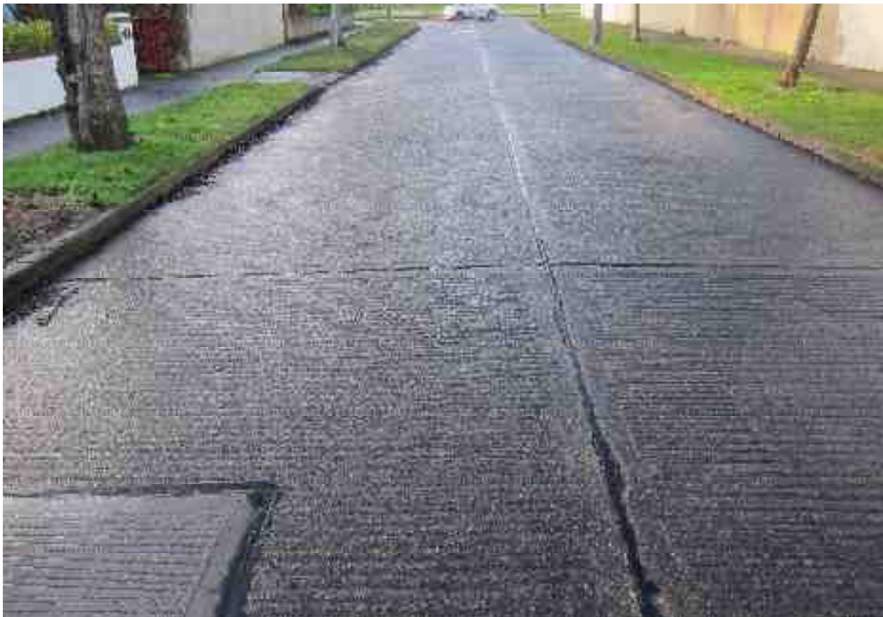
Joint sealant in excellent condition
