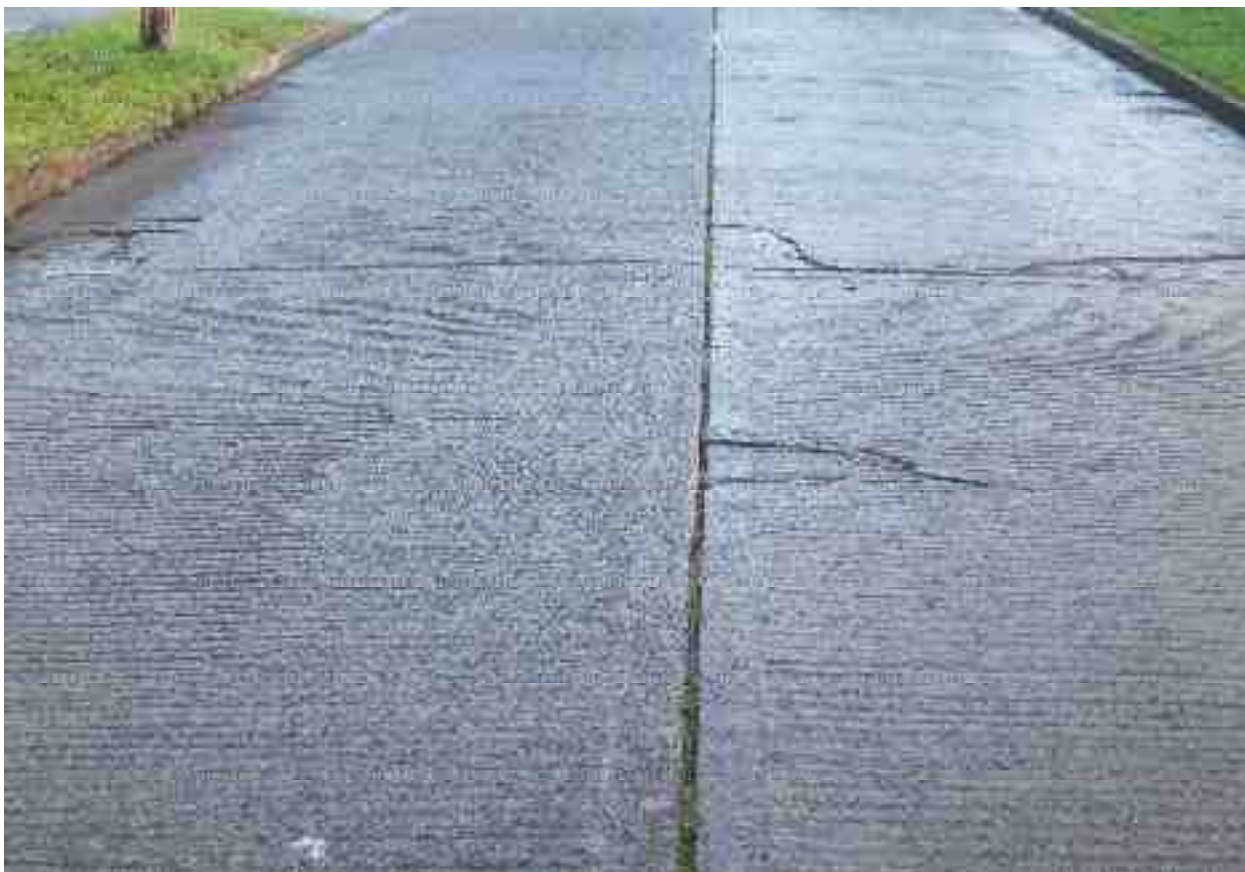
Rating 5: Multiple Corner breaks and some linear cracking present, cracks are narrow in width
