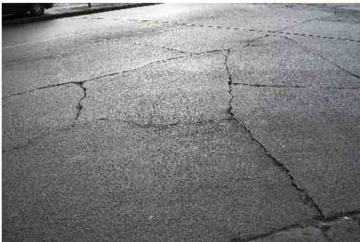
Rating 3: Shattered slab with cracking >12mm
