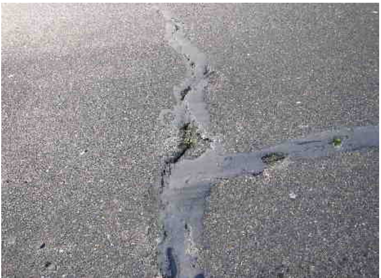
Very wide and Poorly sealed cracks showing severe deterioration
