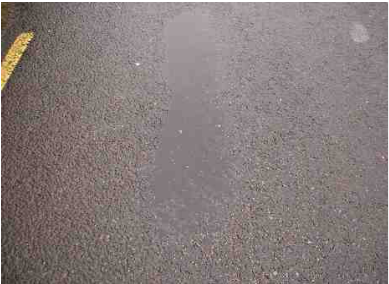
Fatting up of binder along the wheelpath on Clause 942 surface
