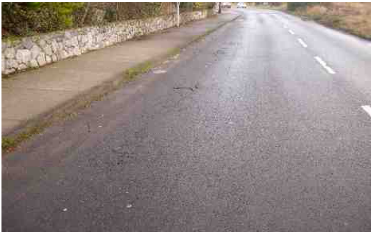
Rating 4: Alligator cracking in wheelpath, 5% to 25% of pavement surface
