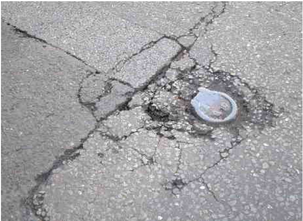
Failed pavement surface in vicinity of small ironworks
