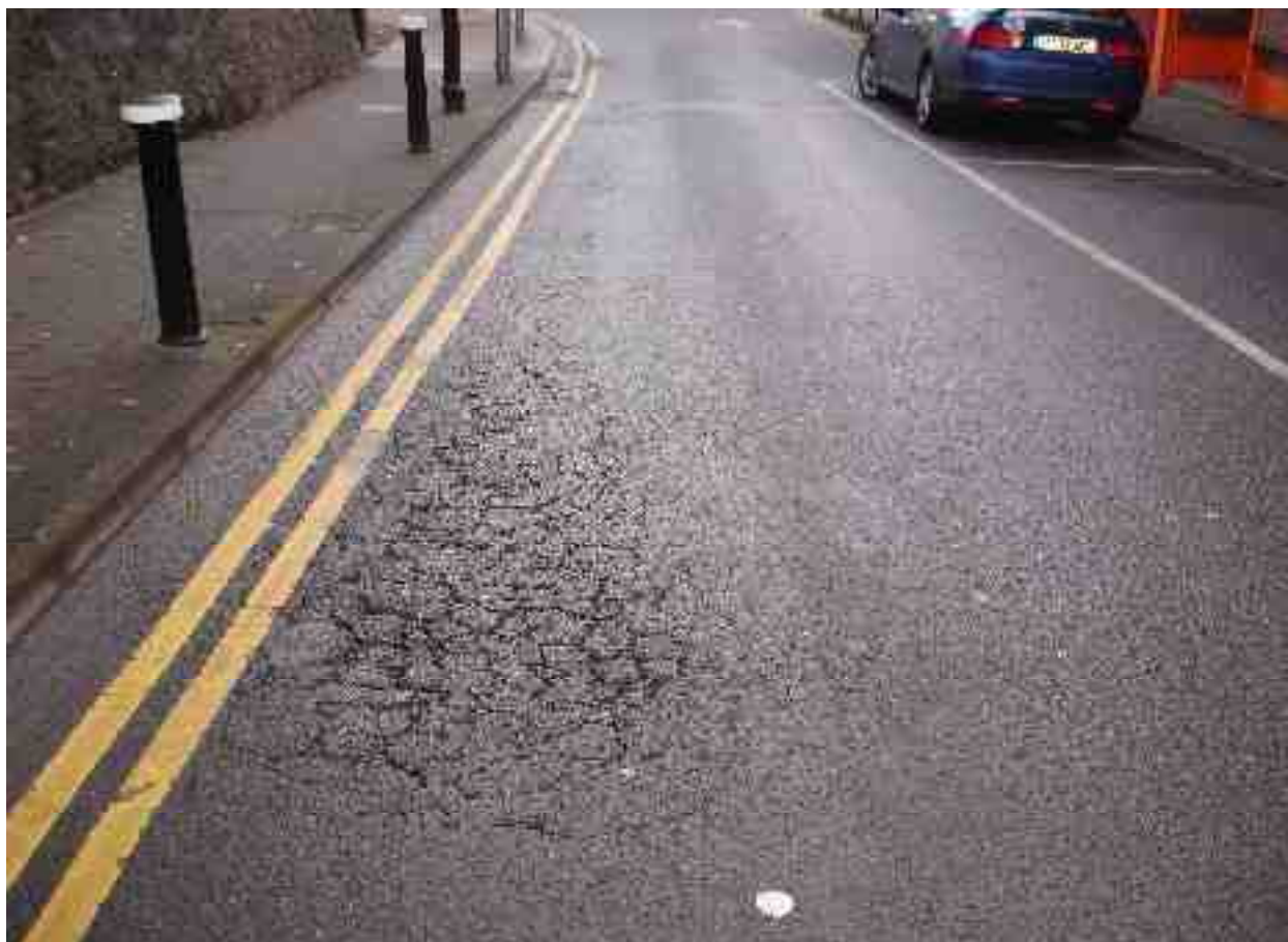
Severe alligator cracking with spalling and loose pieces
