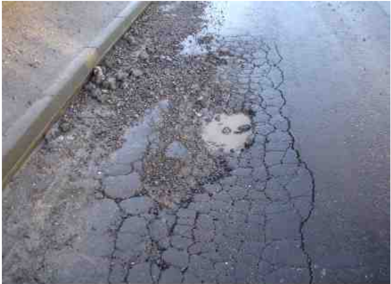
Large isolated pothole, extends through base. Note adjacent alligator cracks which commonly deteriorate into potholes
