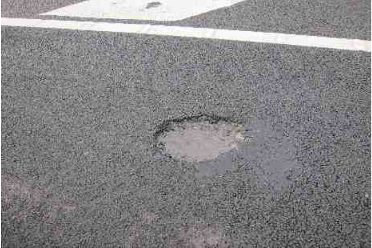
New pothole in PMSMA (Clause 942) surface
