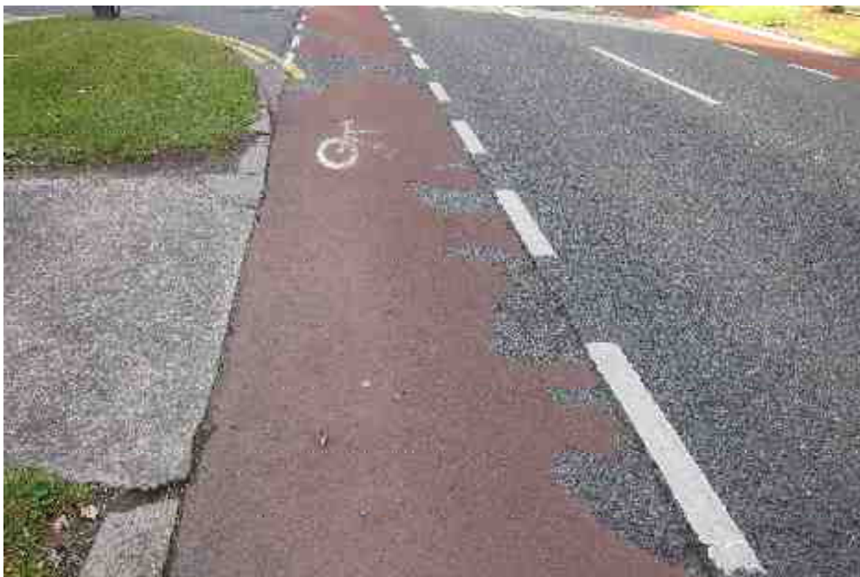
Rating 8: Ravelling in Cycle track on carriageway lane
