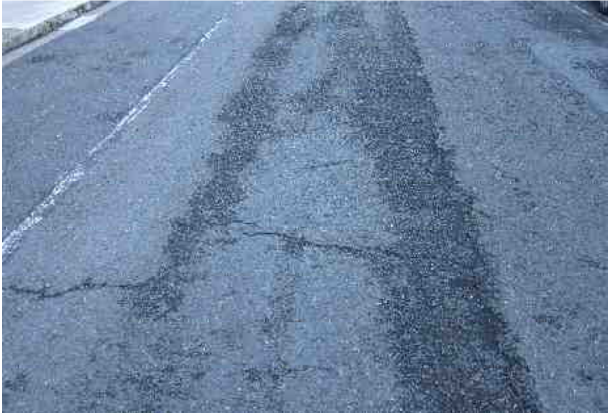
Moderate Ravelling in vicinity of linear cracks
