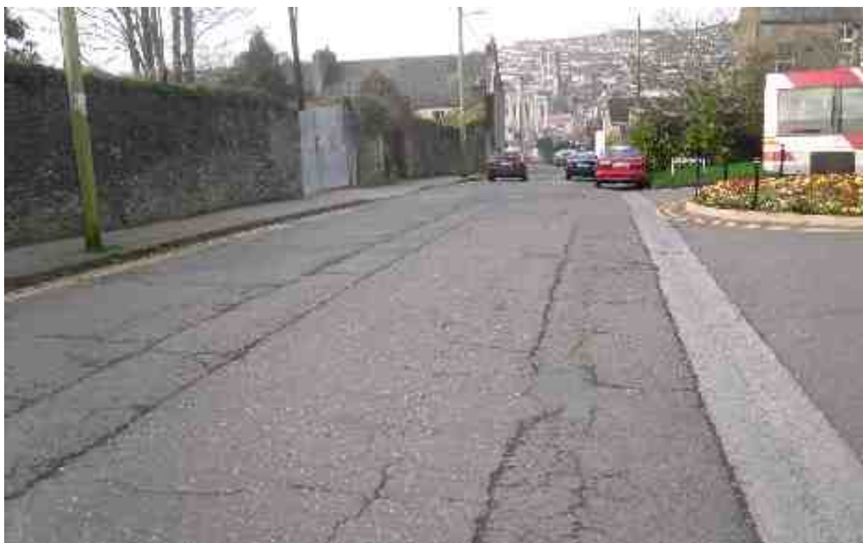
Rating 4: Structural distress (5 to 25%) and linear cracking on pavement surface
