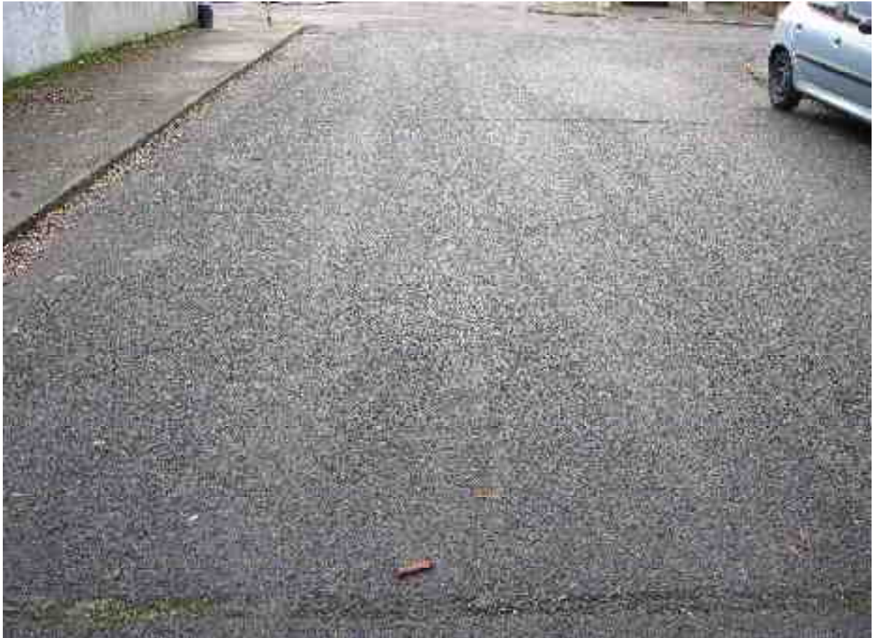
Meander reflection cracking
