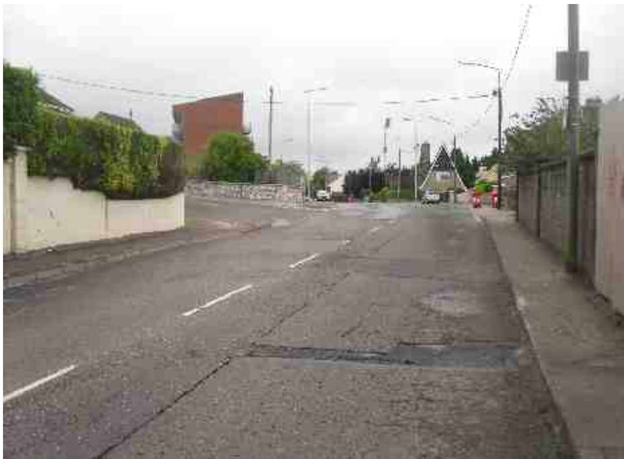
Rating 4: Structural distress (5 to 25%), with some patching in poor condition
