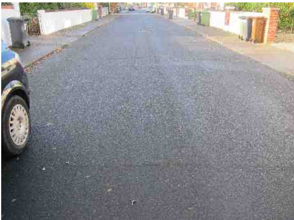
Rating 6: Reflection cracks, tight in nature over less than 20% of pavement surface
