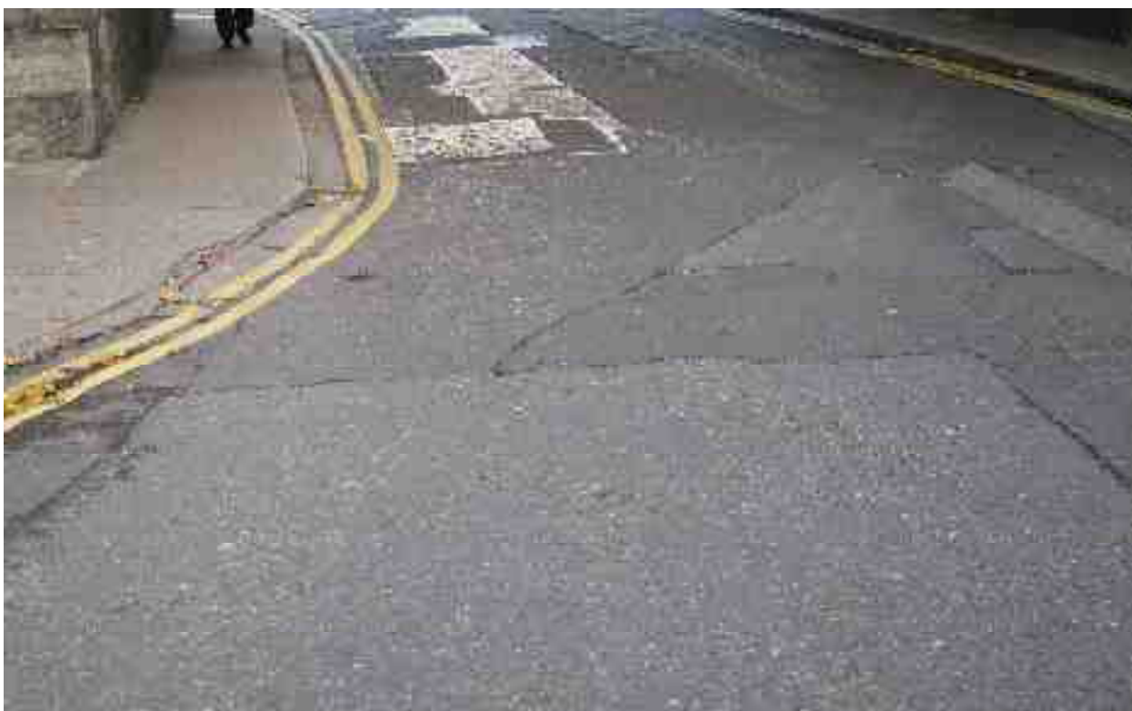
Rating 5: Extensive unsealed patching generally in fair condition
