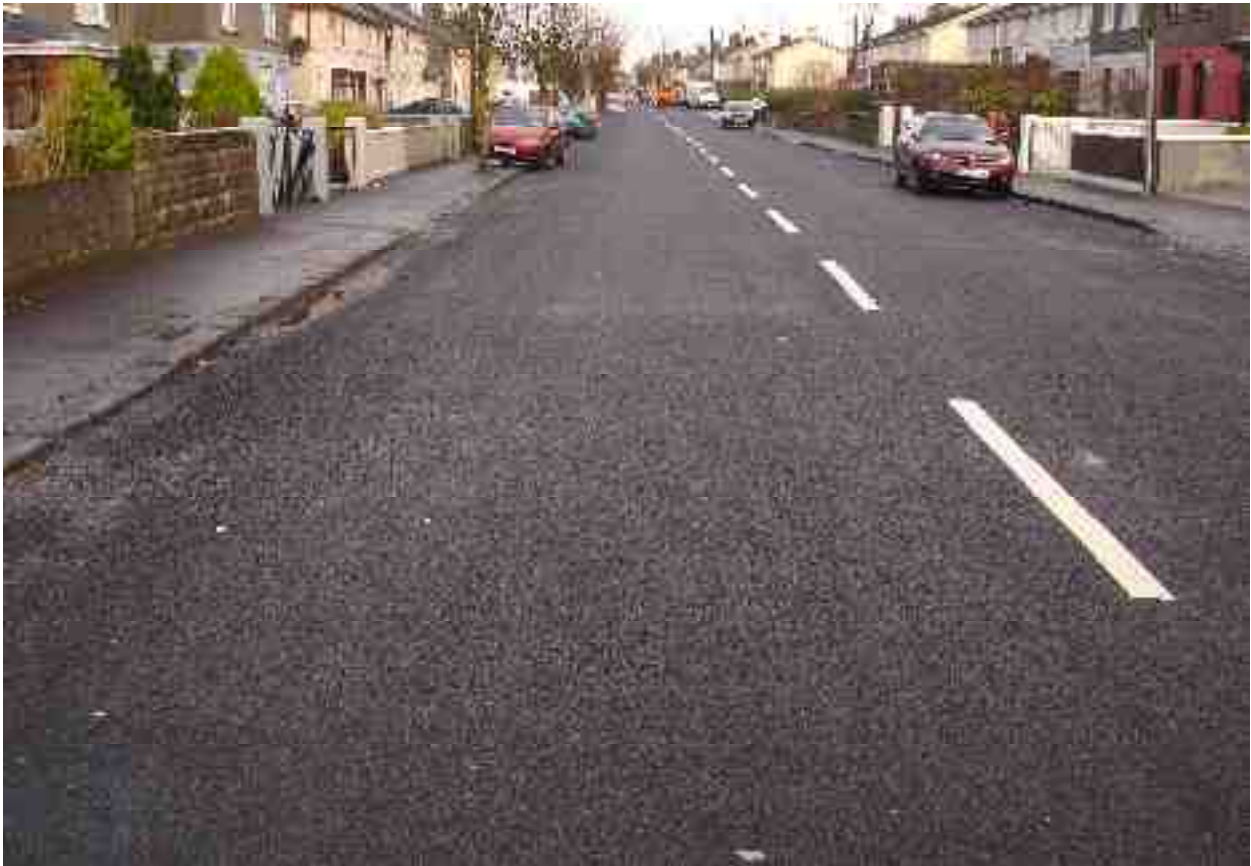
Rating 10: Road with no visible pavement defects, relatively new surface dressing
