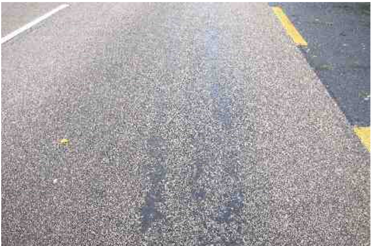
Ravelling along wheelpath on High Friction Surface
