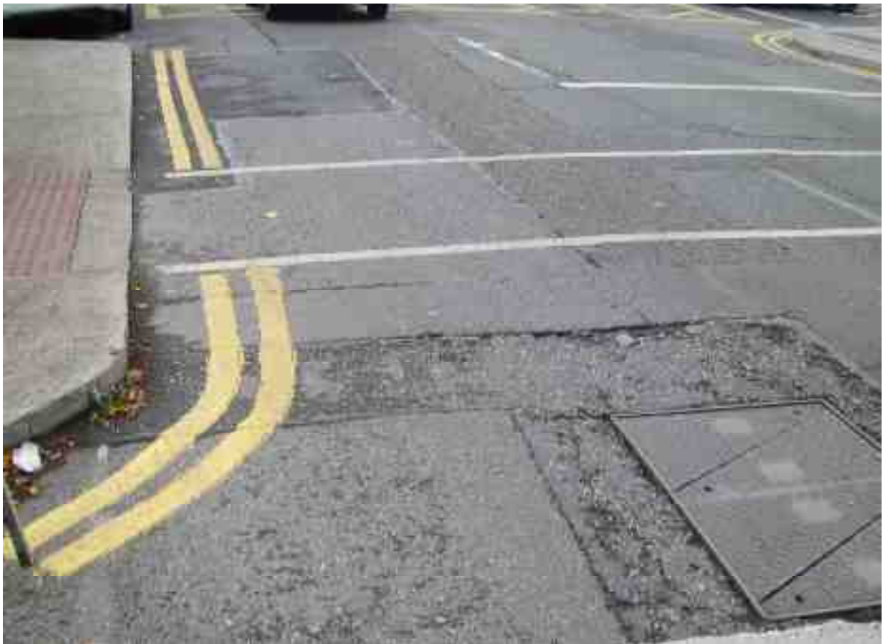
Utility cut patching repairs in fair condition
