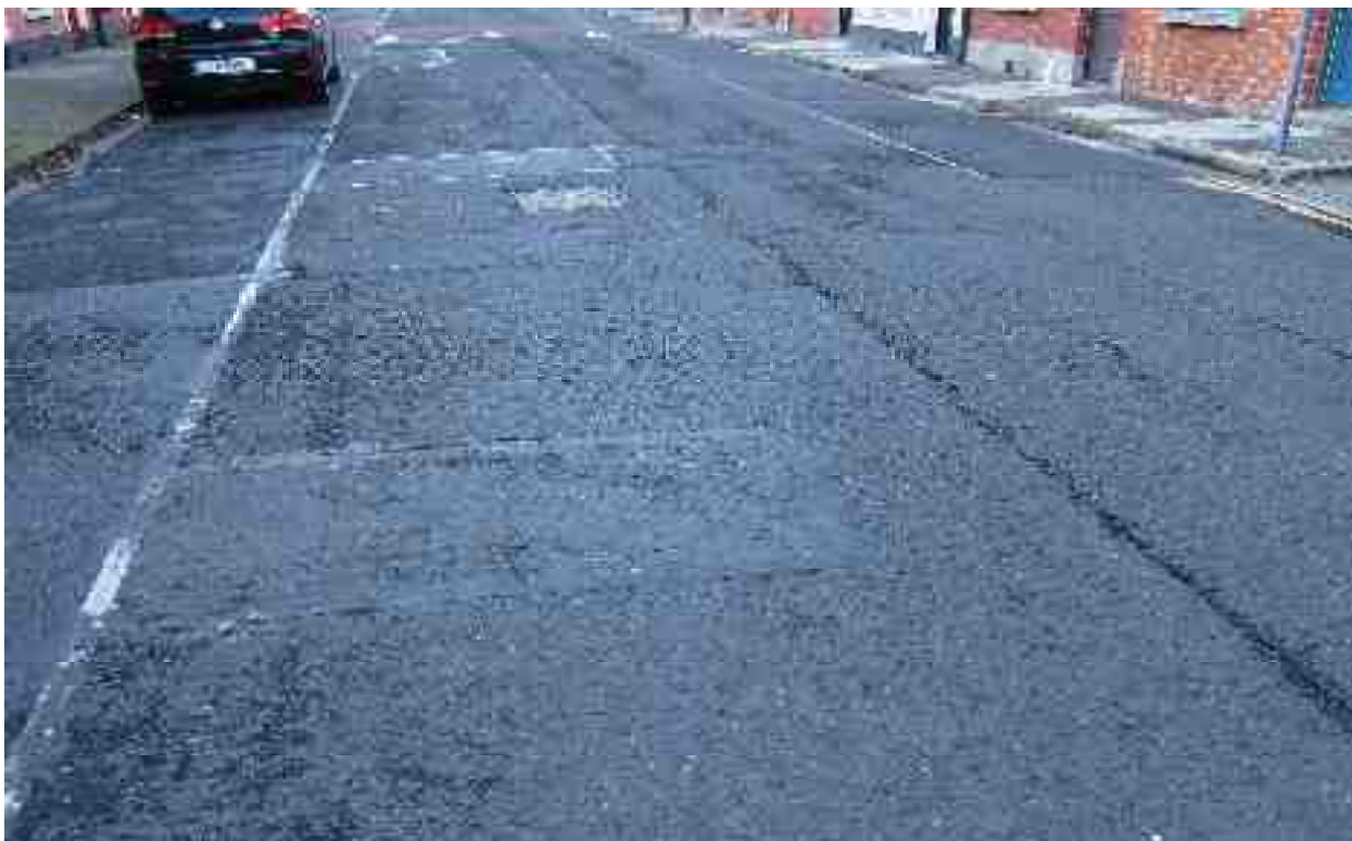
Rating 6: Pavement surface with linear cracking and patching generally in good condition
