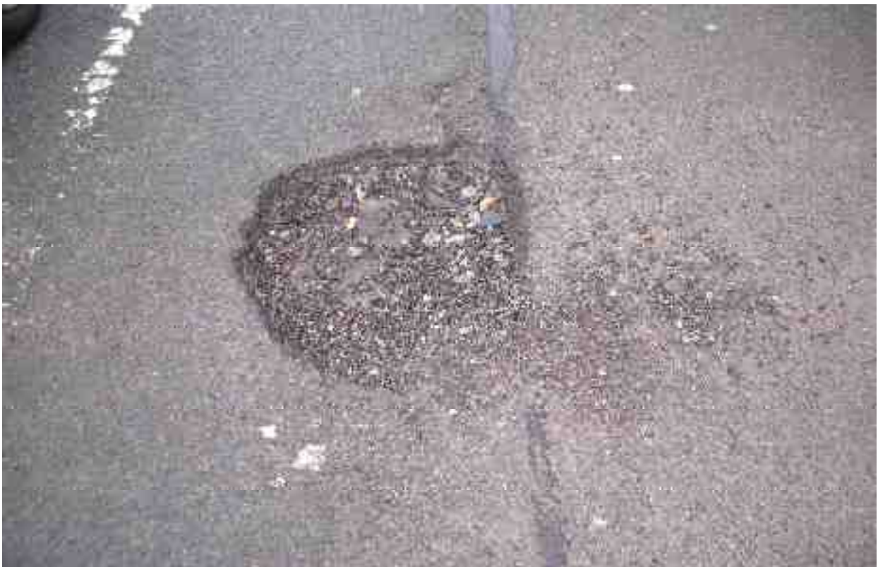
Medium sized pothole where top course has broken away
