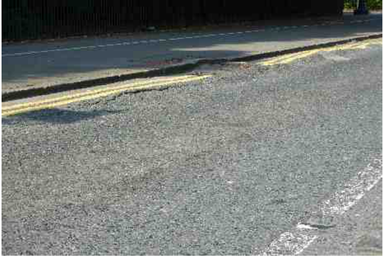
Severe Rutting over 50mm in depth, width of rut indicates subgrade problems
