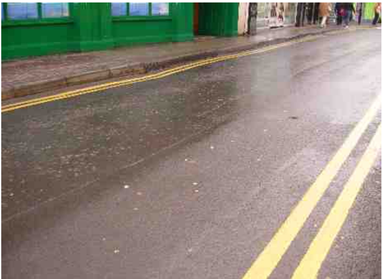
Pavement deformation (note road marking on left edge)
