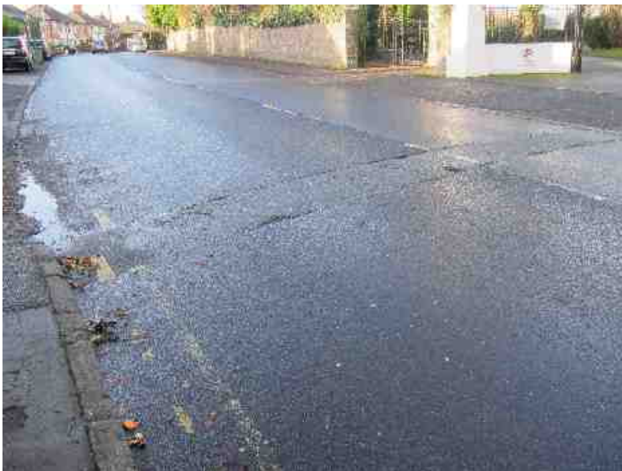
Rating 6: Utility cut patch with surface defects present on pavement
