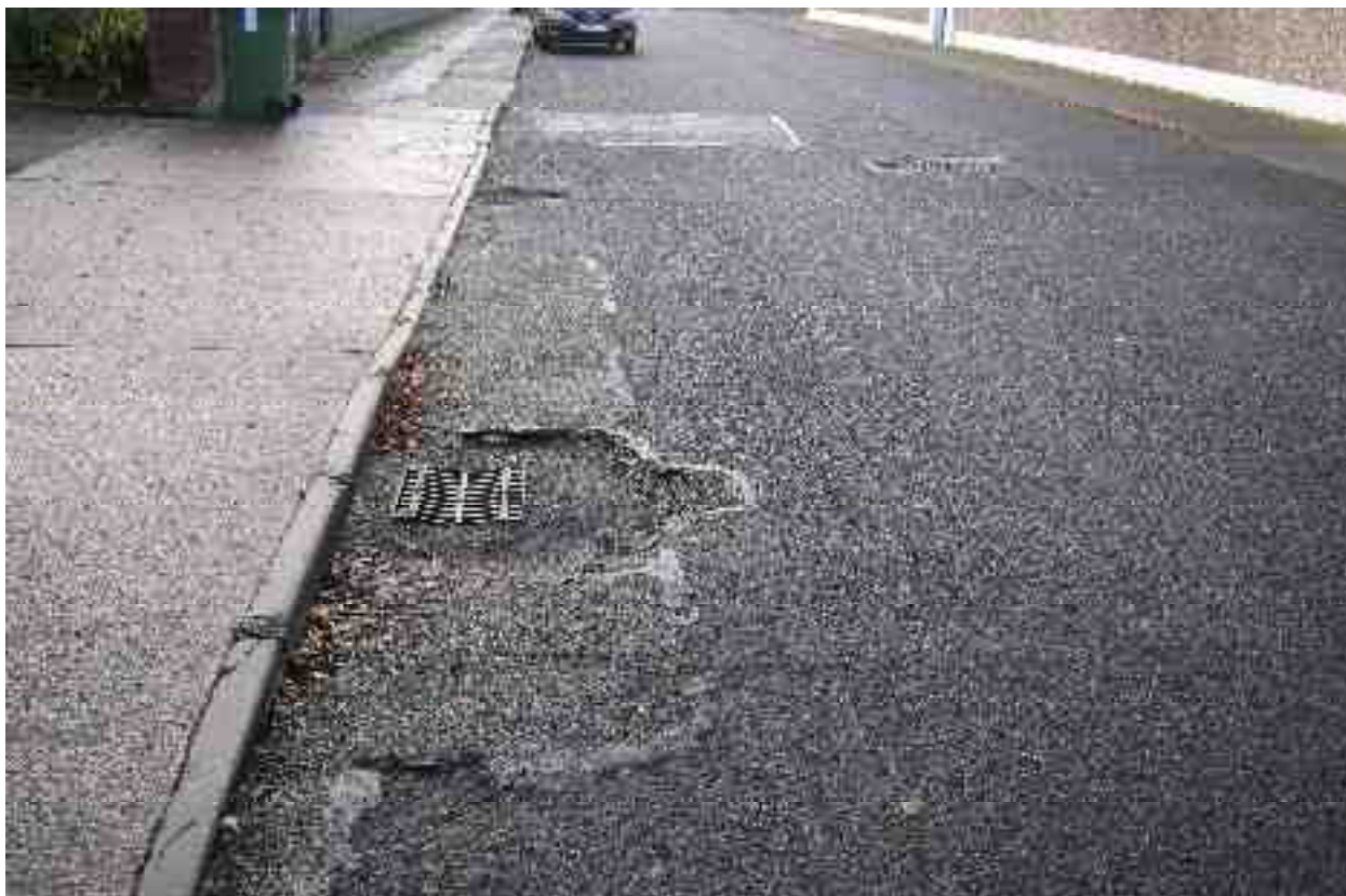
Rating 5: Patching generally in fair condition but failed in vicinity of ironworks
