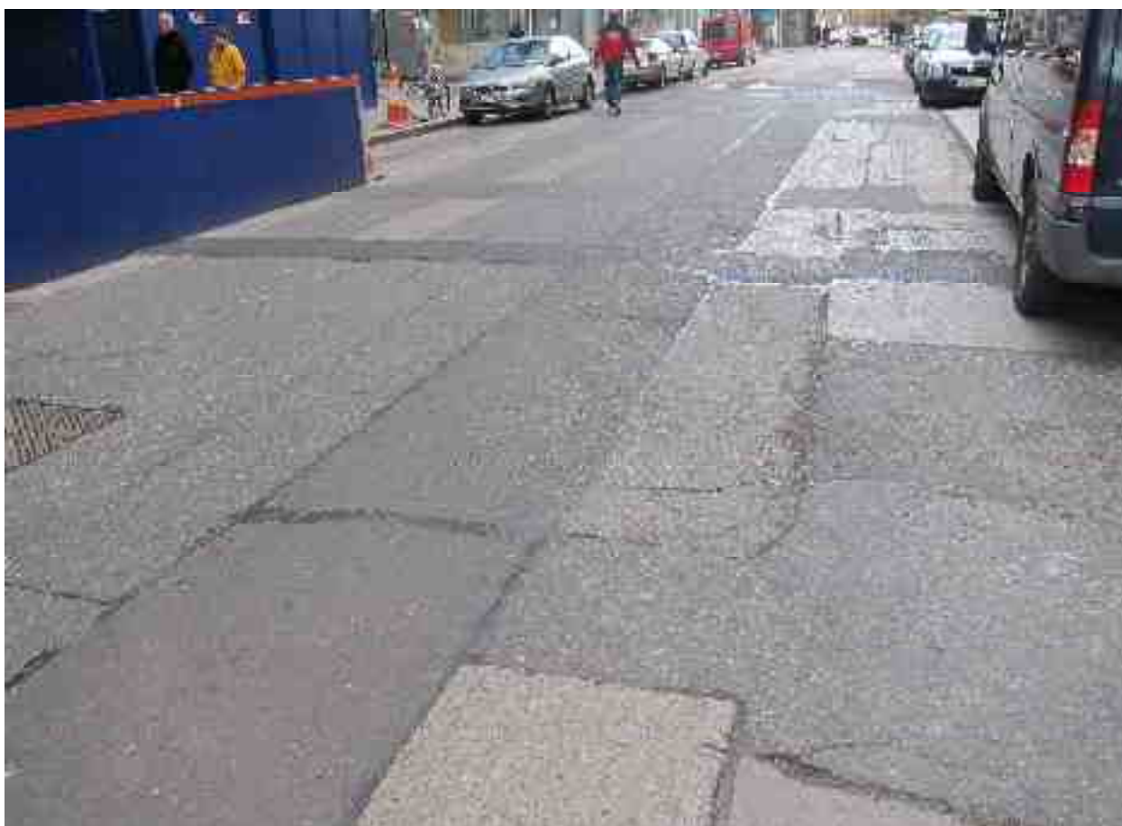
Rating 4: Extensive patching showing signs of distress and deterioration
