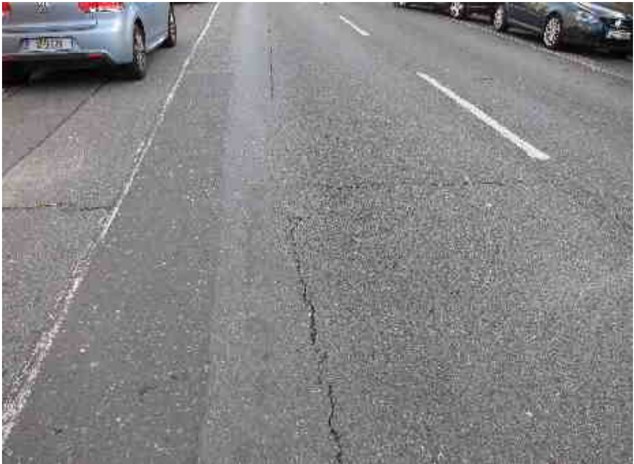
Reflection cracking, narrow width ( \leq 12\text{mm} )
