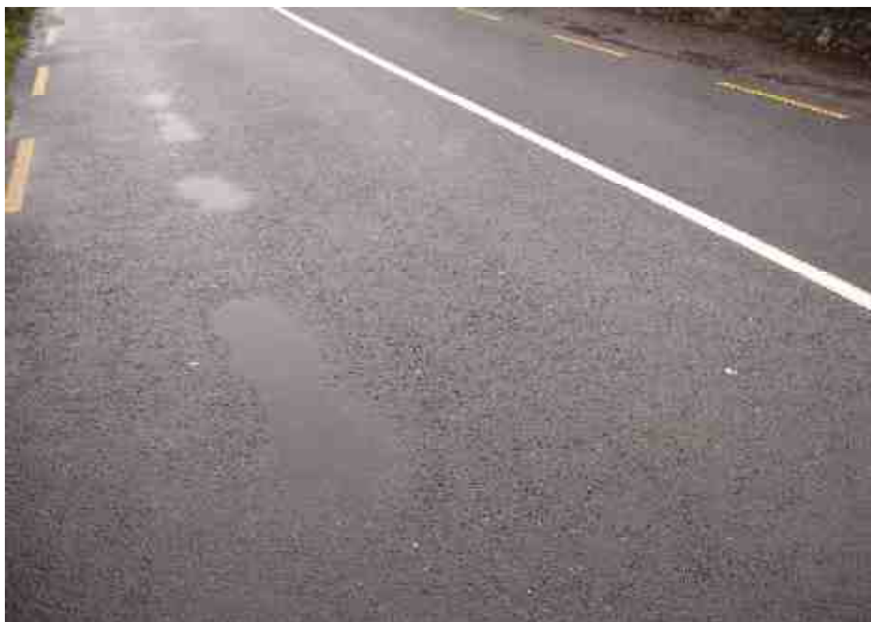
Rating 9: Fatting up of pavement surface less than 10%
