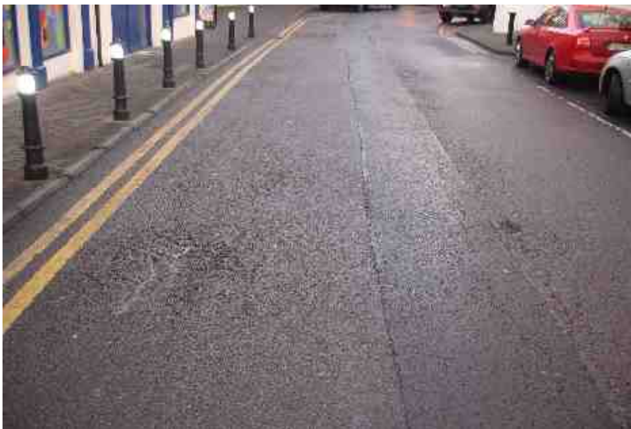
Rating 3: Severe alligator cracking and rutting evident over 50% of surface
