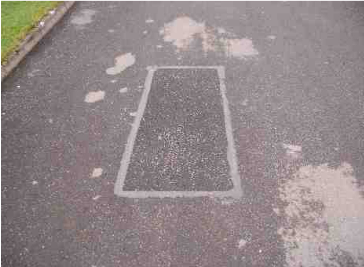
Well sealed small patch in very good condition
