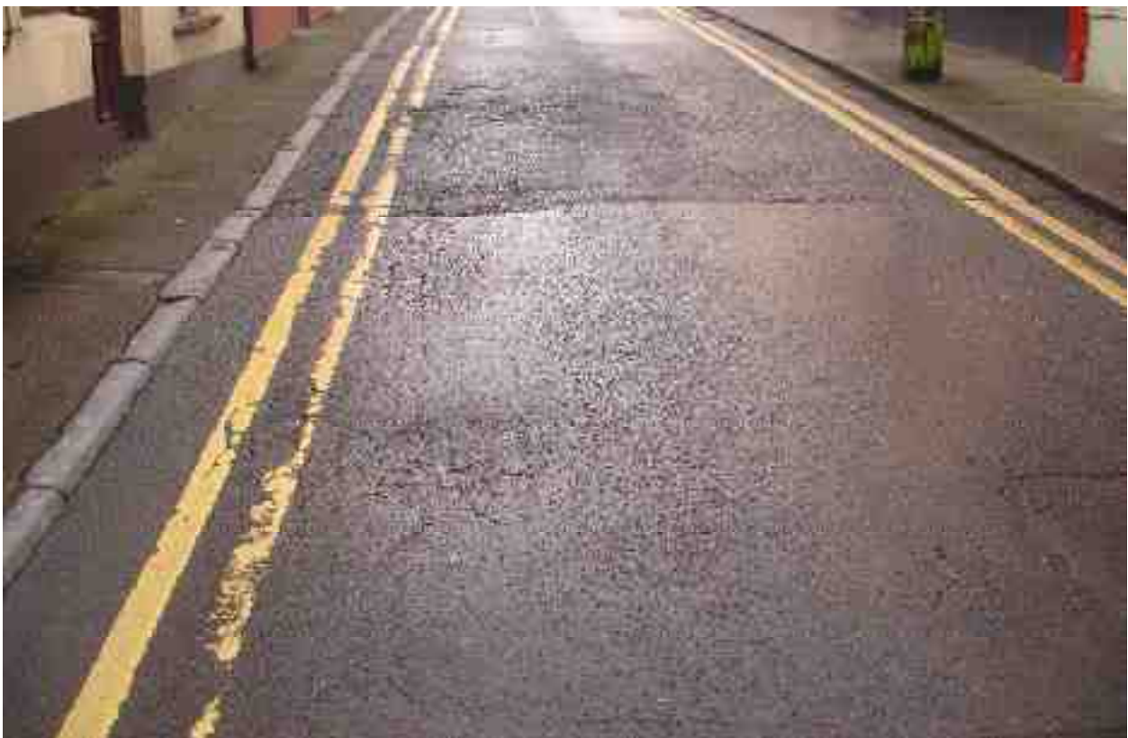
Rating 3: Extensive alligator cracking with surface deformation
