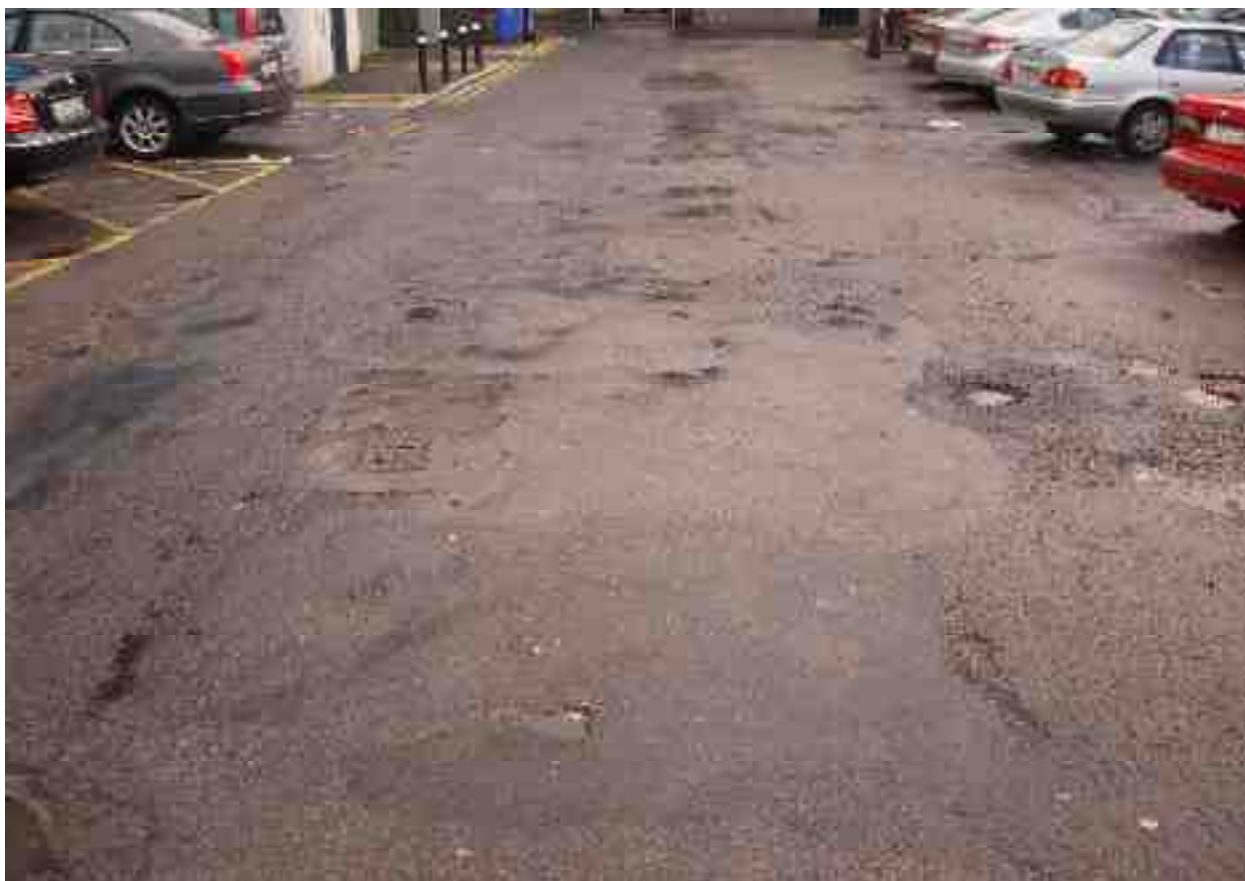
Rating 1: Severely deteriorated, extensive patching and structural problems, loss of surfacing in places
