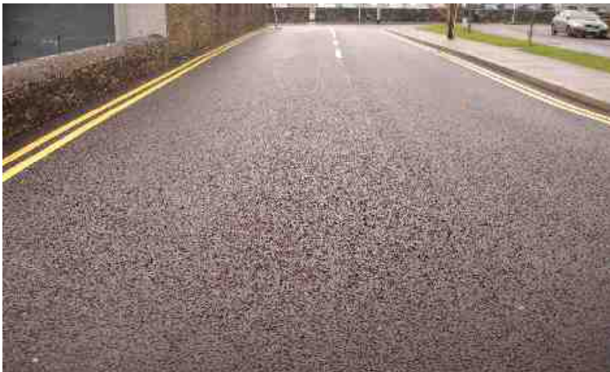
Rating 10: Road with no visible pavement defects, new Clause 942 surface
