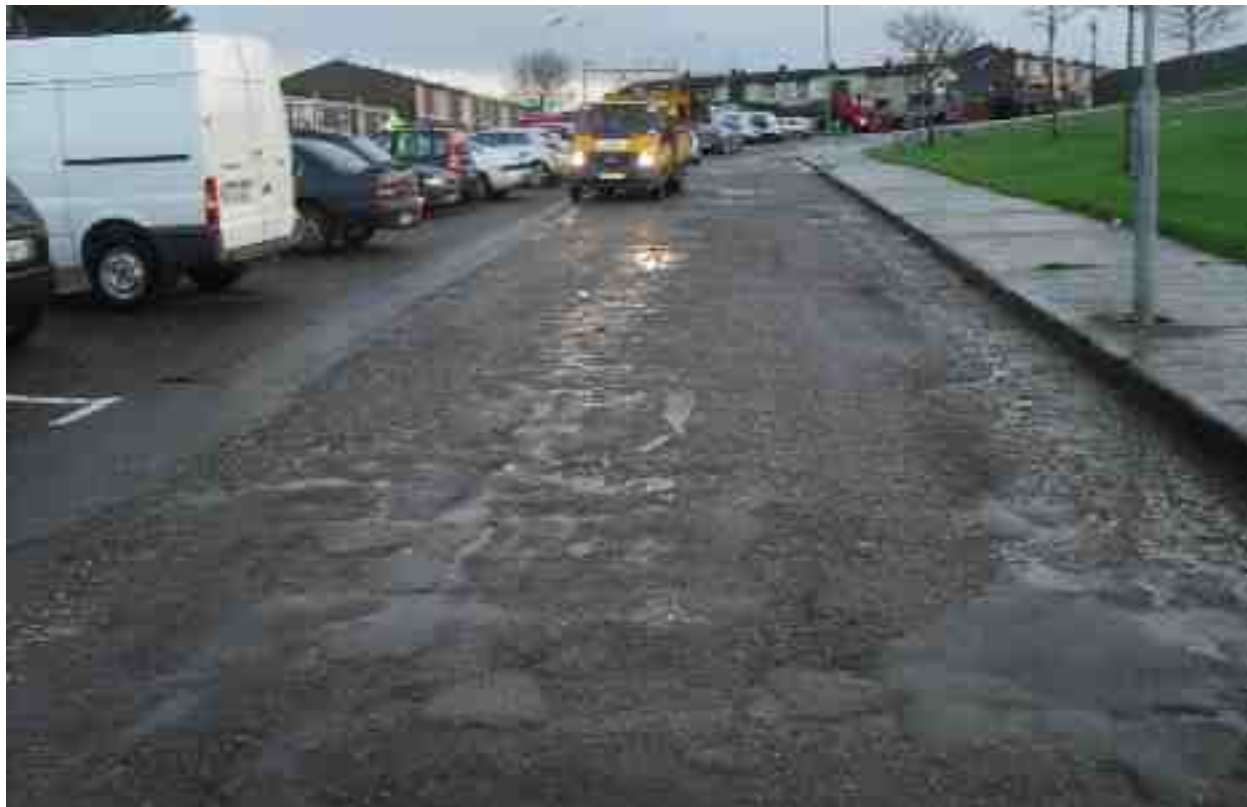
Rating 1: Extensive failed patching with severe deterioration, pavement failure
