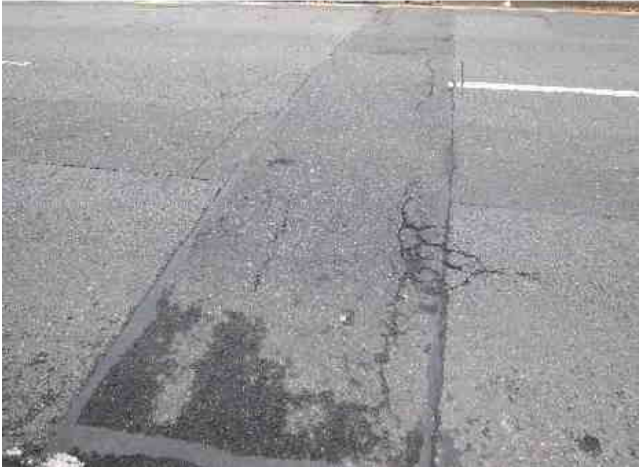
Utility Patch showing deterioration with linear and alligator cracking present
