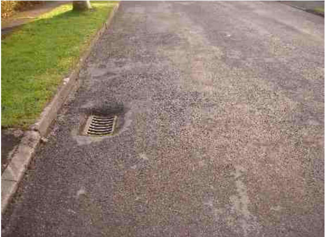
Inlet gully not raised to new road surface causing severe and sudden dip in left wheelpath
