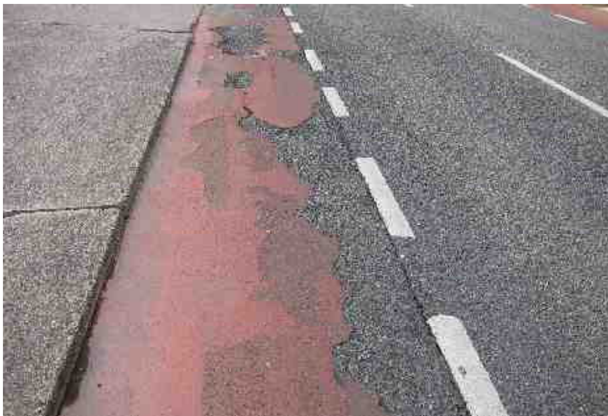
Ravelling along cycle track on carriageway lane
