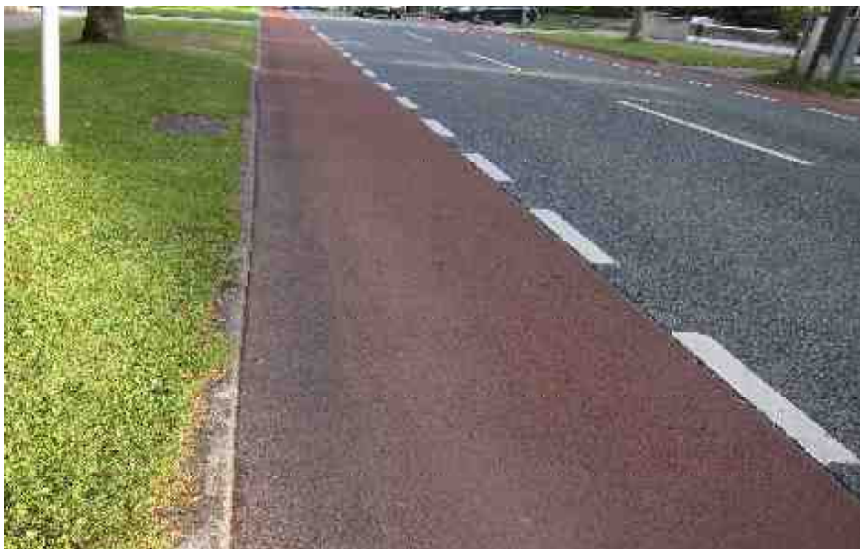
Rating 9: Pavement surface on carriageway and cycle lanes in very good condition
