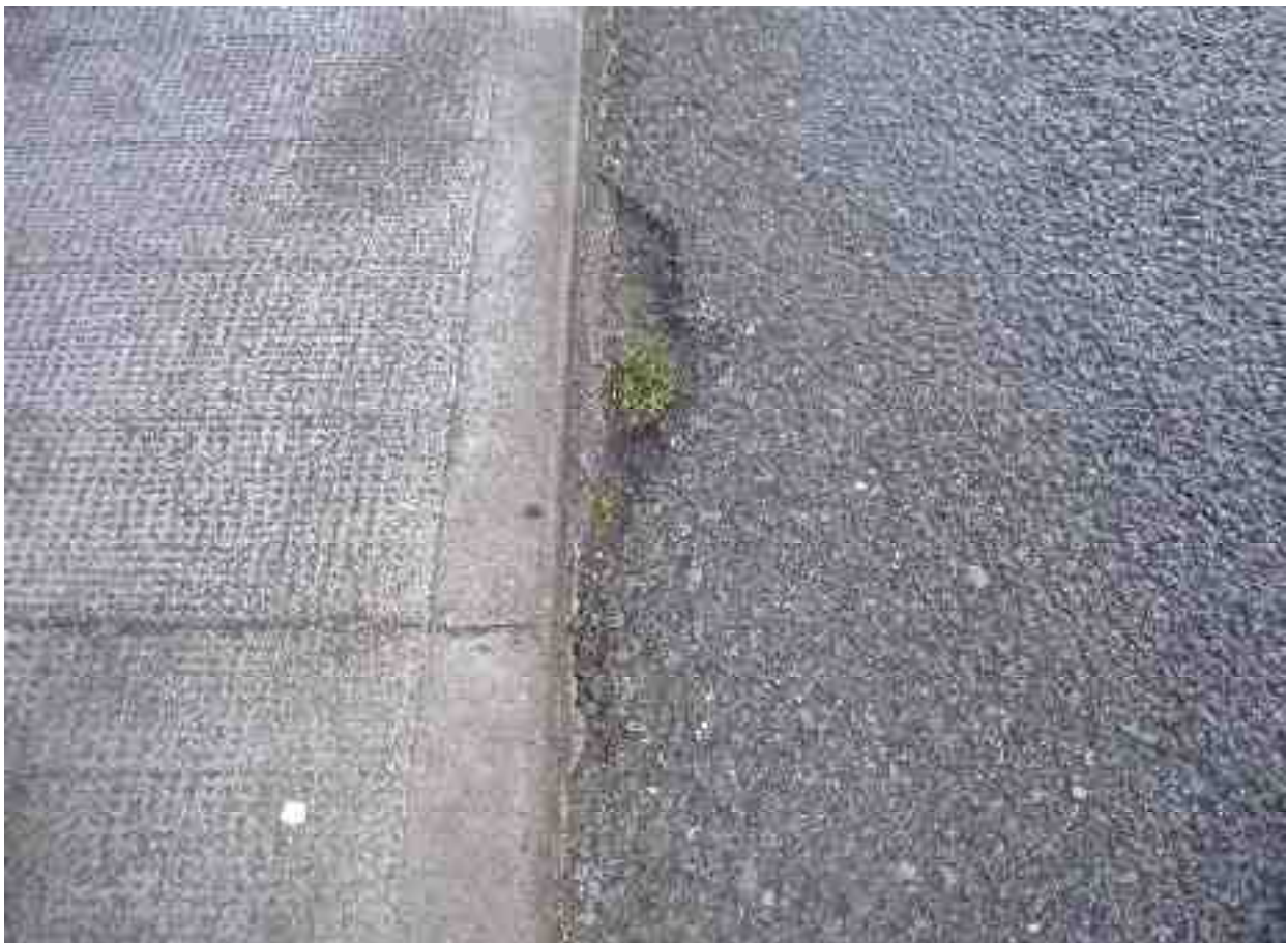
Edge breakup with loss of pavement material
