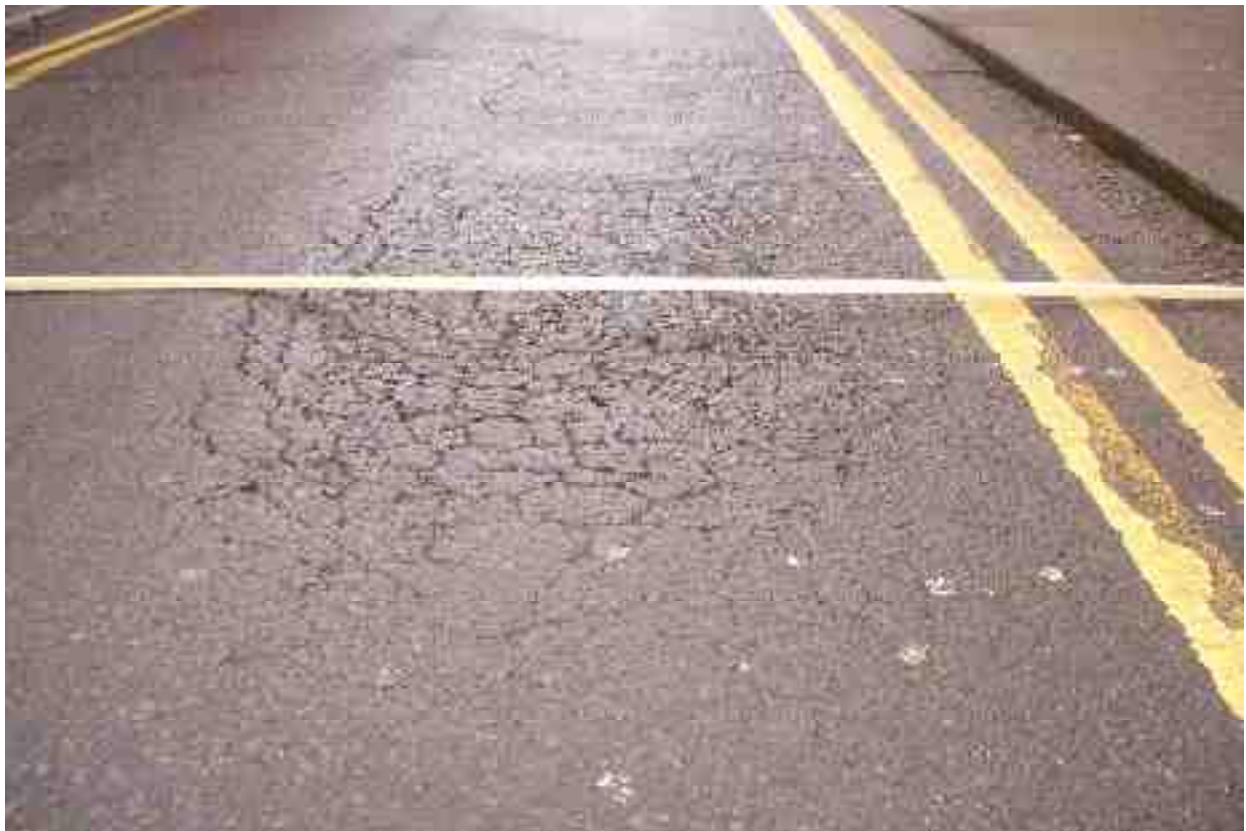
Severe Rutting with severe alligator cracking present
