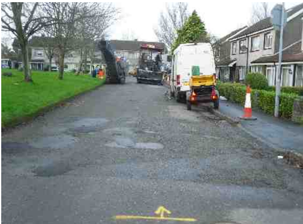
Rating 2: Severely deteriorated, extensive patching and structural problems , loss of surfacing in places
