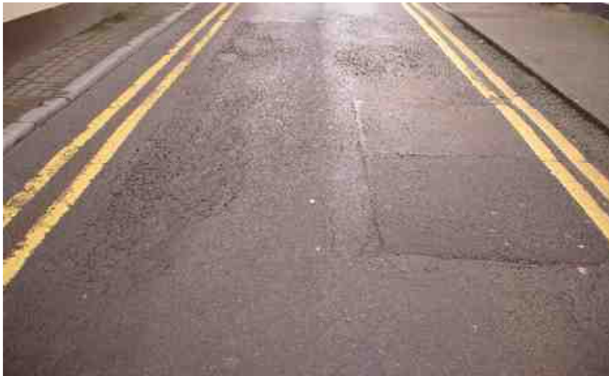
Rating 2: Severe alligator cracking and rutting (> 50mm) evident (> 50% of surface)
