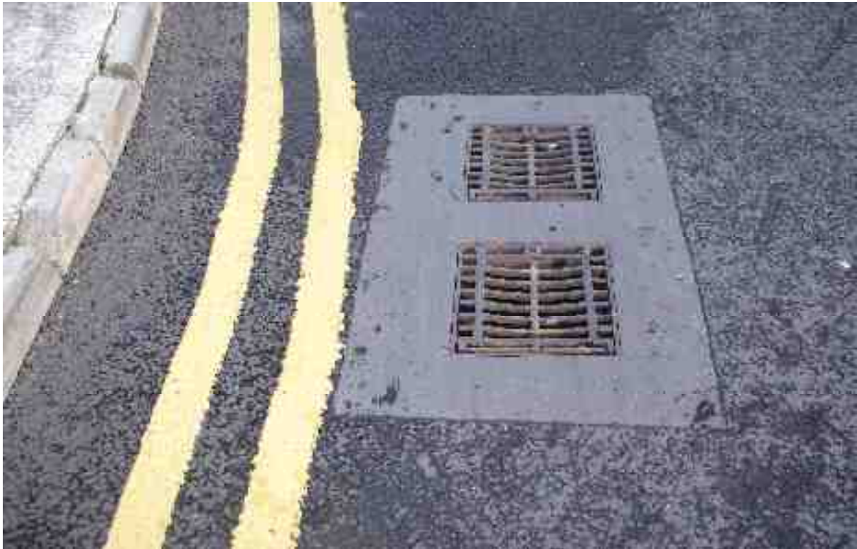
Dual pavement inlet gullies with new well sealed utility cut patch in excellent condition
