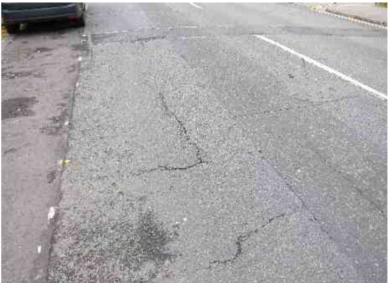
Longitudinal and Transverse cracking, relatively tight cracks
