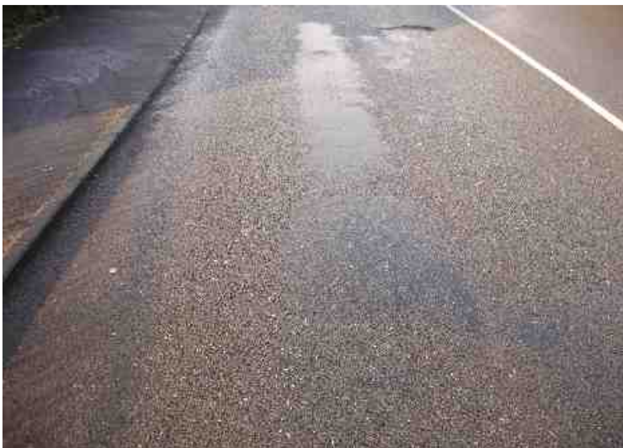
Rating 8: Bleeding on pavement surface (10% to 30%)
