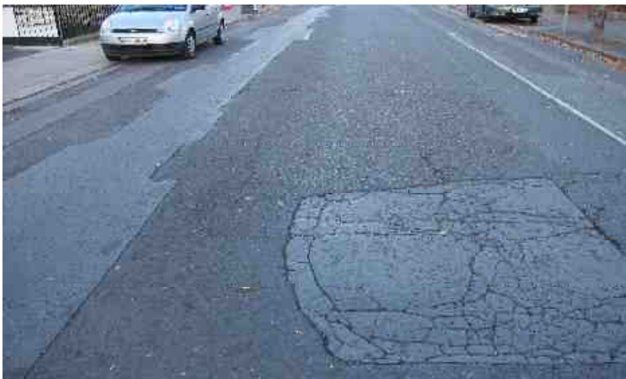
Rating 5: Utility patching in fair condition and localised structural distress in isolated patch
