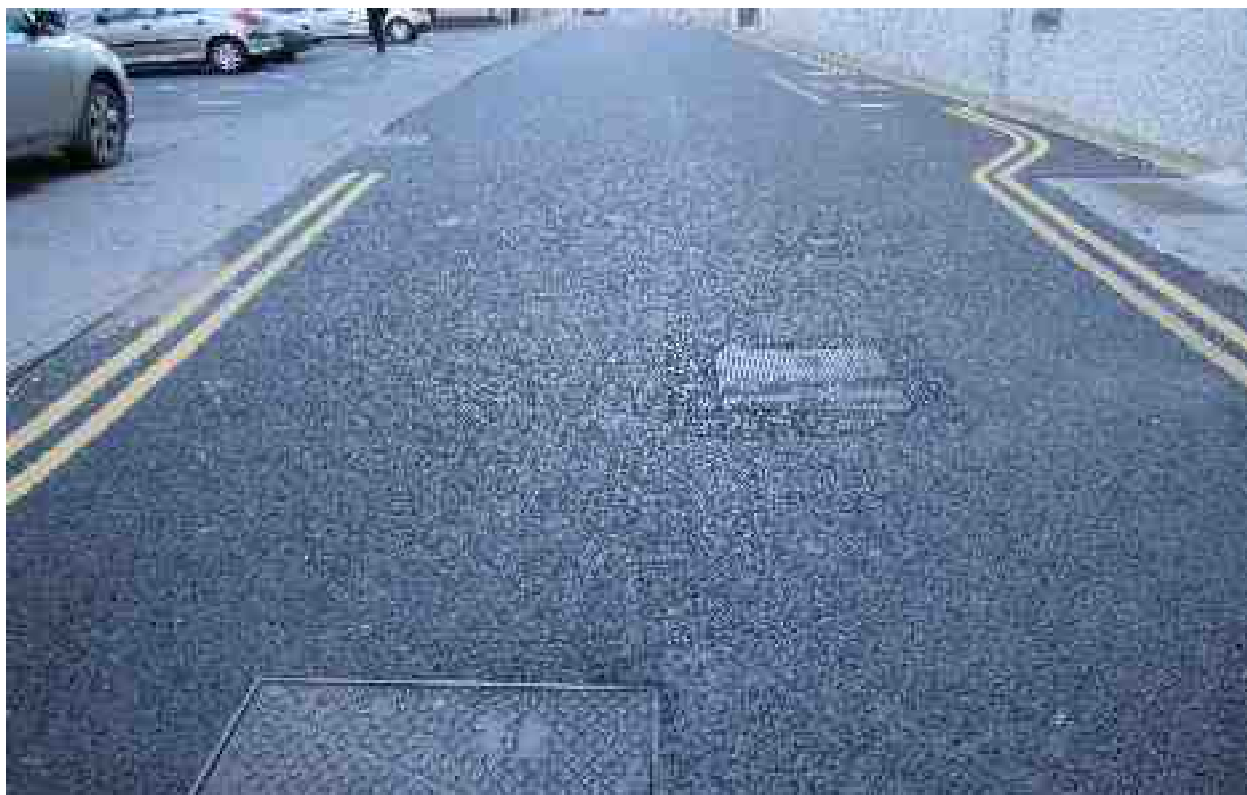
Rating 9: New surface with Manhole/ironworks patching in very good condition
