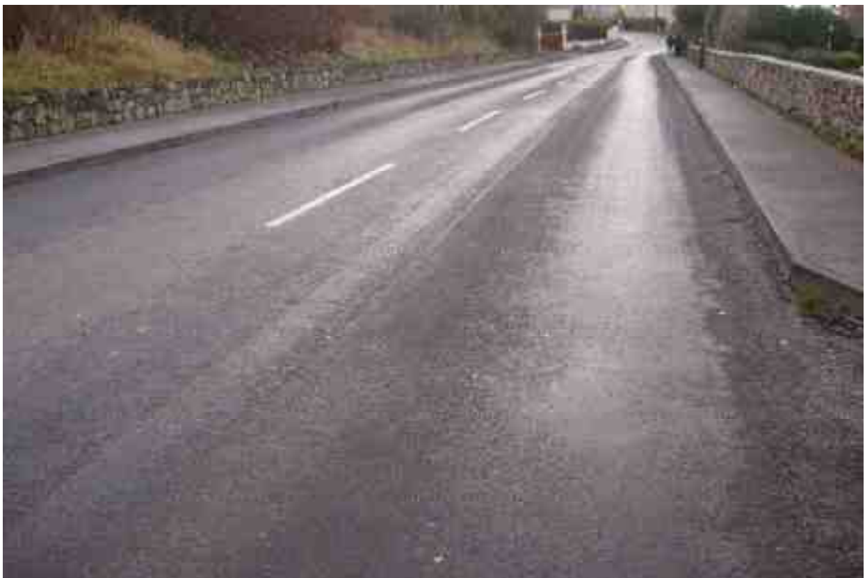
Bleeding: Darker, Shiny areas extending along the wheelpaths
