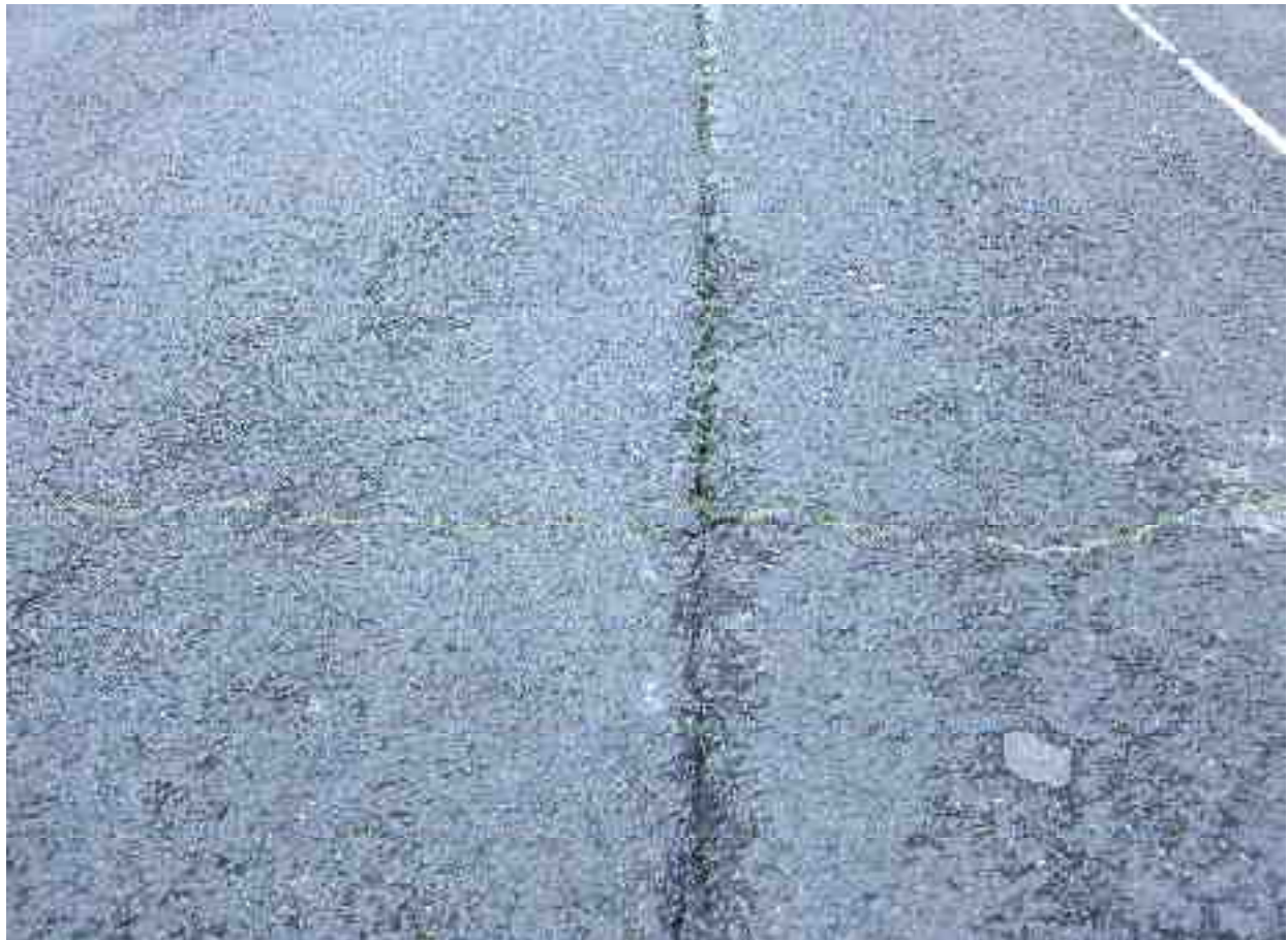
Reflection cracking, open ( > 12\text{mm} ) and unsealed
