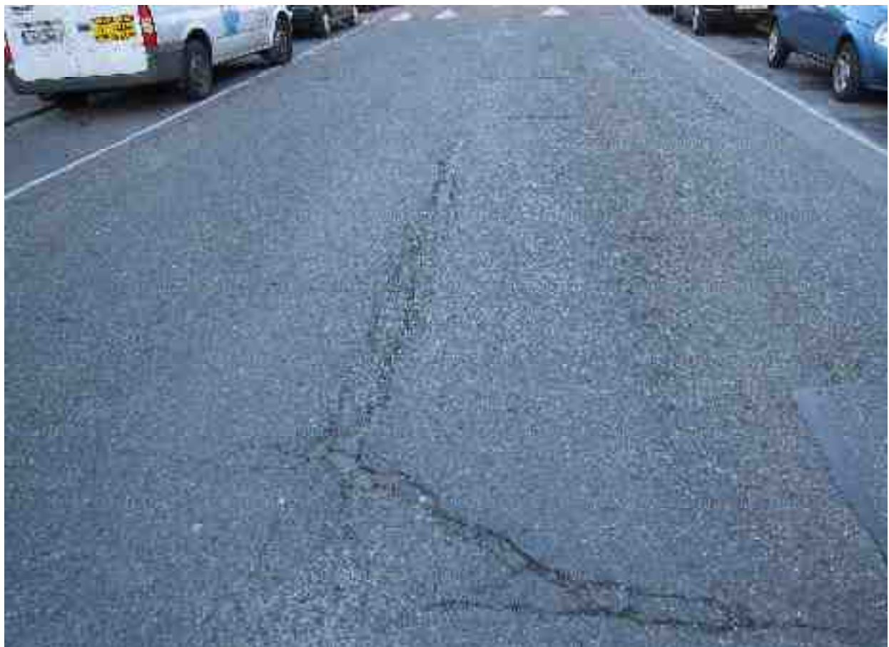
Wide open reflection cracking ( >12\text{mm} ) with spalling of edges
