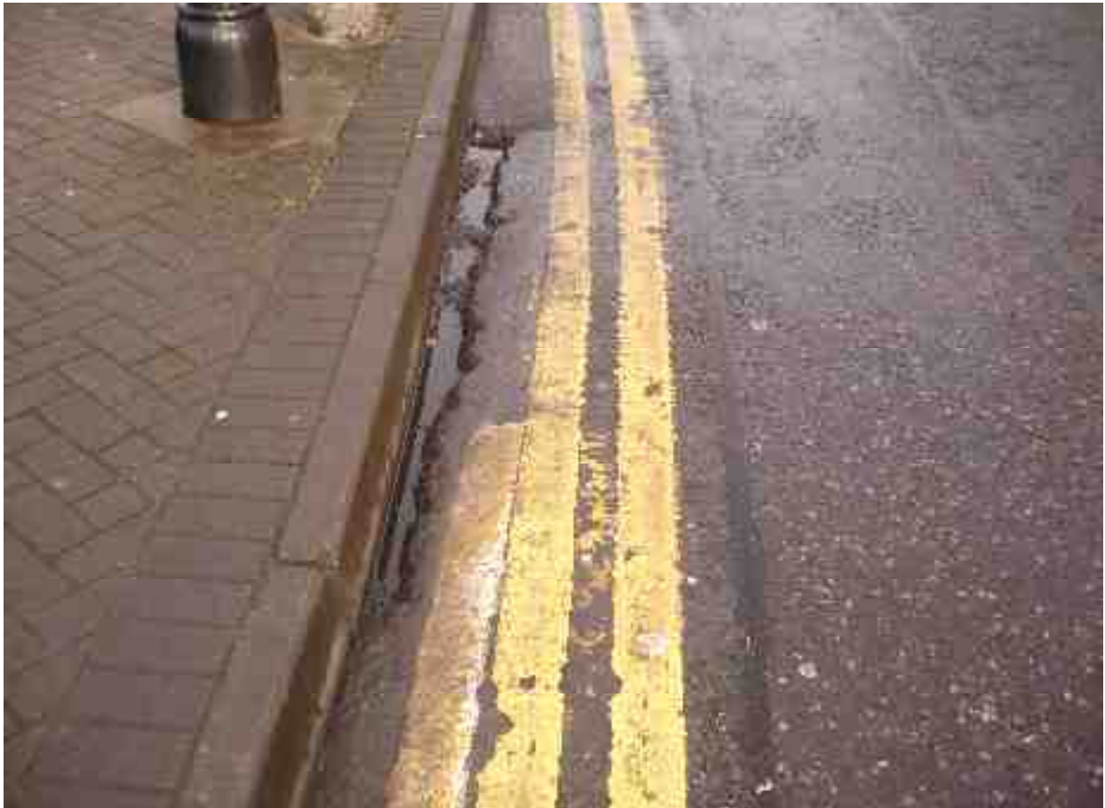
Edge breakup at road/footpath edge with material loss
