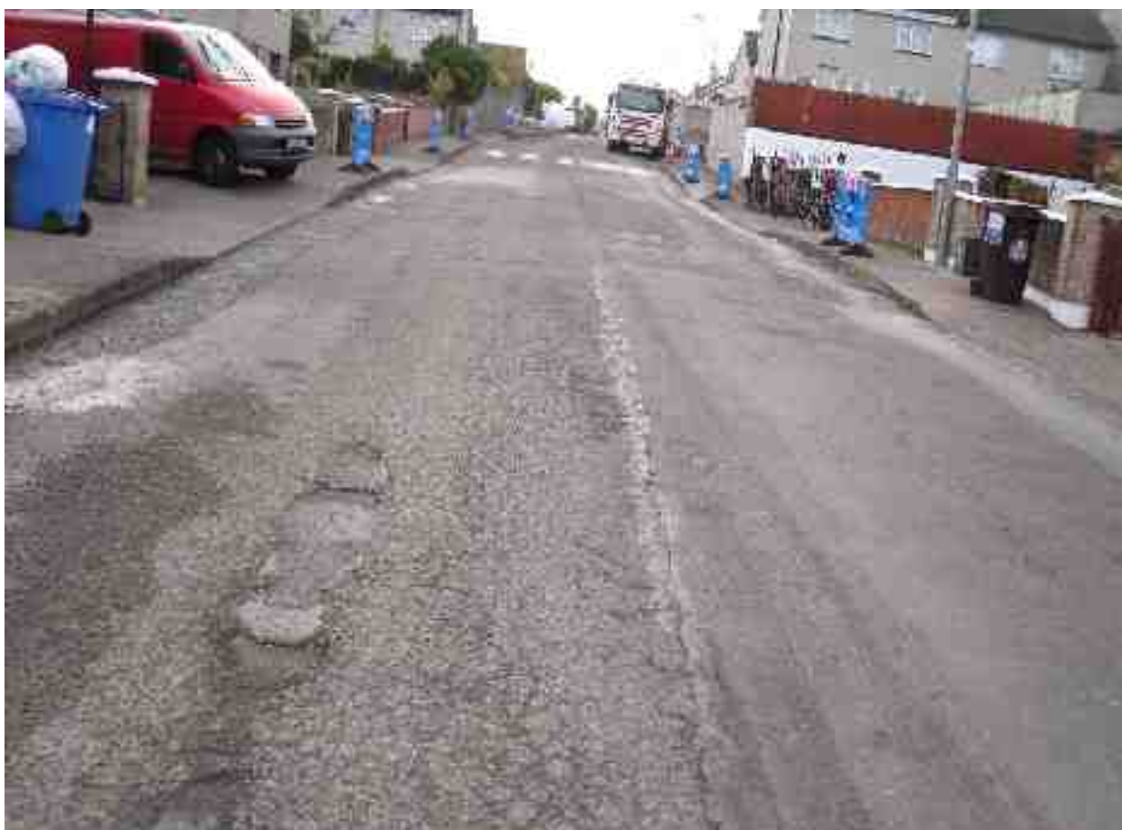
Rating 2: Extensive alligator cracking, very poor patching and potholes present, in very poor overall condition
