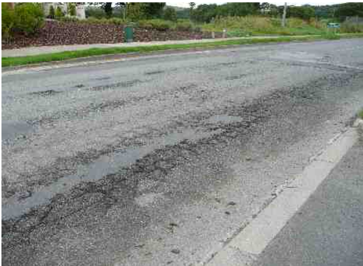
Rating 3: Extensive Alligator cracking and poor patching
