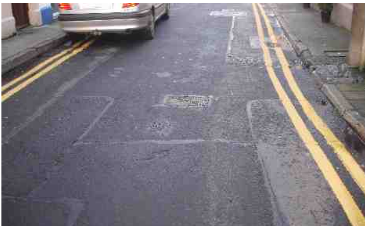
Rating 6: Extensive utility patching, generally in good condition
