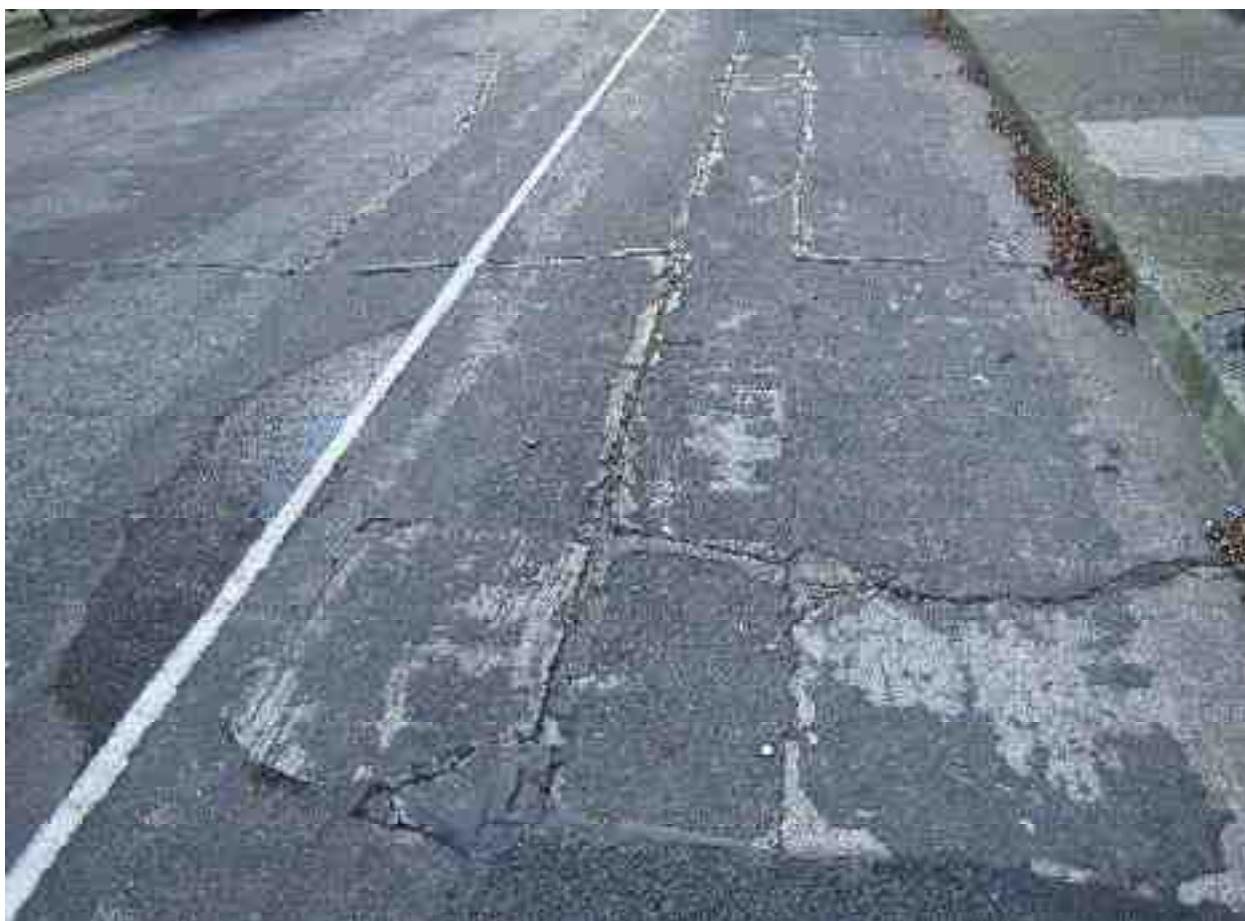
Rating 4: Wide open cracks and poorly sealed joints and cracks, bituminous surface failed on concrete pavement
