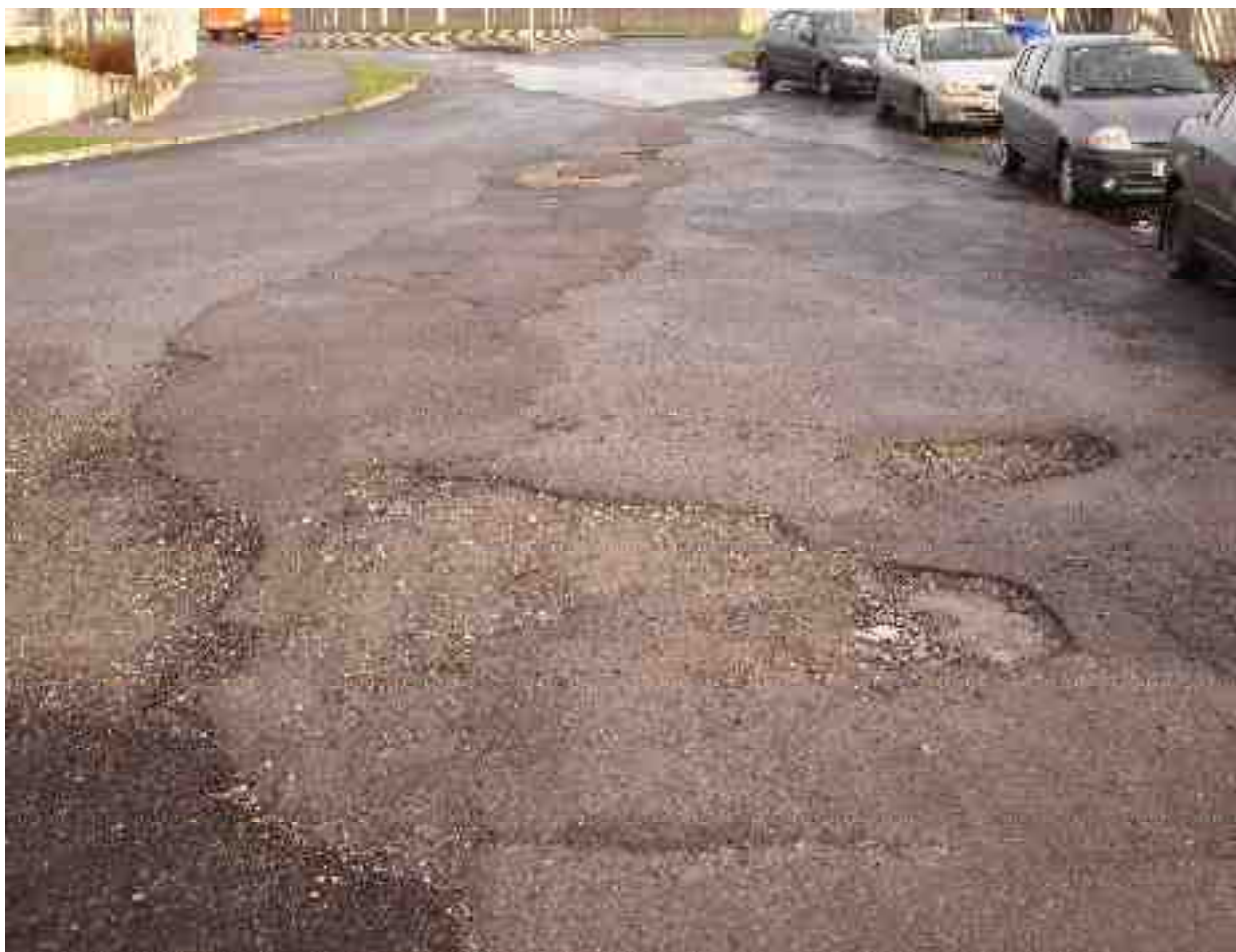
Rating 1: Failed pavement with extensive failed patching and large surface openings
