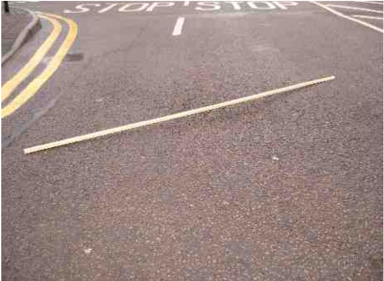
Depression in pavement surface producing flat irregular shaped basin
