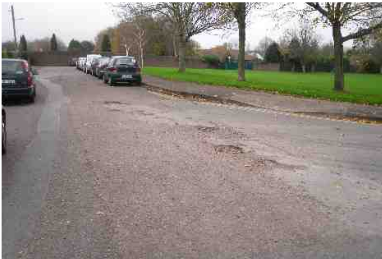
Rating 3: Pavement in poor condition, with potholes and poor patching present
