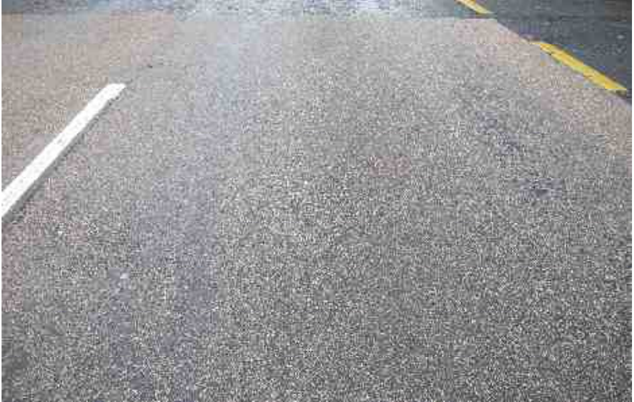
Rating 8: Ravelling in wheelpaths of High Friction Surface (10% to 30%)
