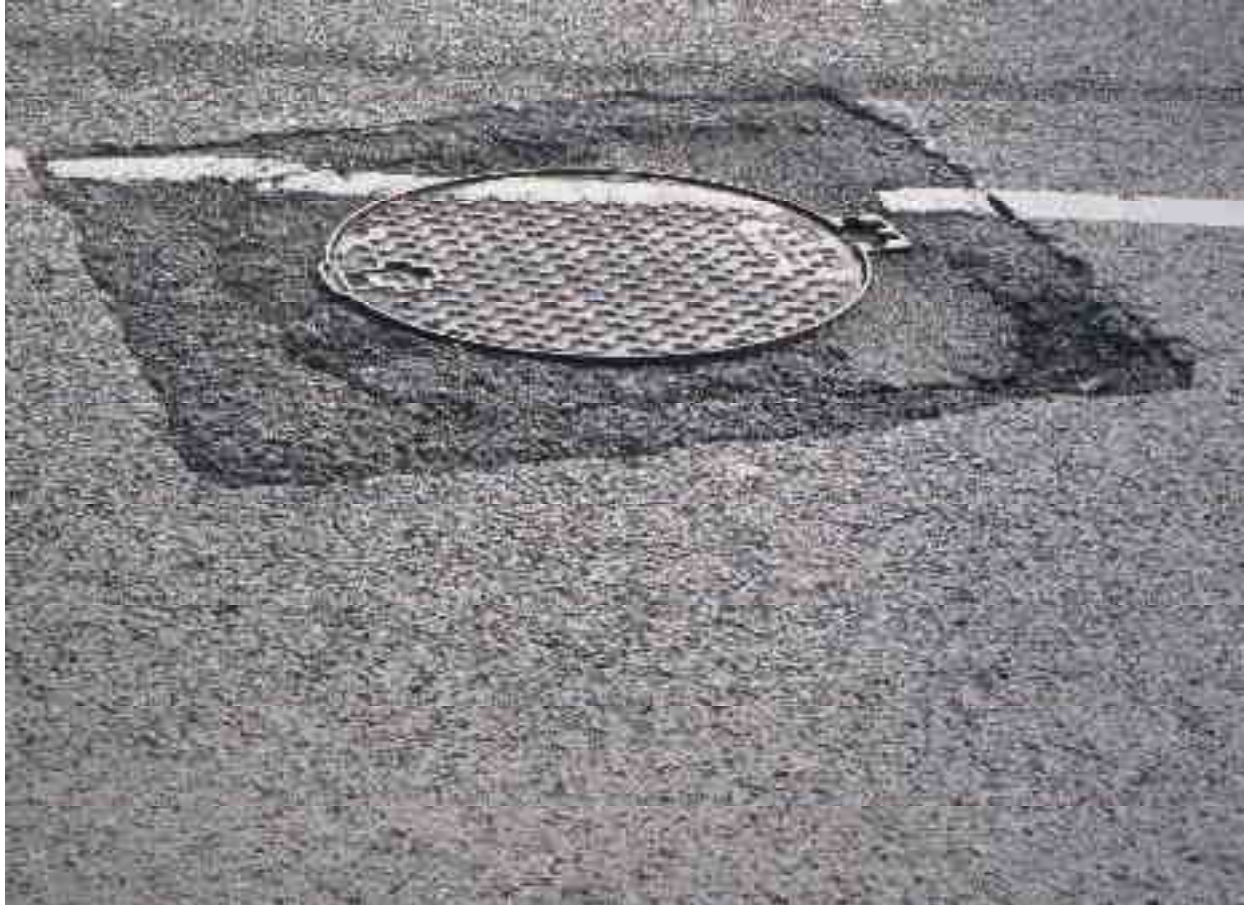
Manhole with utility repair in poor condition
