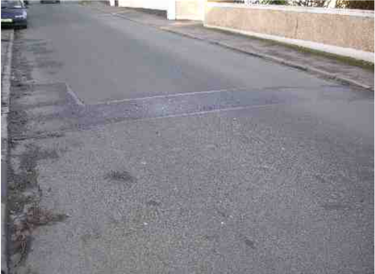
Utility cut repair in very good condition with well sealed joints
