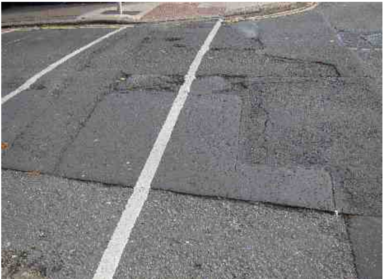
Very poor patching with extensive distress present
