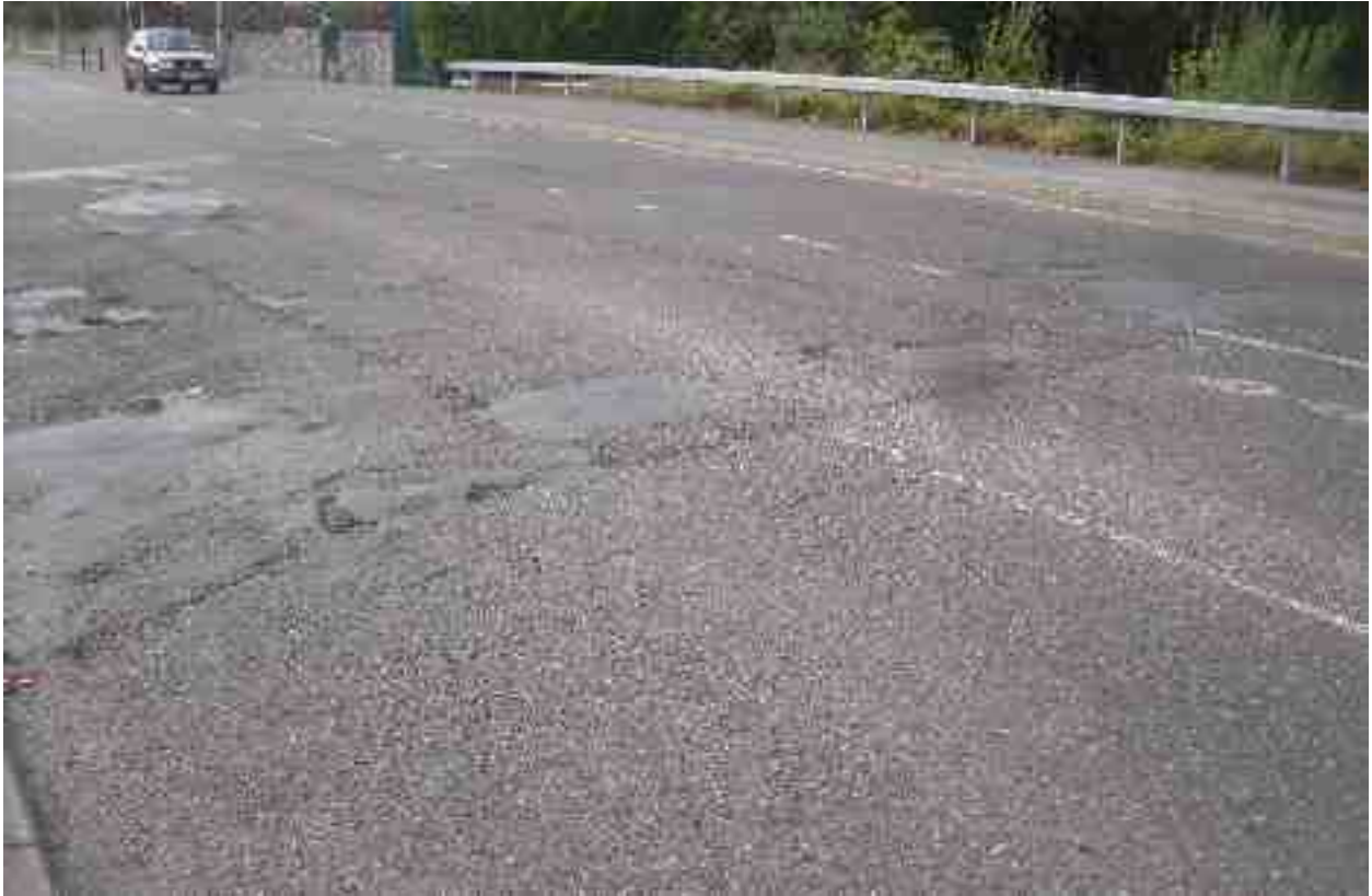
Rating 3: Extensive patching in poor condition
