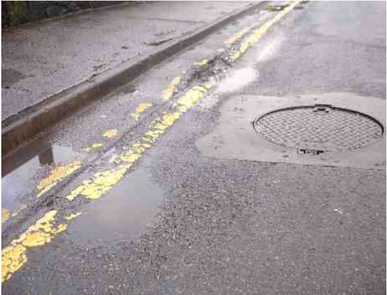
Severe Rutting with uplift of sides in the wheelpath
