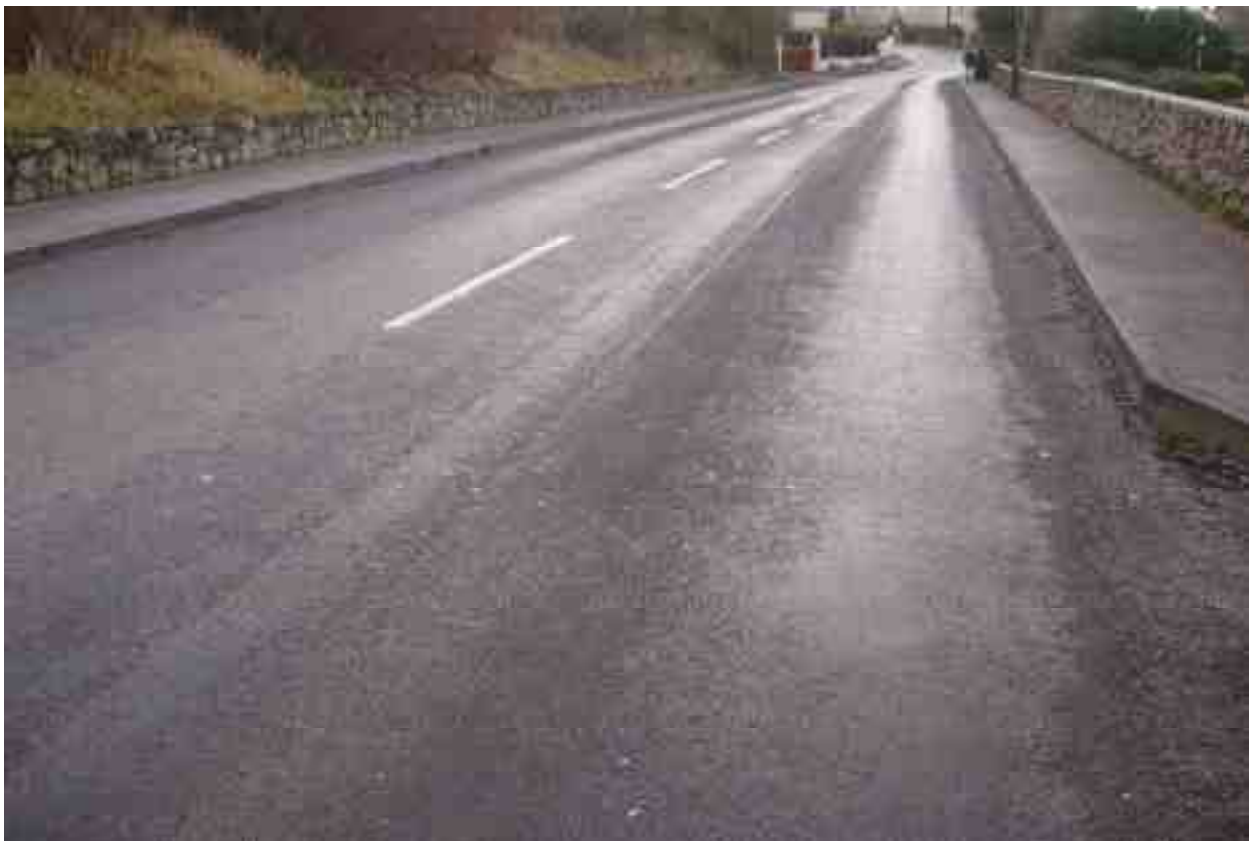
Rating 7: Bleeding in wheelpaths greater than 30% of surface
