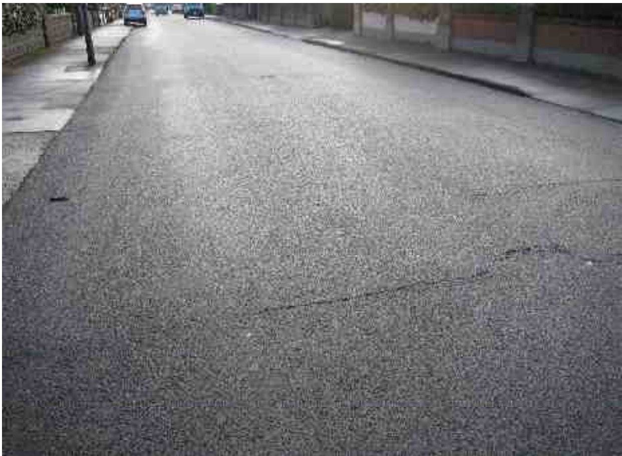
Reflection cracking on new pavement surface
