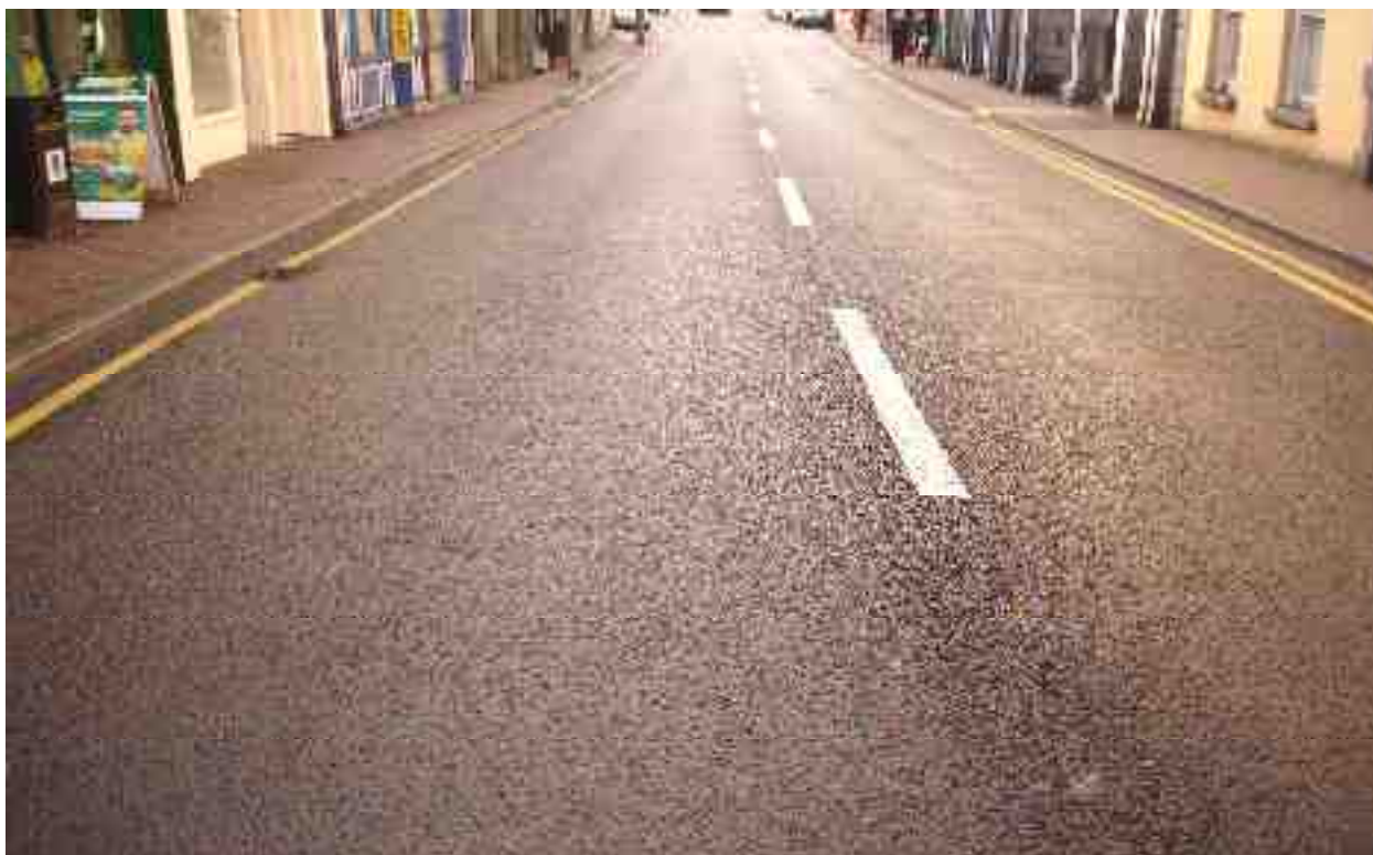
Rating 10: Road with no visible pavement defects, new Clause 942 surface
