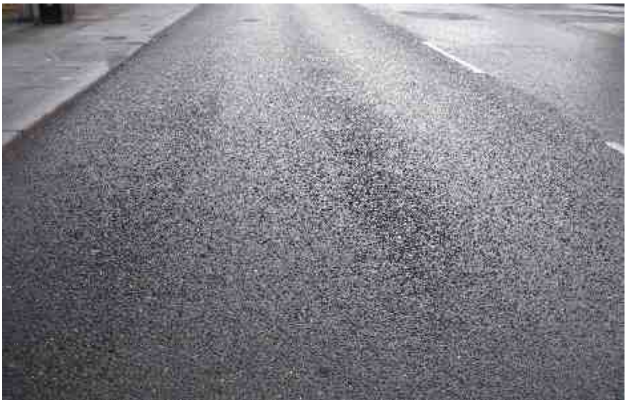
Rating 8: Ravelling evident in wheelpaths, 10% to 30% of surface
