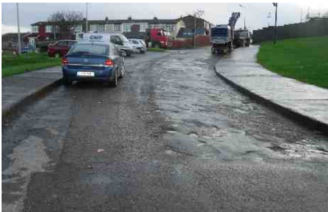
Rating 1: Extensive failed patching, almost total loss of pavement integrity
