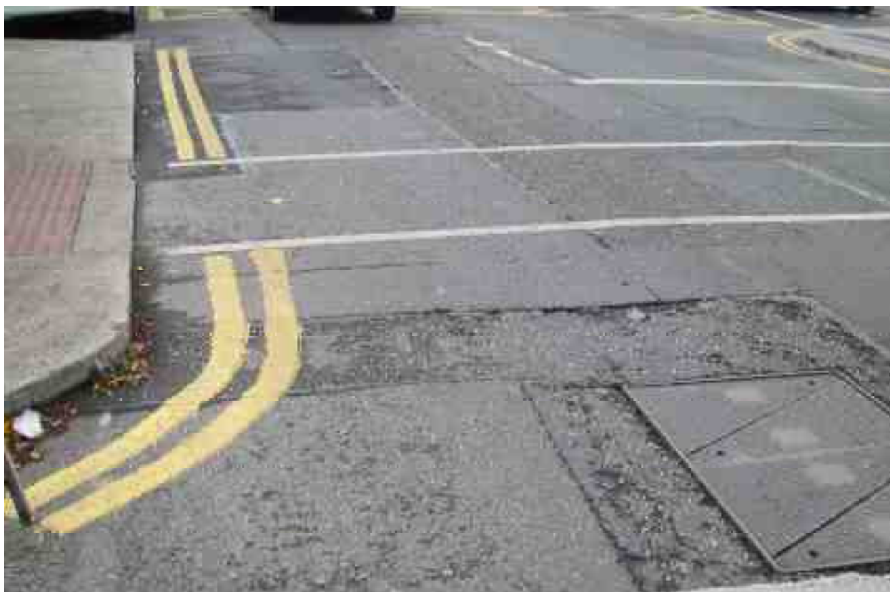
Rating 5: Patching generally in fair condition with signs of distress in vicinity of ironworks
