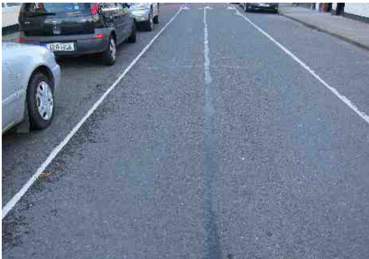
Rating 9: Road with good surface and well sealed joint
