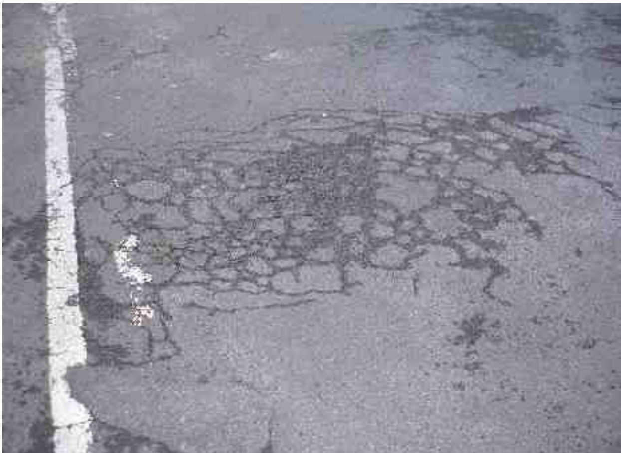
Alligator cracking made more visible by moisture in cracks
