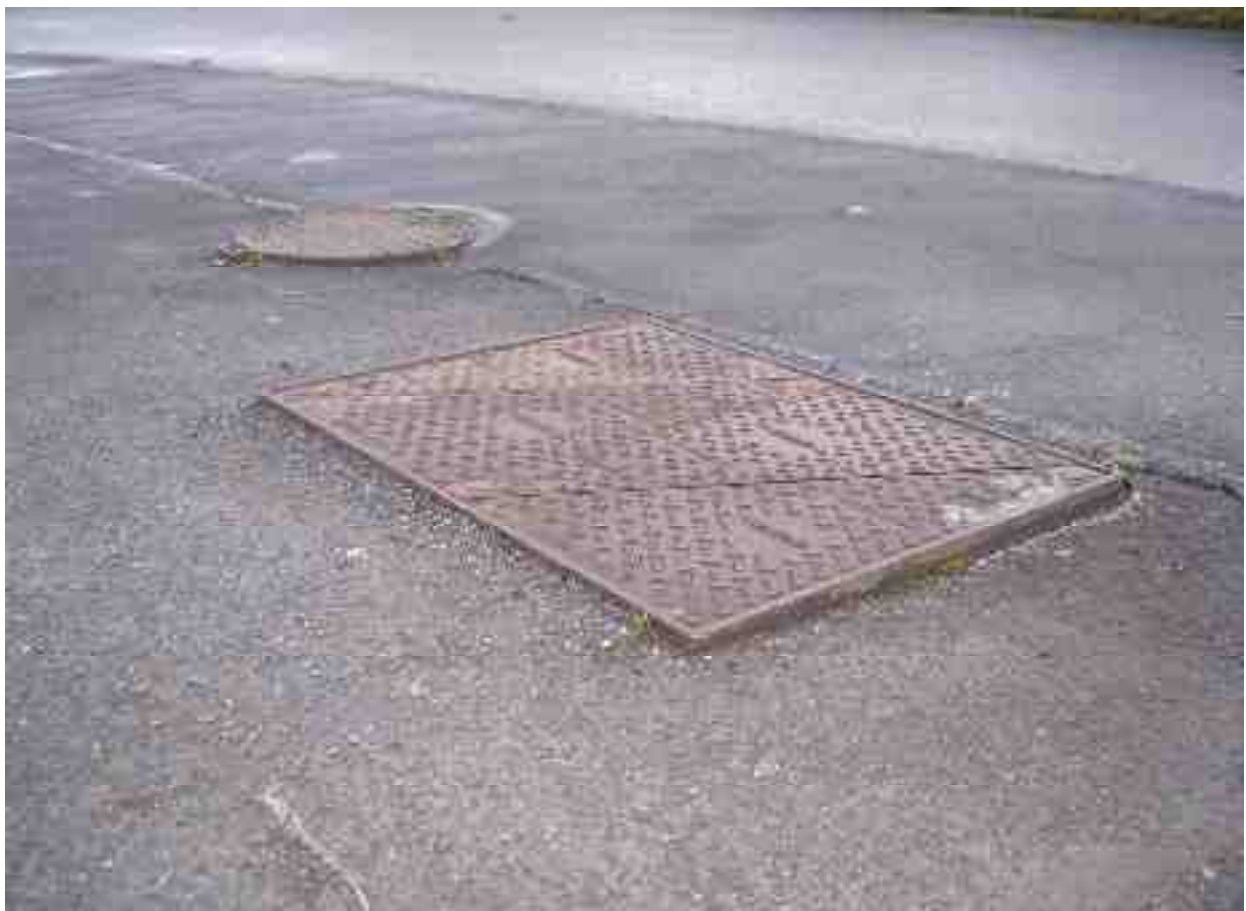
Ironworks above the pavement surface causing poor ride quality
