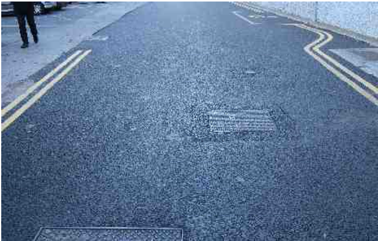
Dual pavement inlet gullies with new well sealed utility cut patch in excellent condition
