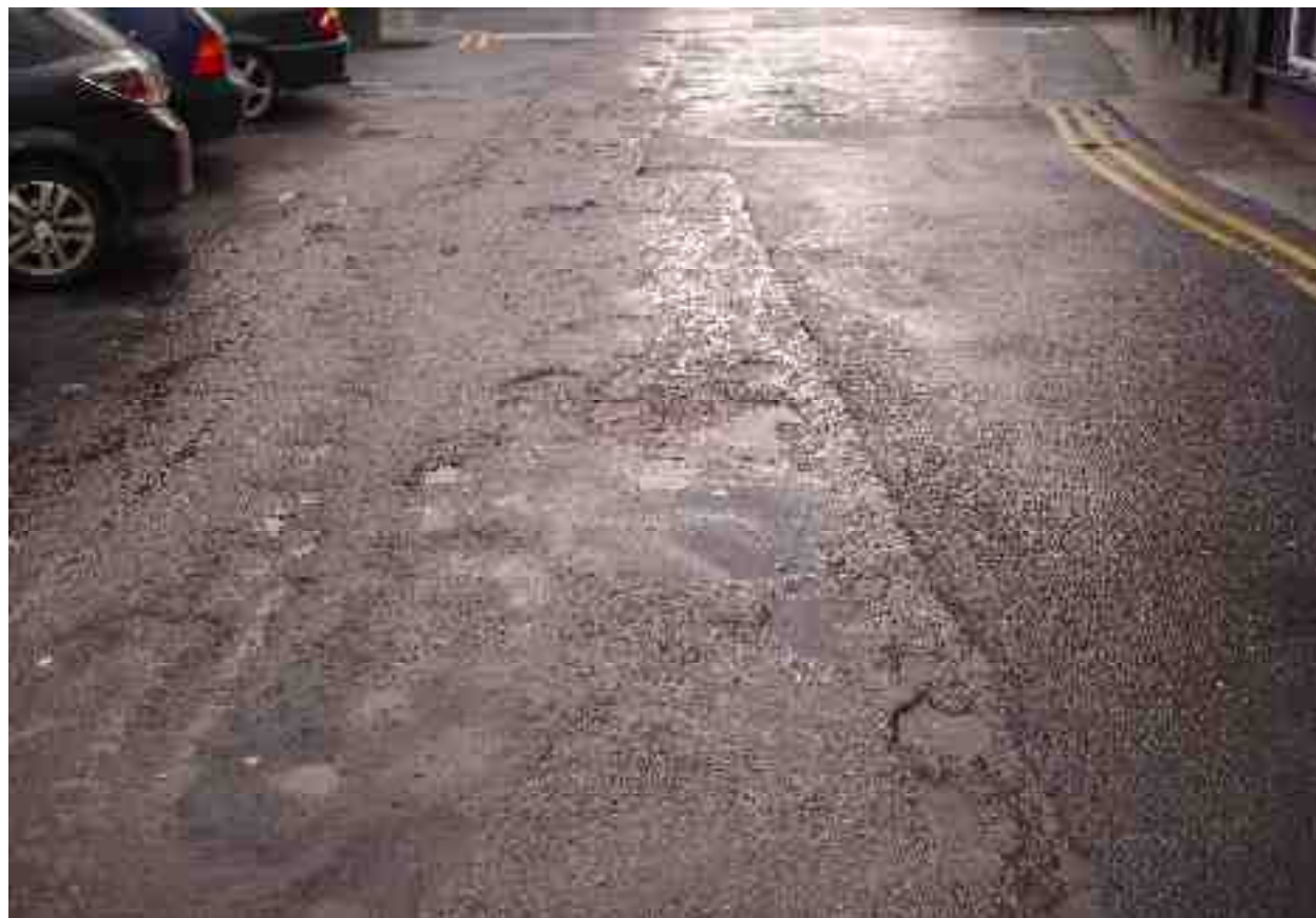
Rating 2: Failed pavement surface with very poor patching
