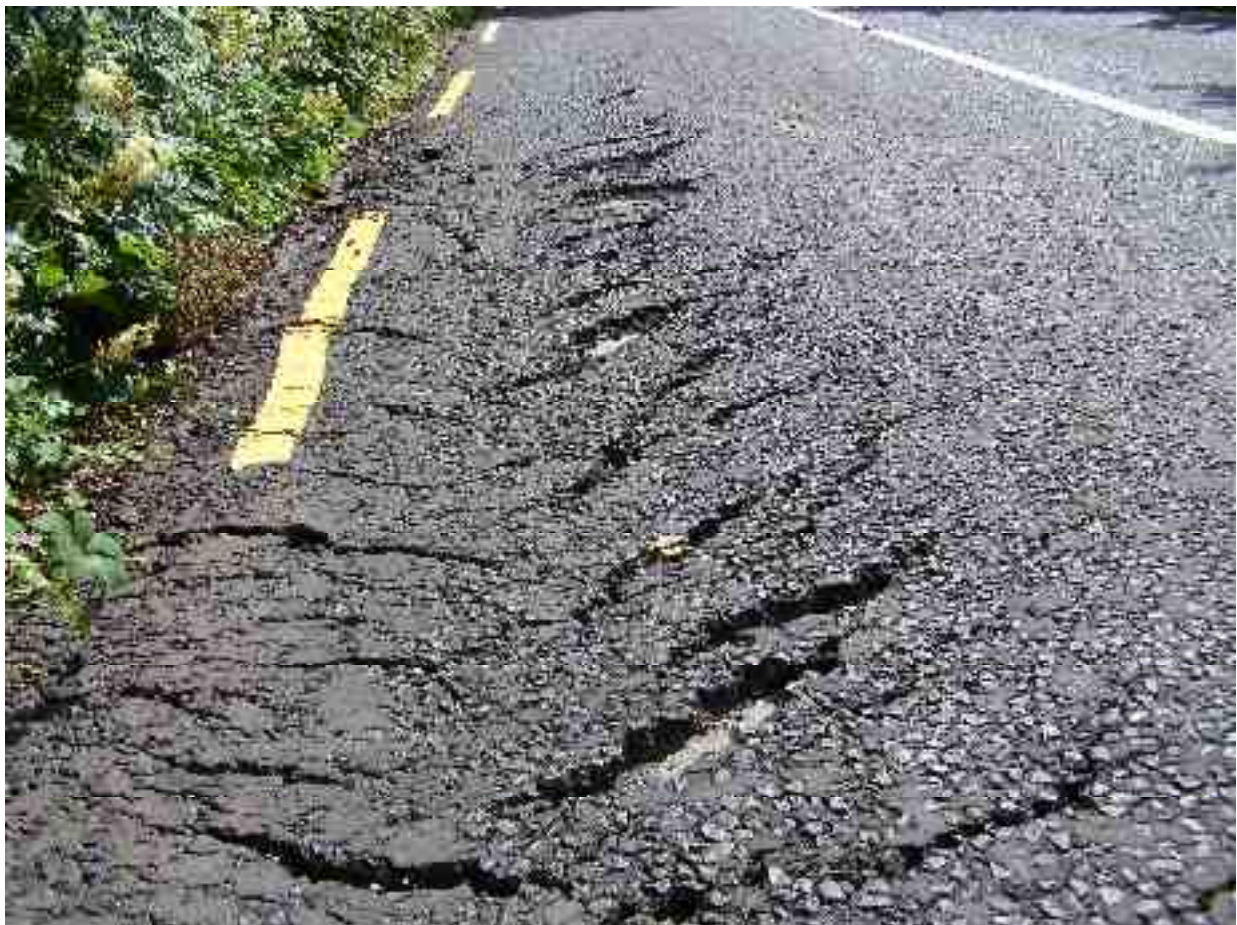
Slippage cracking with underlying stability problems
