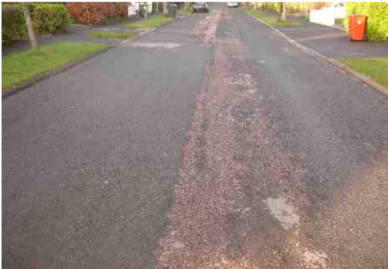
Rating 7: Extensive Ravelling over most of pavement surface (> 30%)
