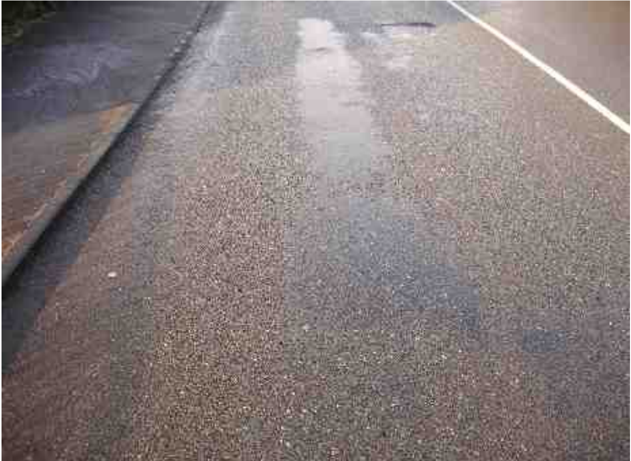
Bleeding: Dark, shiny areas show where binder has worked to the surface along the wheelpath
