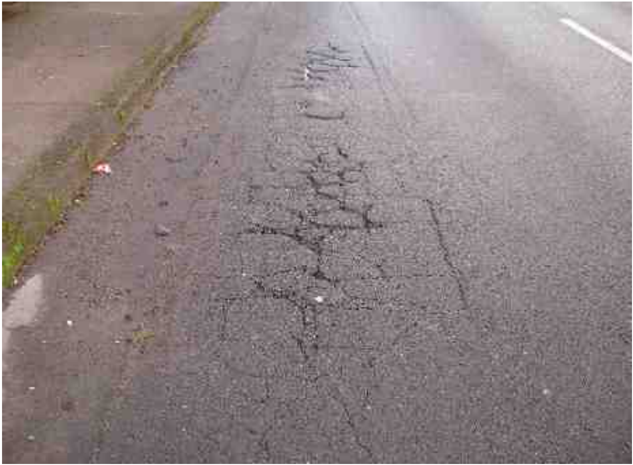
Open and spalled alligator cracking in the wheelpath
