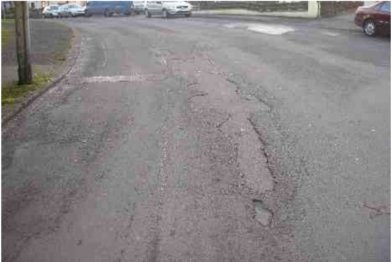
Rating 7: Ravelling or stripping of material from pavement surface
