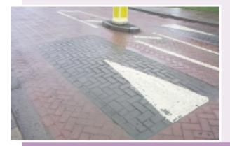
Bitumen based material with block pattern
