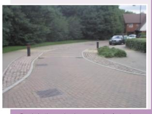
Bends in the road reduce excessive forward visability and control speed on new roads
