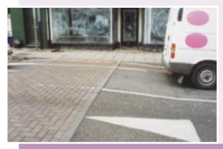
Ramp with composite construction and 'lip' between materials
