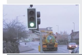
Cranked signal poles allow push buttons to be sited close to the crossing and provide clearance from passing vehicles without obstructing the footway
