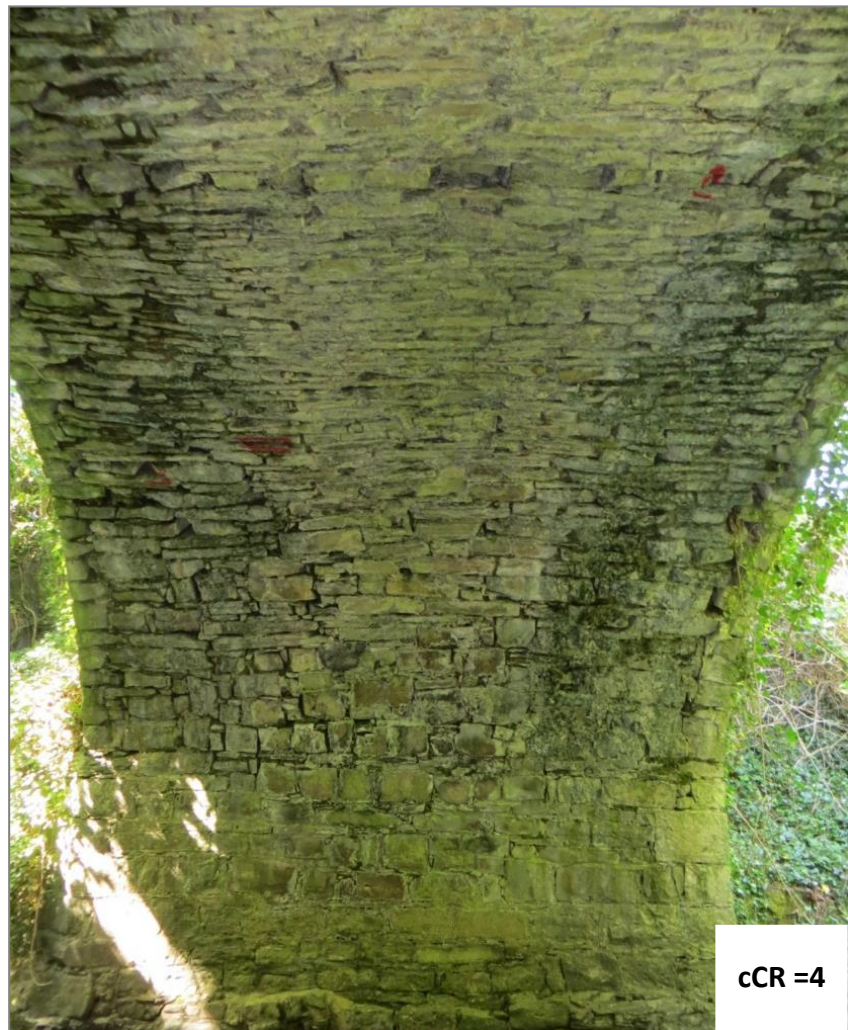
Figure A.25 – Cracked Arch
