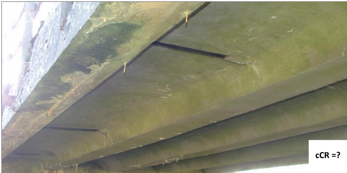
Figure A.27 – Cracks in Soffit
