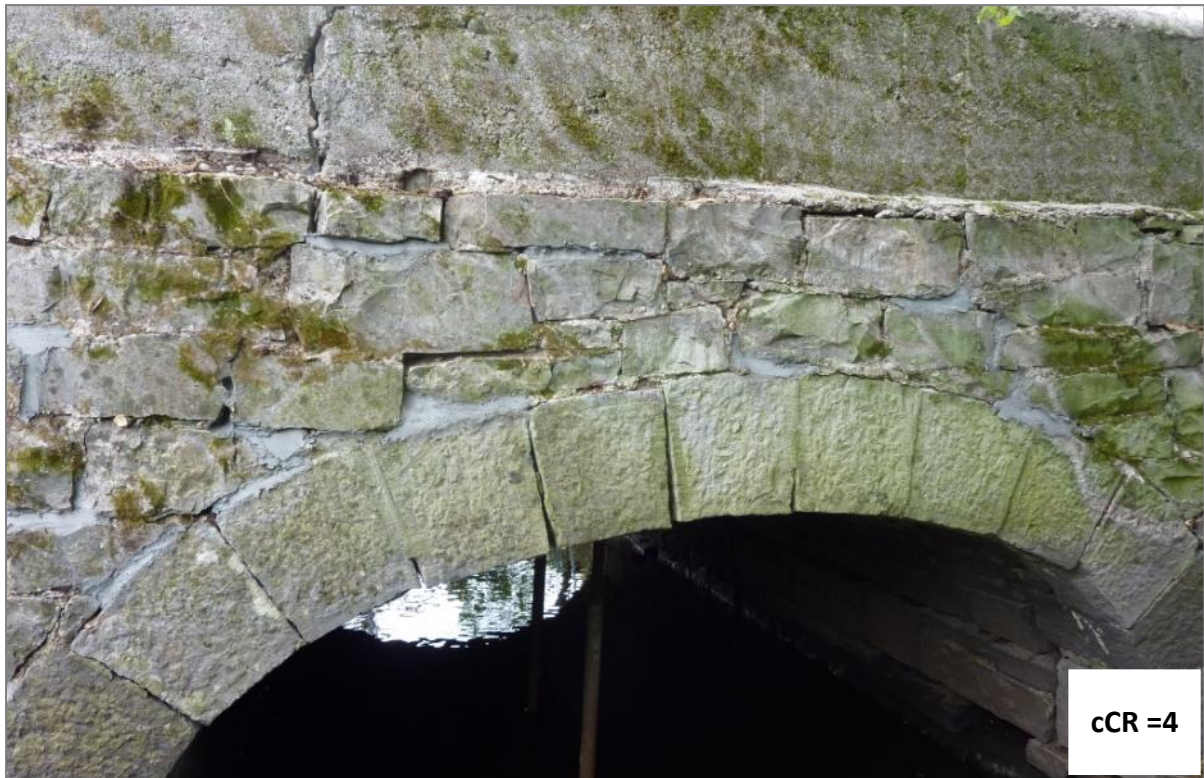
Figure A.22 – Transverse Cracks in External Voussoirs
