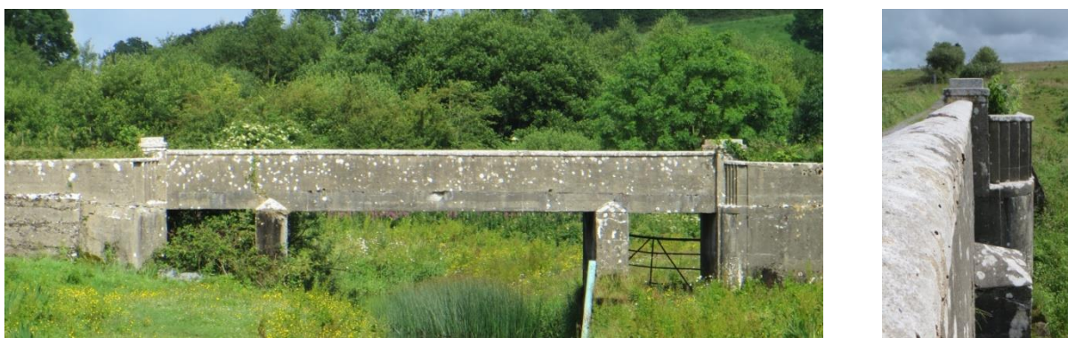
Figure 7.1 – Example of early rural in-situ concrete bridge with decorative parapet feature at abutments
