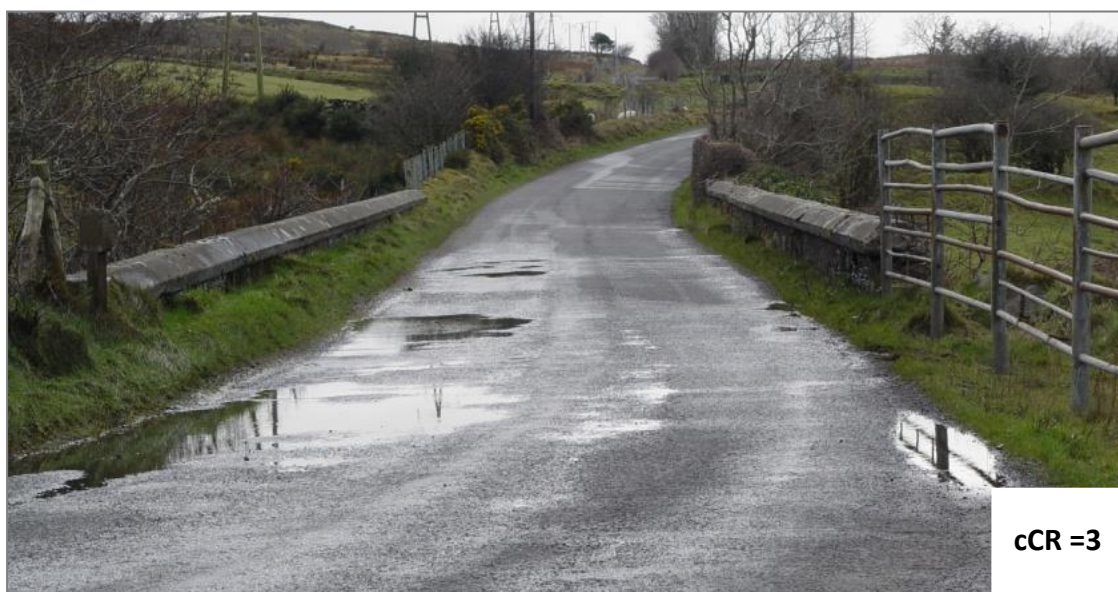
Figure A.2 – Surface Water Ponding (and permeable grass verges)
