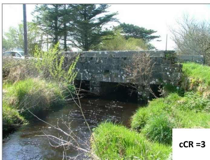
Figure A.31 – Compromised Concrete Slab Deck
