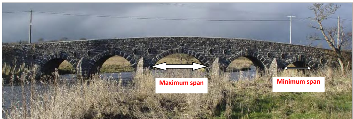
Figure 3.18 – Bridge in Elevation Depicting Max/Min Spans
