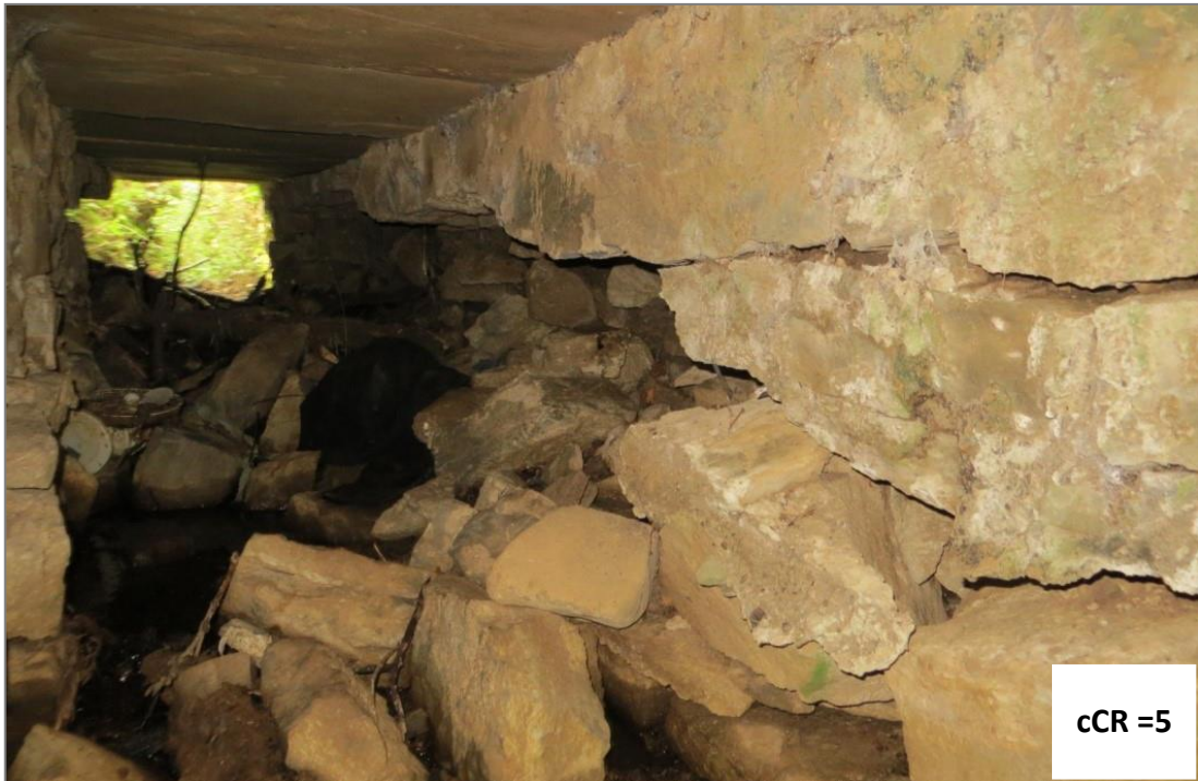
Figure A.15 – Abutment Failure
