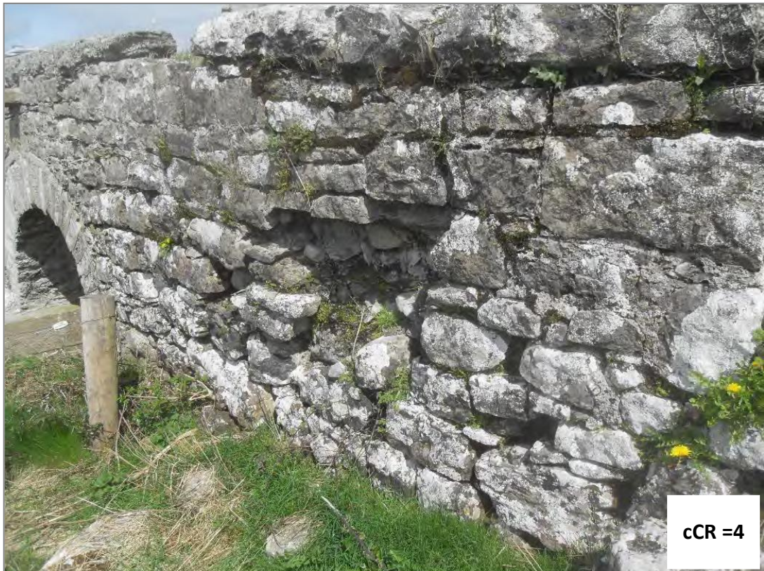
Figure A.11 – Collapsing Outer Stone on Wingwall
