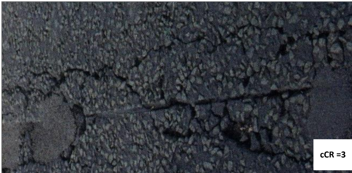
Figure A.40 – Breakdown in Buried Expansion Joint
