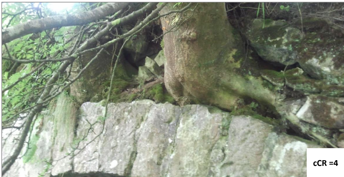
Figure A.20 – Tree Roots Boring into Barrel
