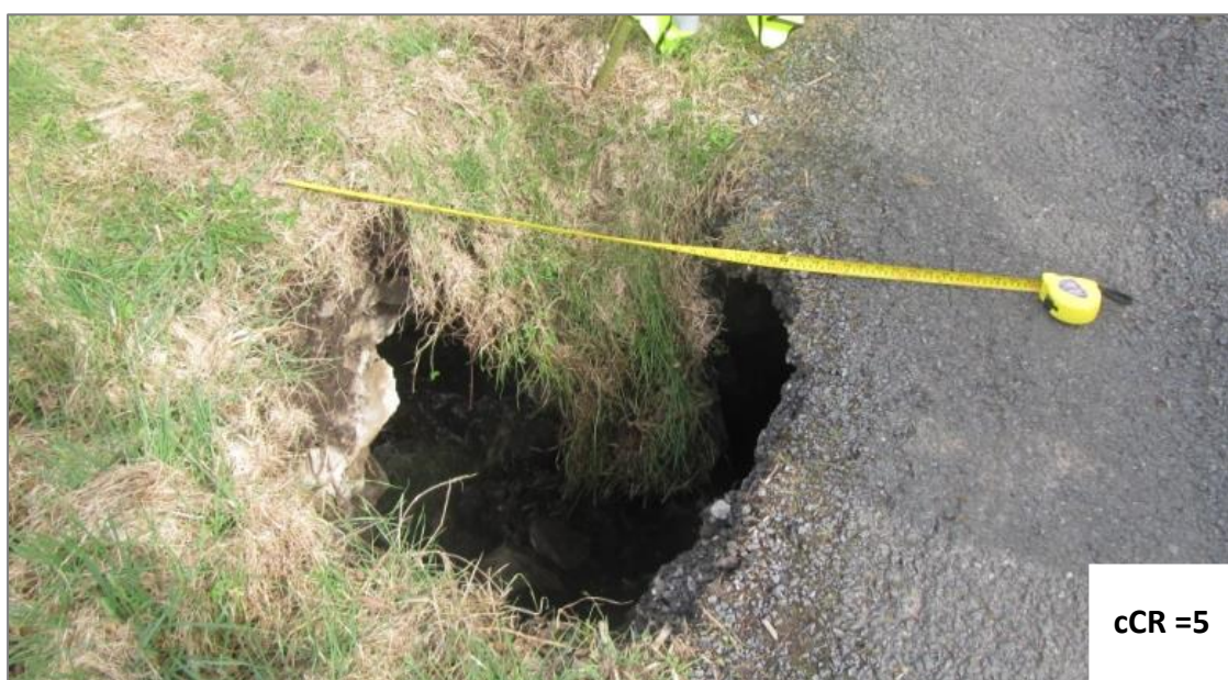
Figure A.1 – Hole in Carriageway to River Bed Below
