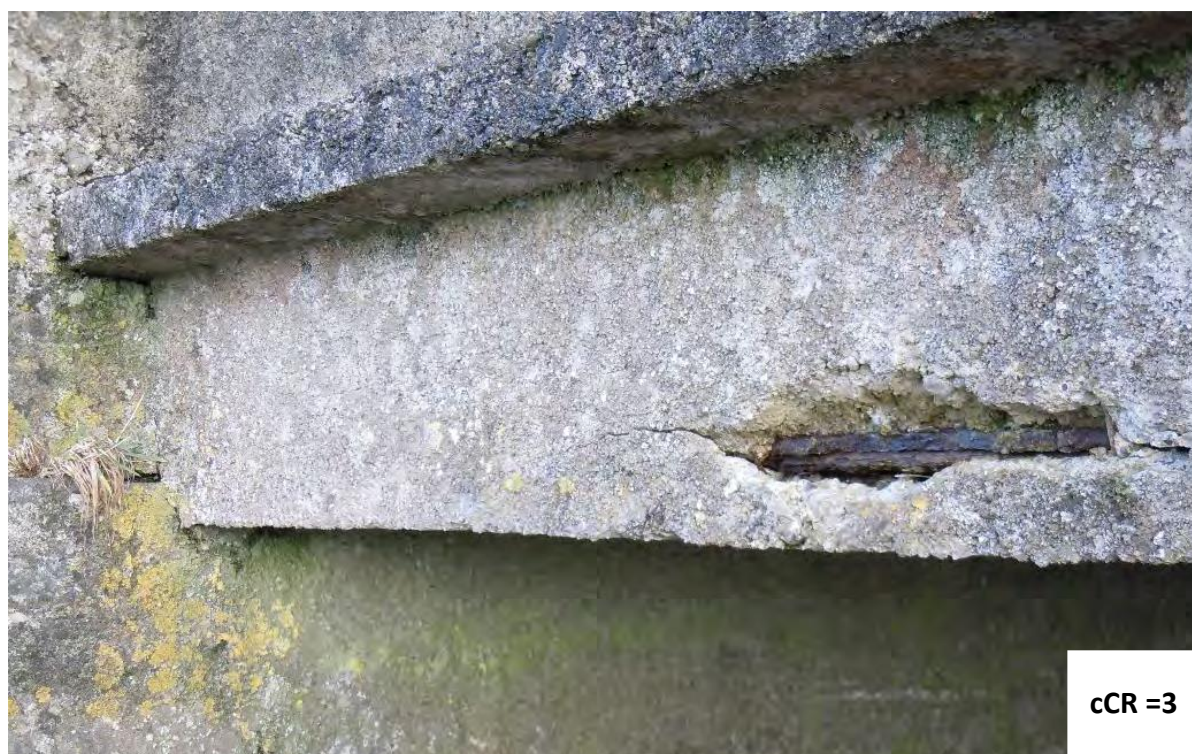
Figure A.30 – Exposed Steel Flange
