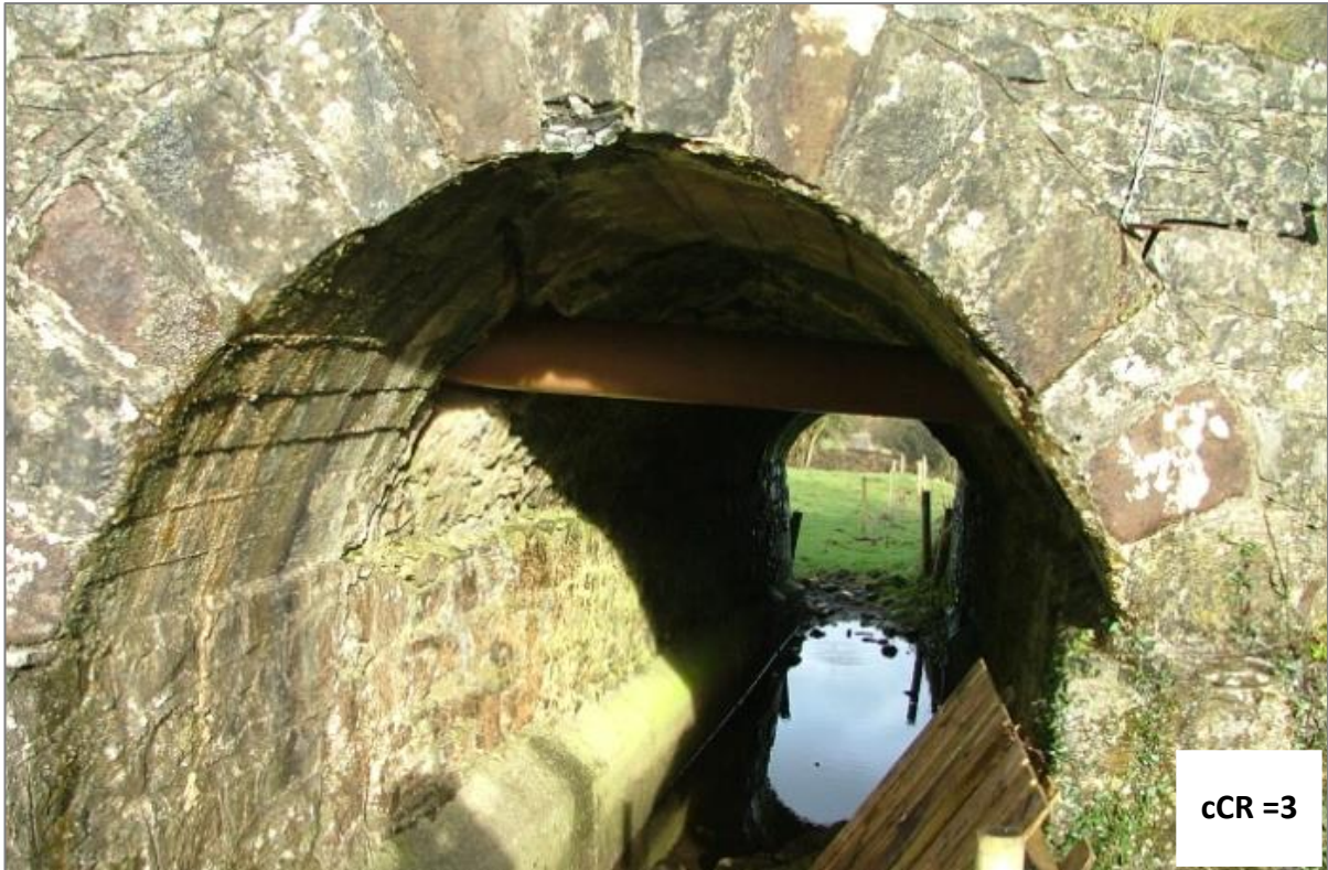
Figure A.43 – Services Causing Damage
