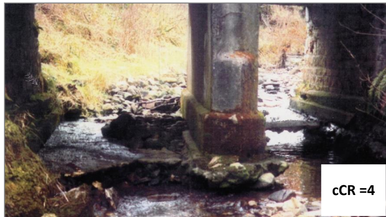
Figure A.35 – Bed Protection Failure
