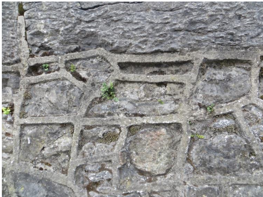
Figure 7.4 – Inappropriate opc 'strap' Pointing
