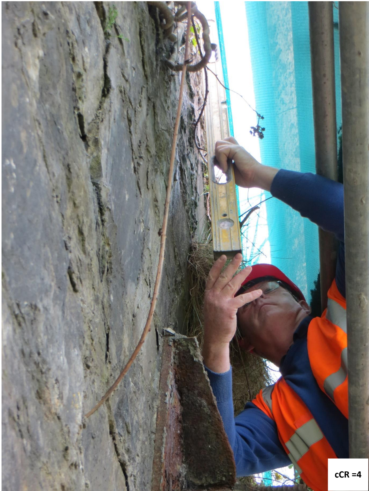
Figure A.21 – Leaning and Bulging Spandrel Wall
