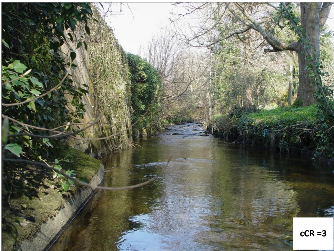
Figure A.12 – Missing Stone at Water Level
