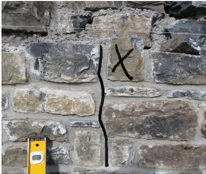
Figure 7.6 – Inappropriate Masonry Repair Example
