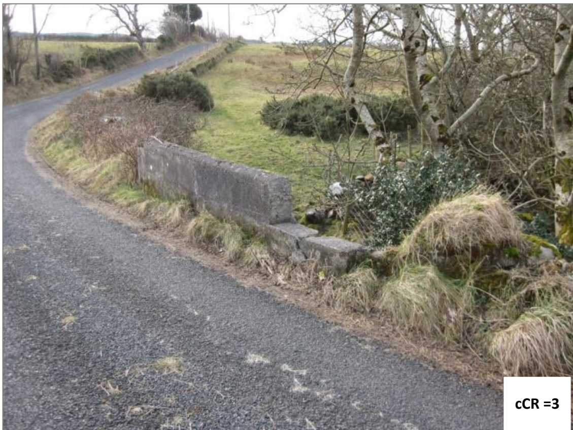
Figure A.4 – Concrete Parapet Partially Missing
