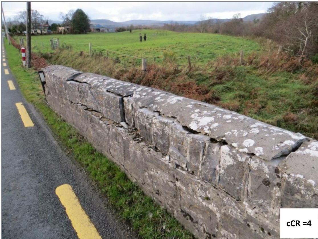
Figure A.5 – Impact Damage to Masonry Parapet
