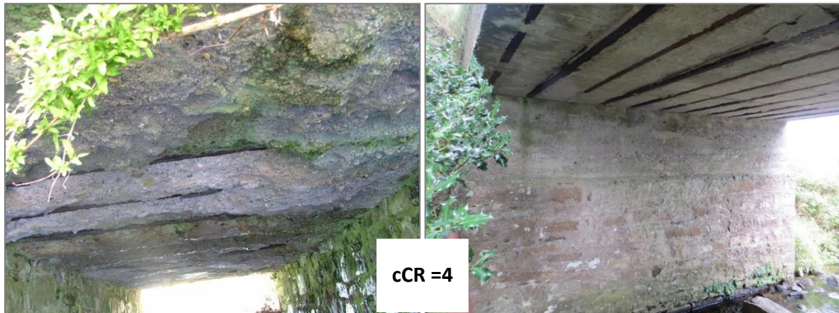
Figure A.32 – Compromised Flanges
