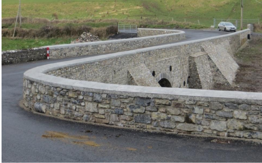
Figure 7.5 – Good Masonry Parapet Wall
