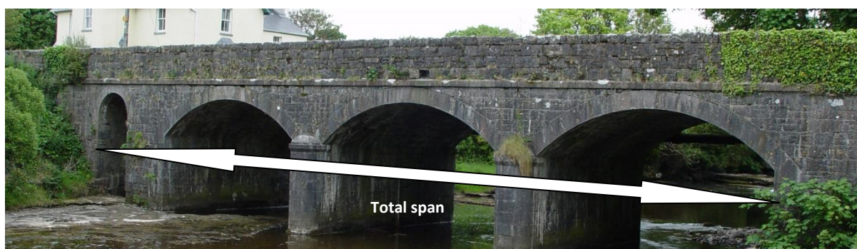
Figure 3.16 – Bridge in Elevation Depicting Total Span
