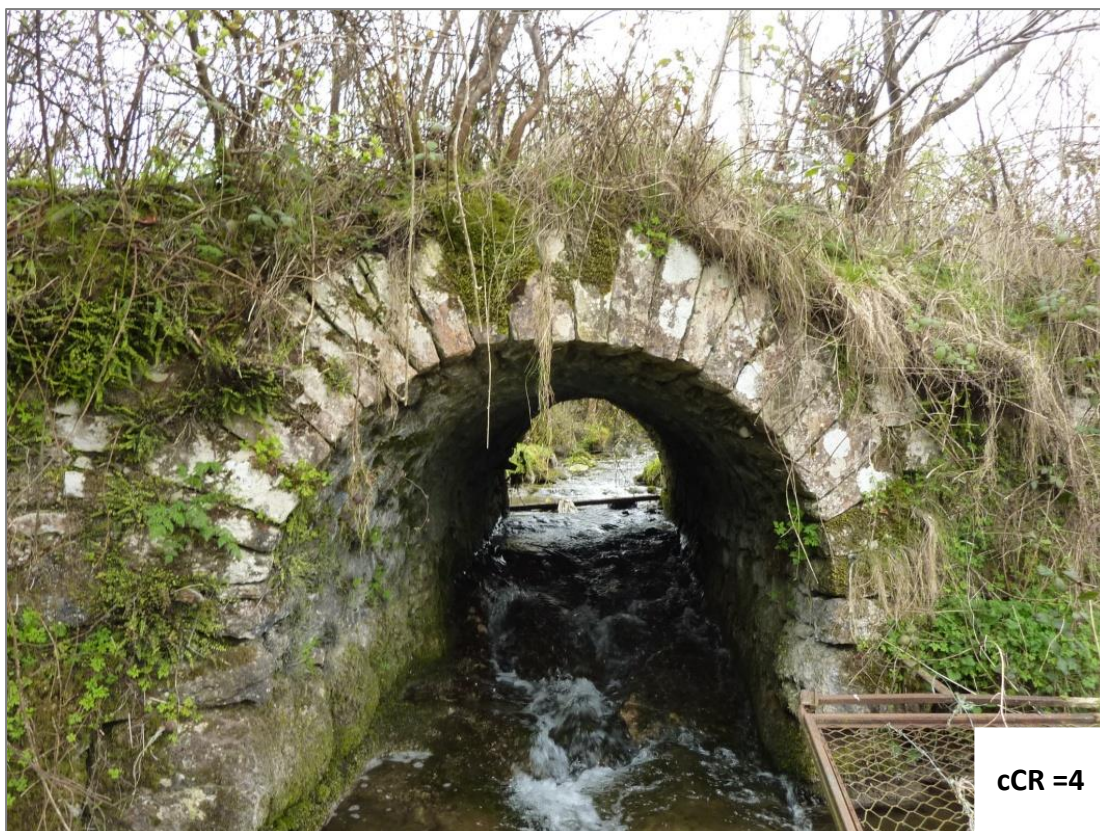
Figure A.7 – Missing Parapets and Spandrels
