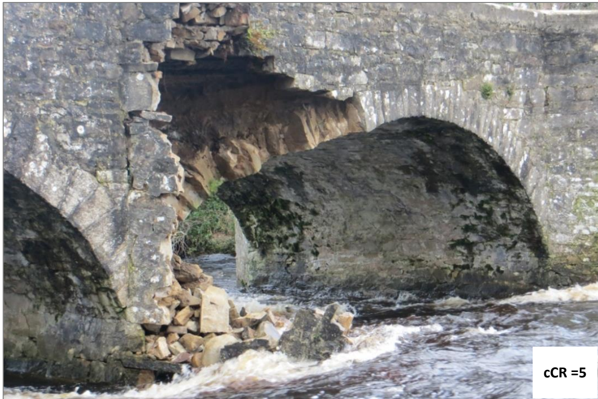
Figure A.19 – Scour at Pier Head and Pier Causing Collapse of Cutwater, Part of Pier and Arch
