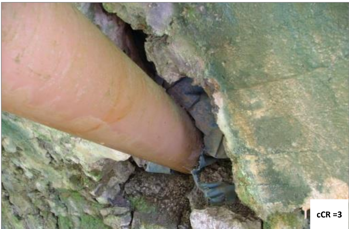
Figure A.44 – Pipe Smashed through Arch, poor repair work, if any.
