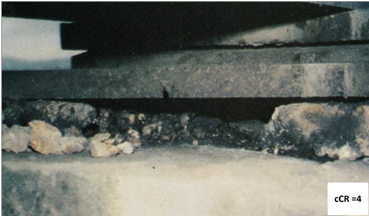
Figure A.39 – Bearing Seat Failure.
