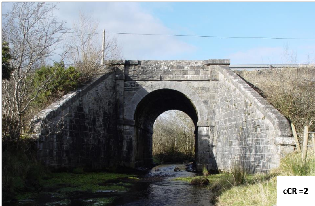
Figure A.10 – Masonry Wingwalls and Retaining Walls
