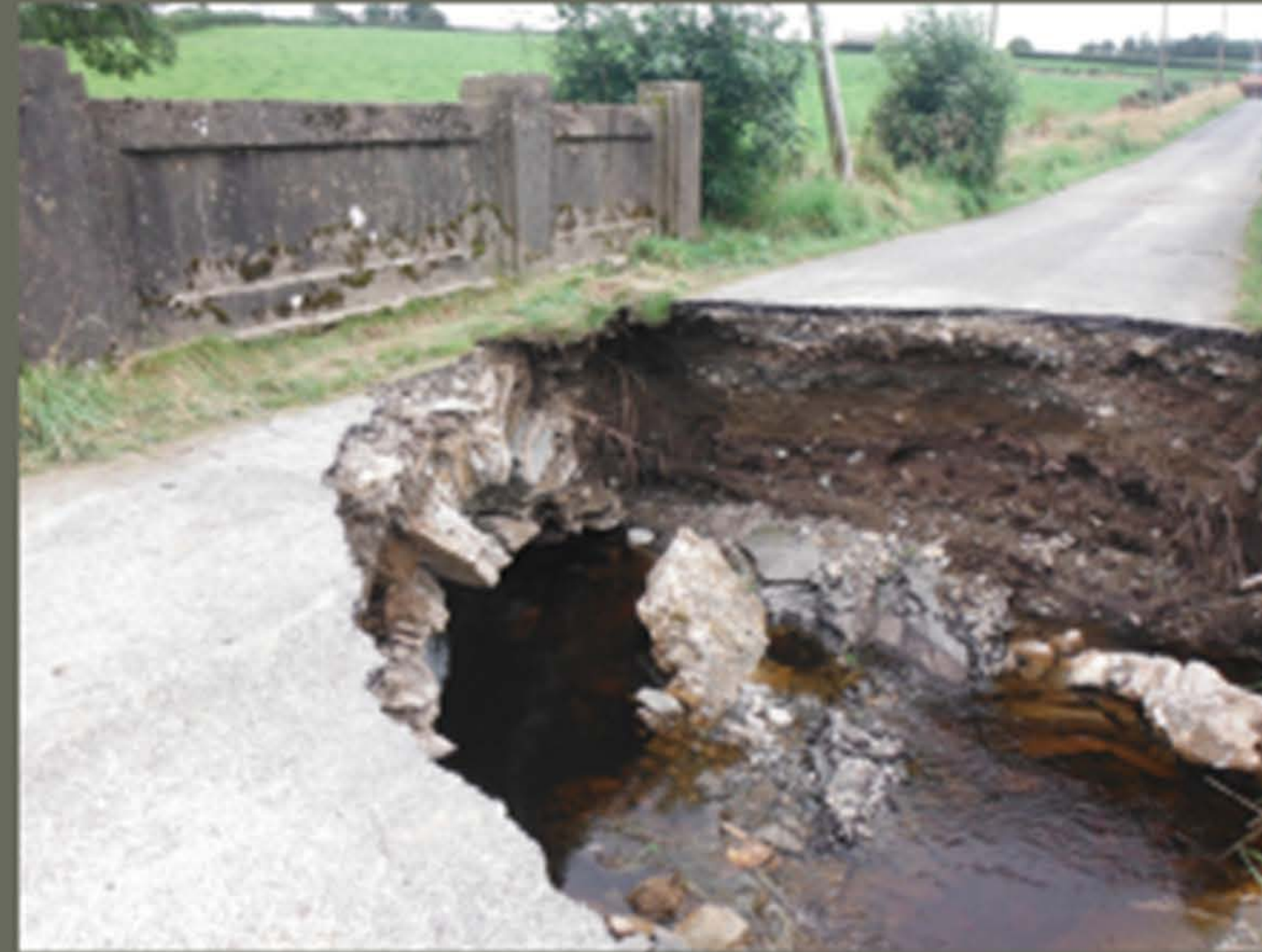
Extreme example - potential for further masonry to fall or sides to collapse
