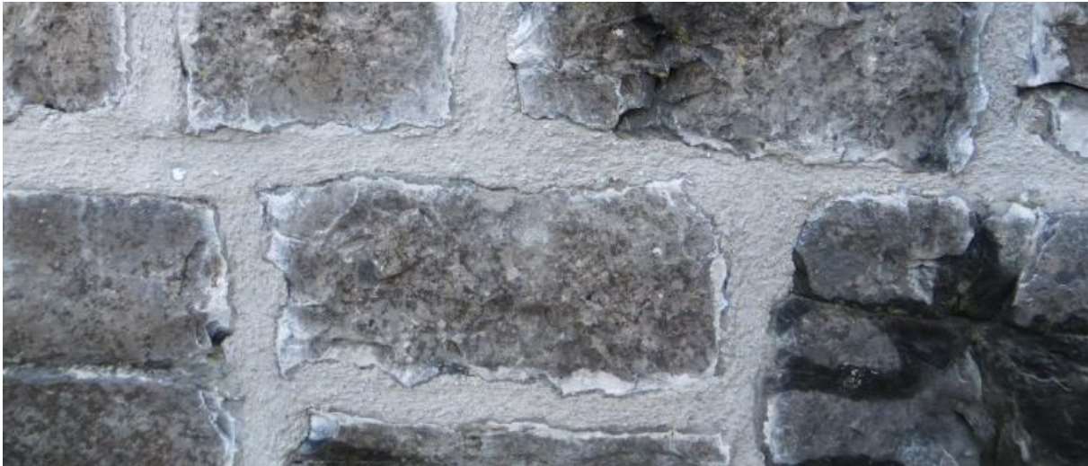
Figure 7.3 – Appropriate Lime Pointing
