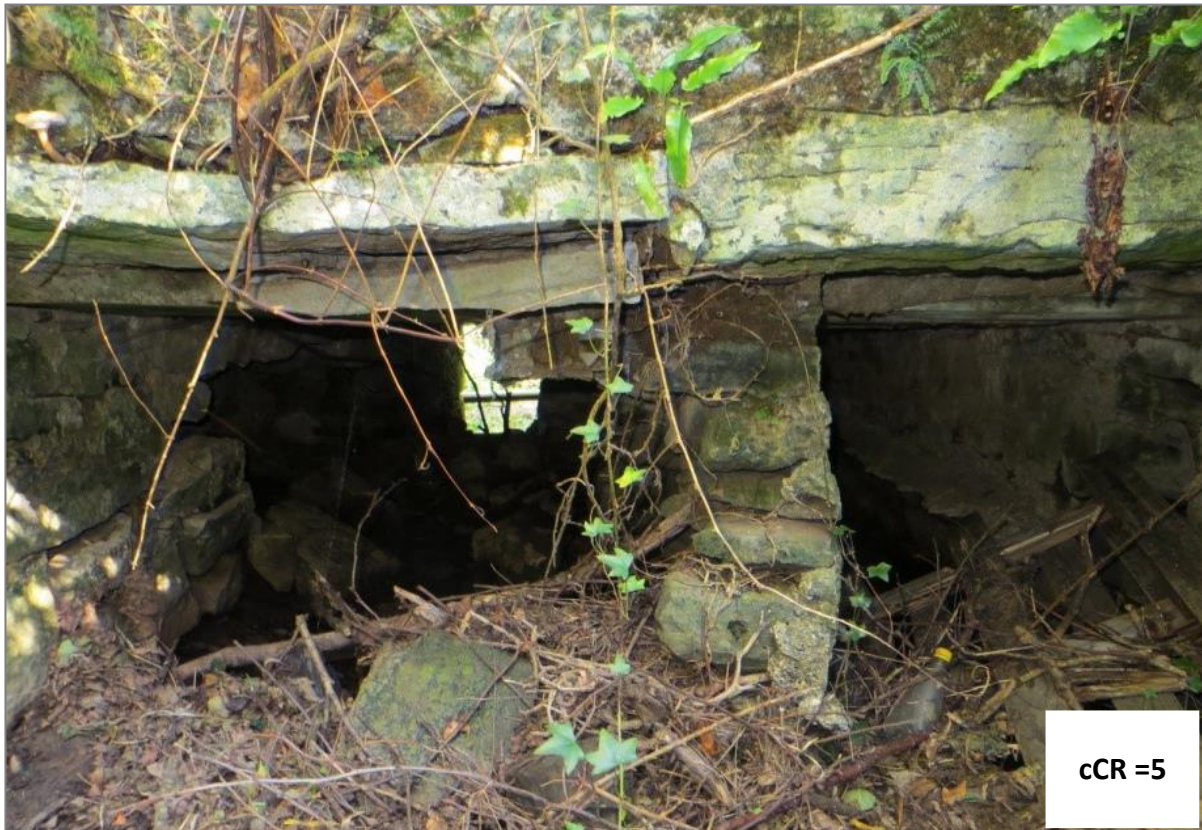
Figure A.17 – Collapsing, buckling pier and stone lintels failing and falling
