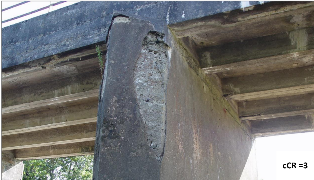
Figure A.16 – Cement Render Failing Exposing Weak Mass Concrete to Greater Weathering
