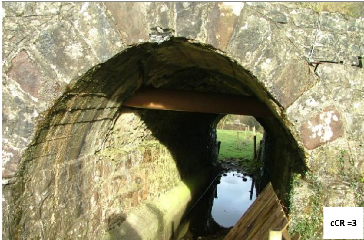
Figure A.43 – Services Causing Damage
