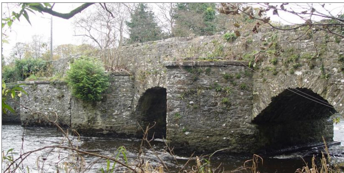
Abbeytown Bridge, Boyle, County Roscommon. Open to vehicular traffic and celebrating its 800th birthday about now! Concrete skirts to the piers were added during the mid-twentieth century but, other than that, the bridge appears to be essentially 'as built'.
