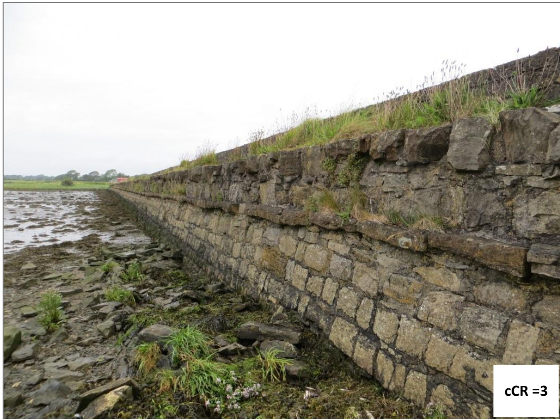
Figure A.9 – Revetment Supporting Road in Tidal Zone (masonry bridge out of view)
