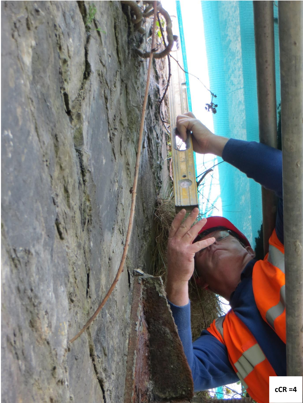
Figure A.21 – Leaning and Bulging Spandrel Wall
