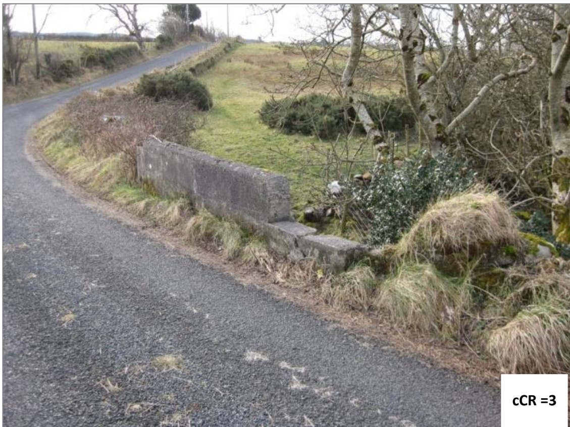
Figure A.4 – Concrete Parapet Partially Missing
