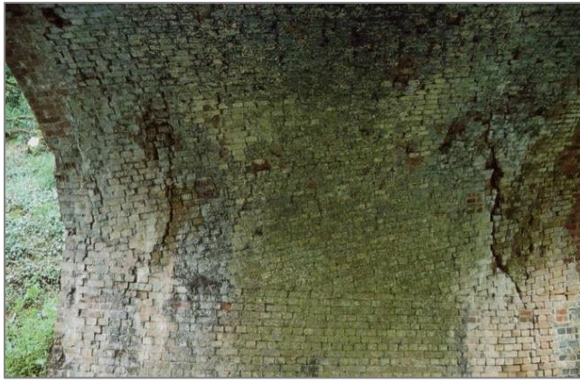
Bridge arch with various longitudinal cracks, separating the arch into individual sections
