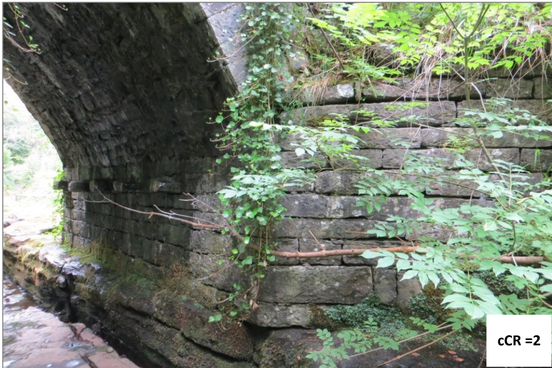
Figure A.13 – River training wall upstream and contiguous with abutment
