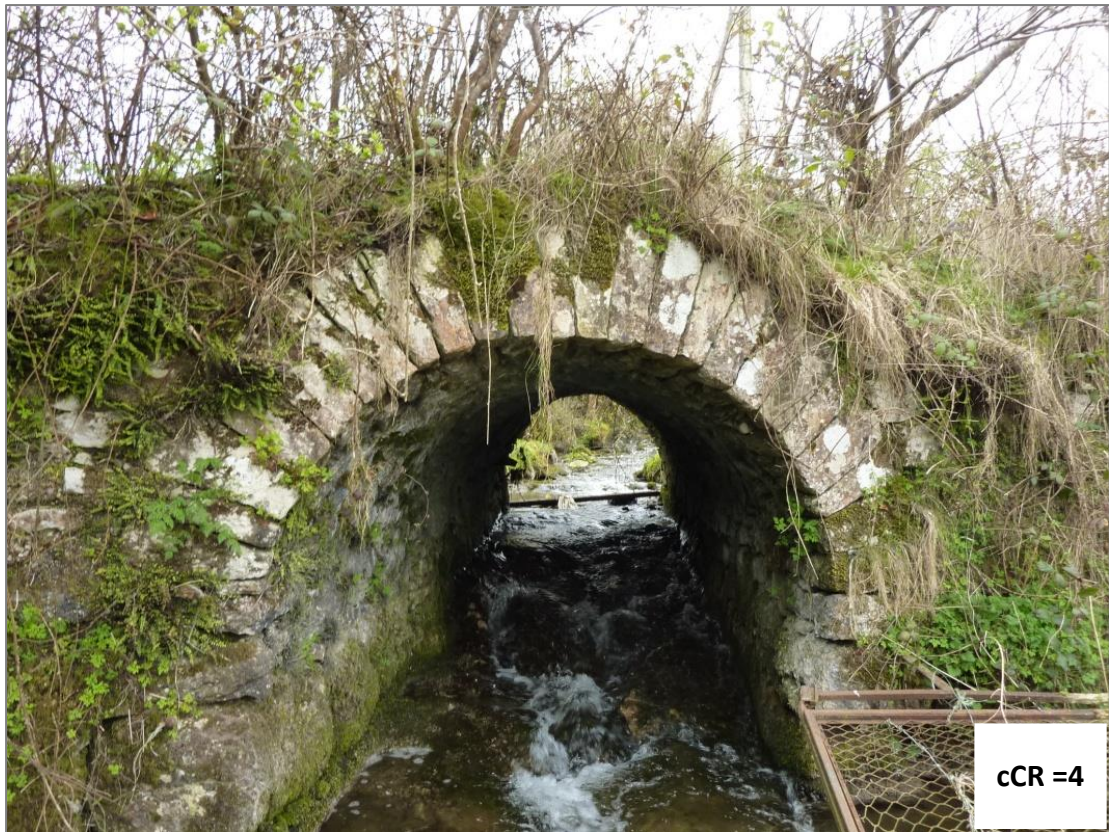
Figure A.7 – Missing Parapets and Spandrels
