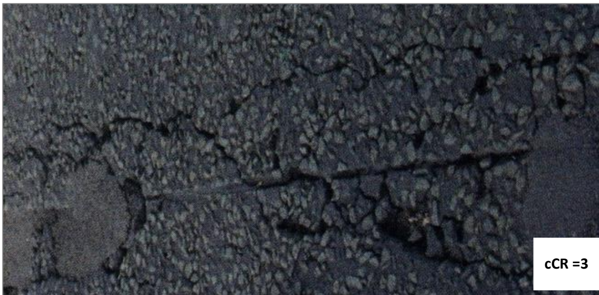
Figure A.40 – Breakdown in Buried Expansion Joint
