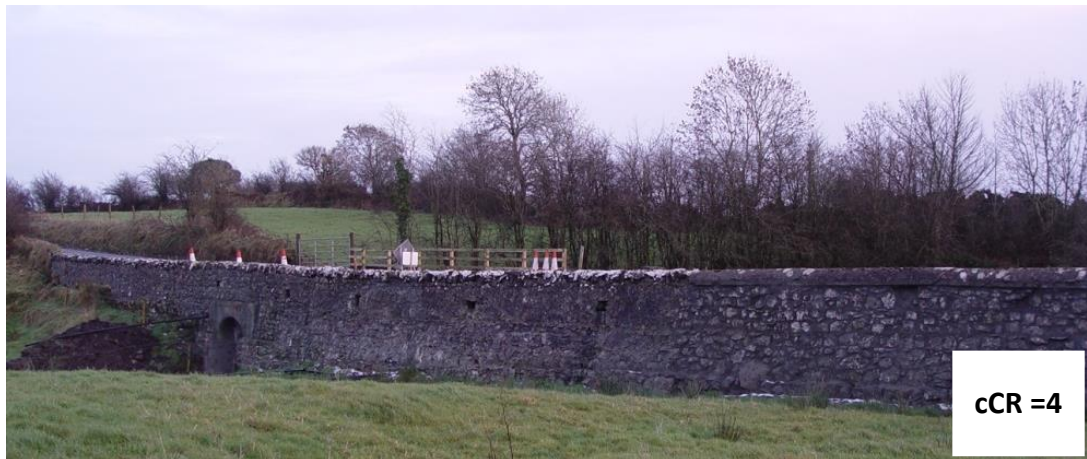
Figure A.8 – Bridge with Sloping Retaining Wall
