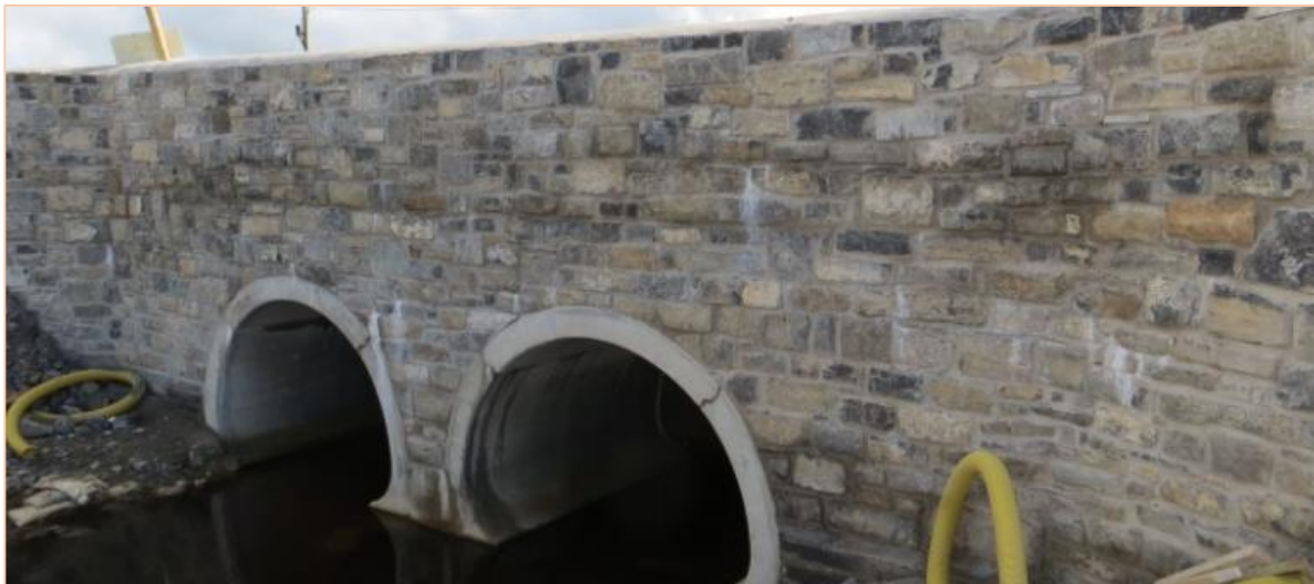
Precast arch units e.g. Matiere arch system 2no.x 2.2m span
