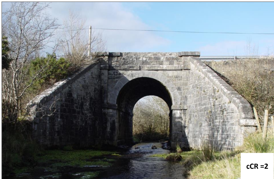
Figure A.10 – Masonry Wingwalls and Retaining Walls
