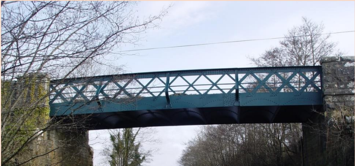
Wrought iron lattice girder 1881
