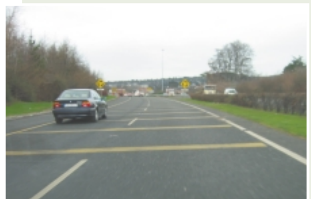
Transverse strips on roundabout approach
