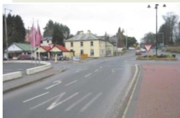
Roundabout without adequate entry deflection
