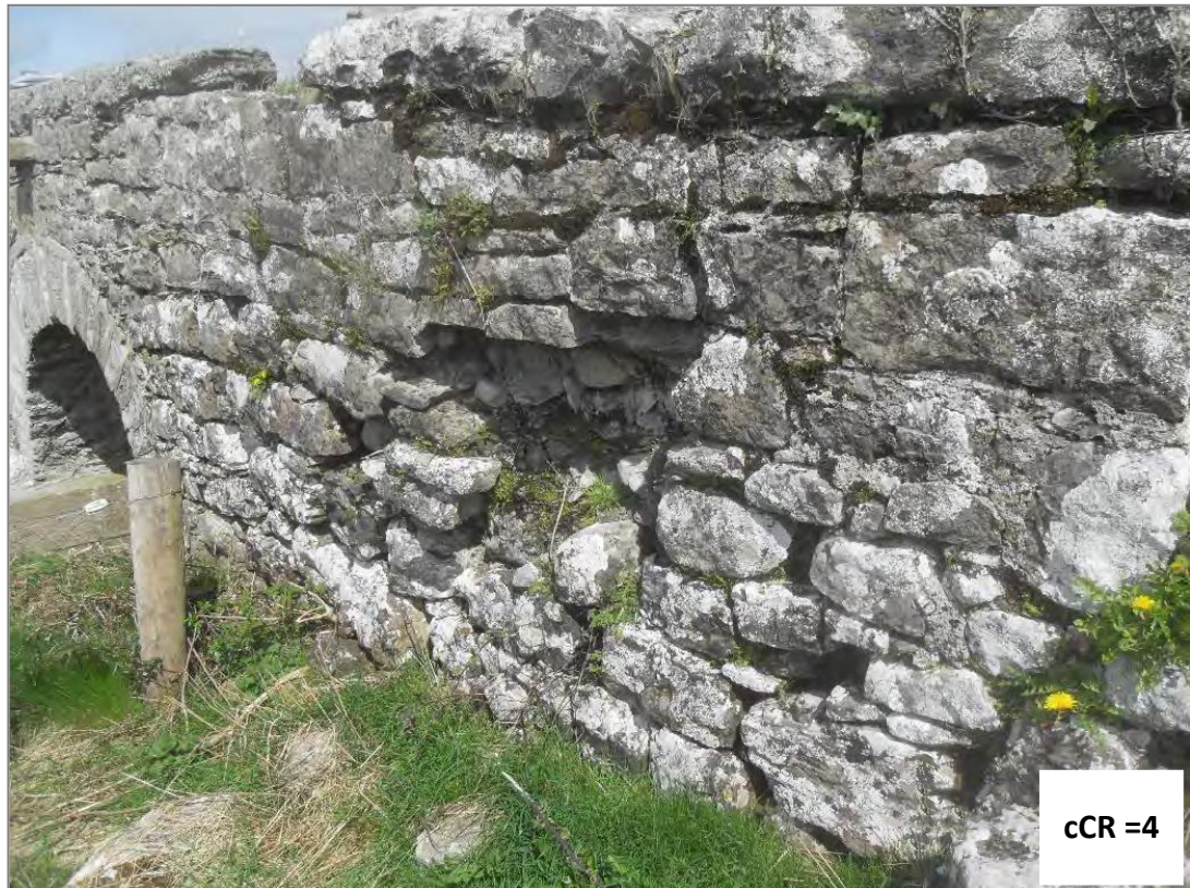
Figure A.11 – Collapsing Outer Stone on Wingwall
