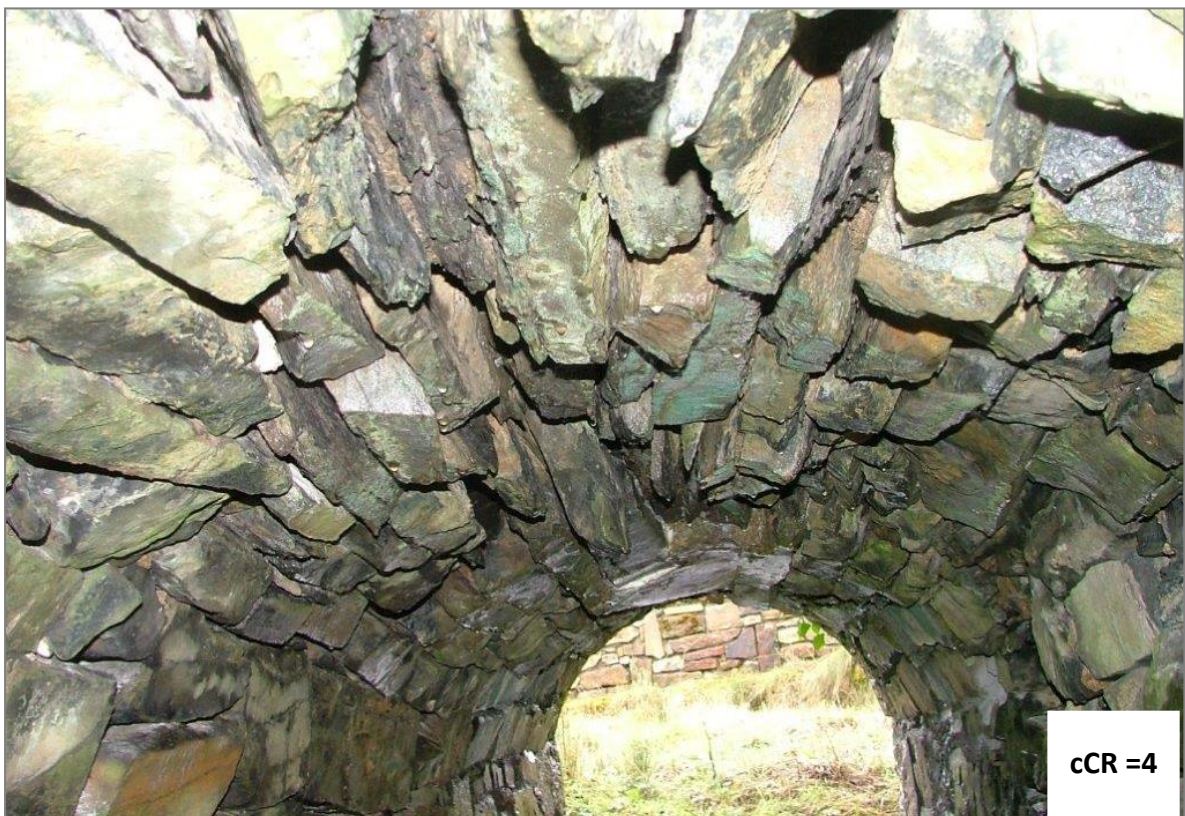
Figure A.23 – Missing Mortar, Sagging and Stone Slippage
