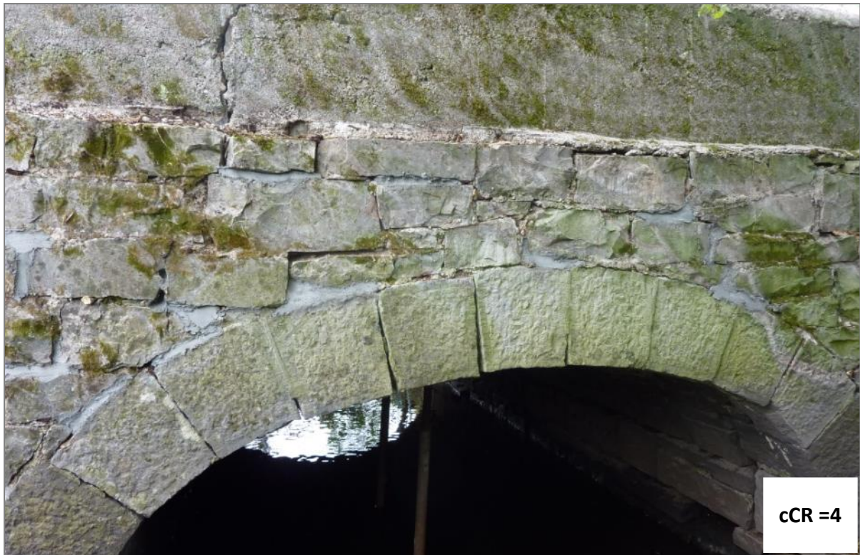
Figure A.22 – Transverse Cracks in External Voussoirs
