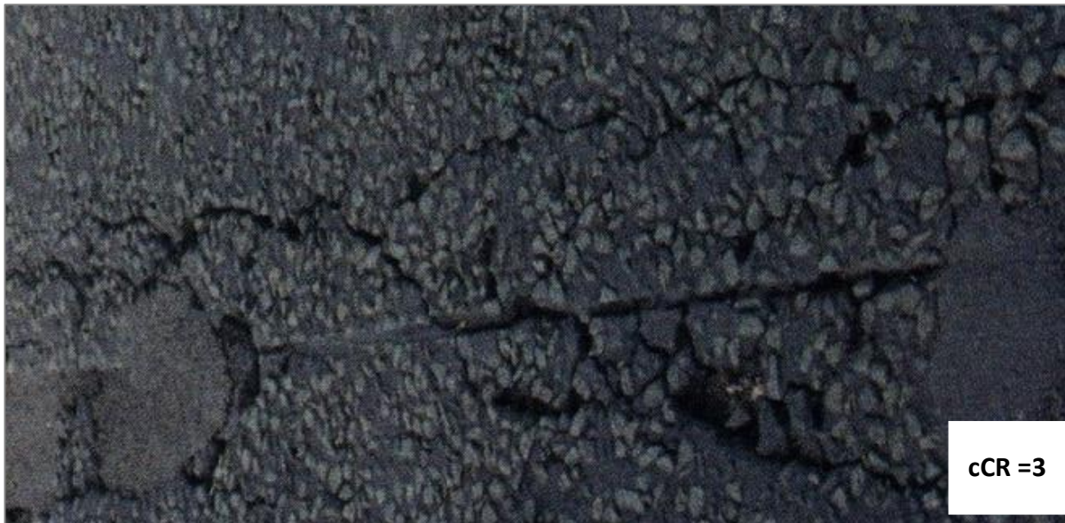
Figure A.40 – Breakdown in Buried Expansion Joint
