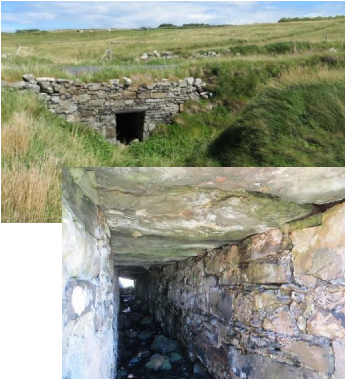
Figure 3.11 – Masonry Clapper
