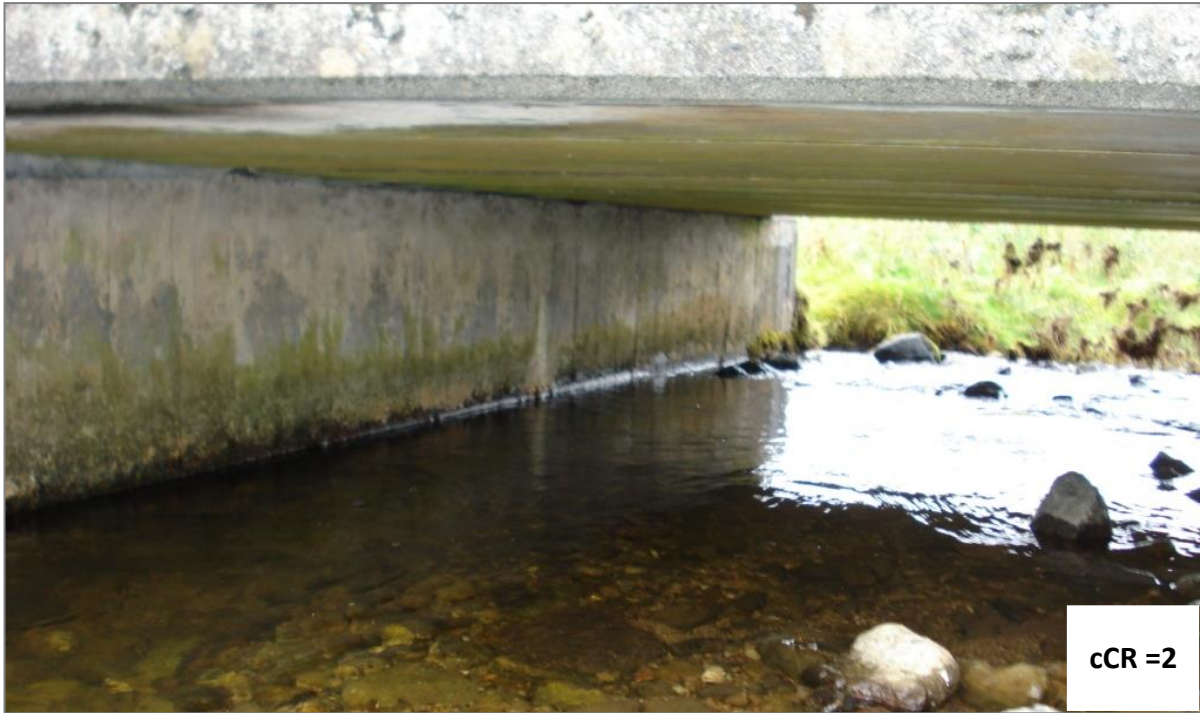
Figure A.37 – No Bearing Pads or Strips Evident.
