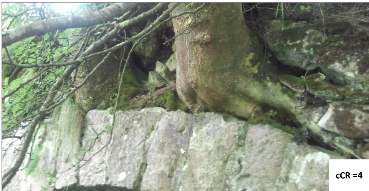
Figure A.20 – Tree Roots Boring into Barrel
