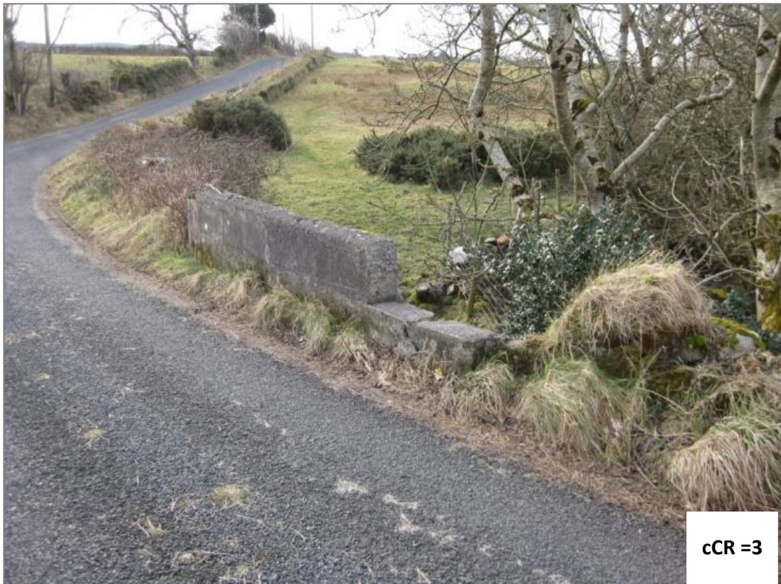
Figure A.4 – Concrete Parapet Partially Missing
