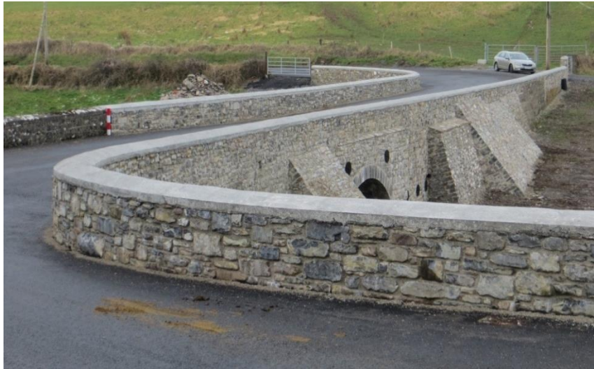
Figure 7.5 – Good Masonry Parapet Wall
