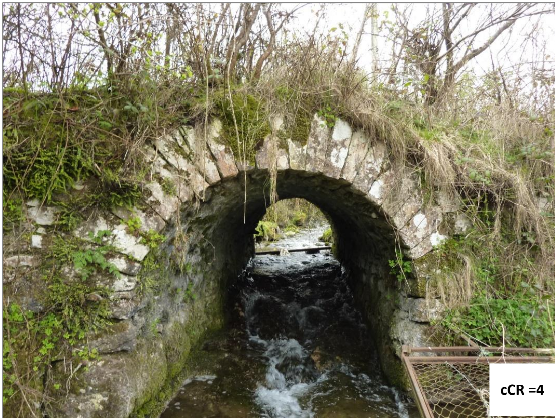
Figure A.7 – Missing Parapets and Spandrels
