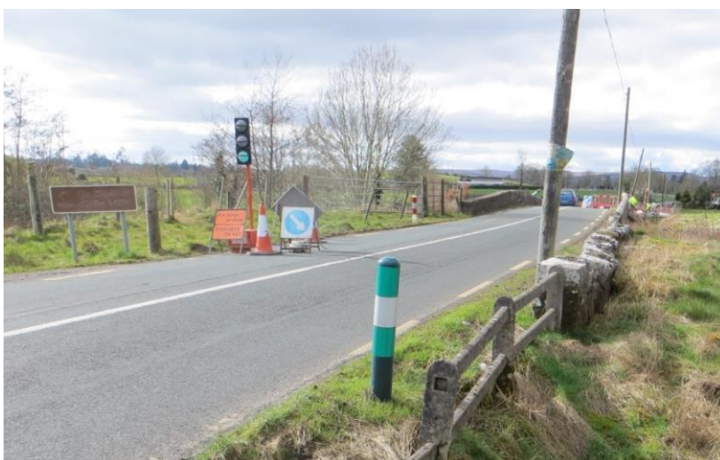
Figure 3.24 – Masonry Wall Not Part of Structure Length
