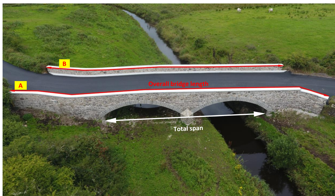
Figure 3.22 – Bridge in Elevation Depicting Overall Length and Total Span
