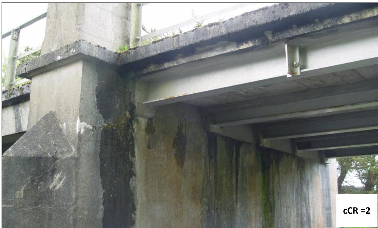
Figure A.28 – Water Seepage
