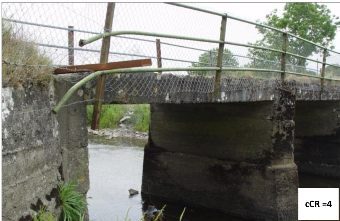
Figure A.6 – Broken Railing on Triple Span Bridge
