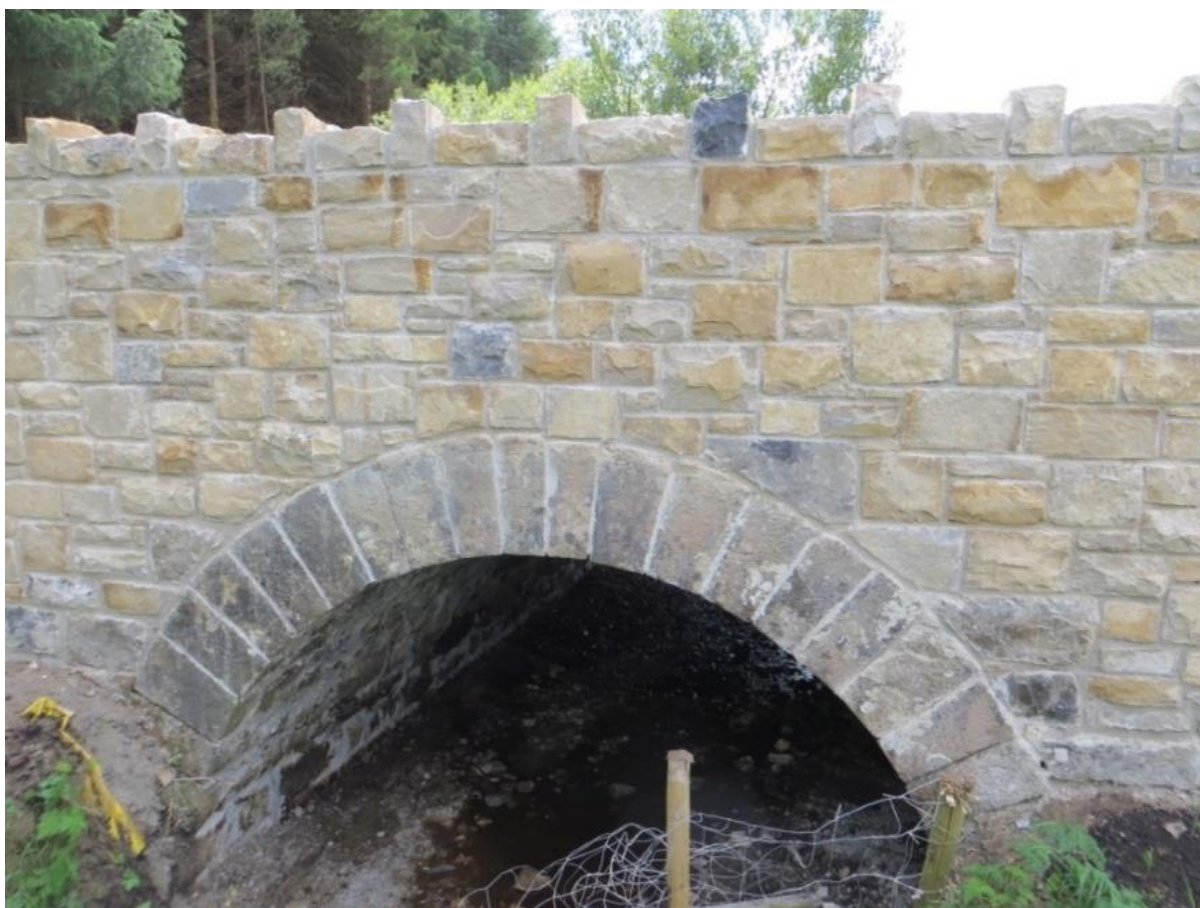
Figure 7.9 – Acceptable cut stone repair
