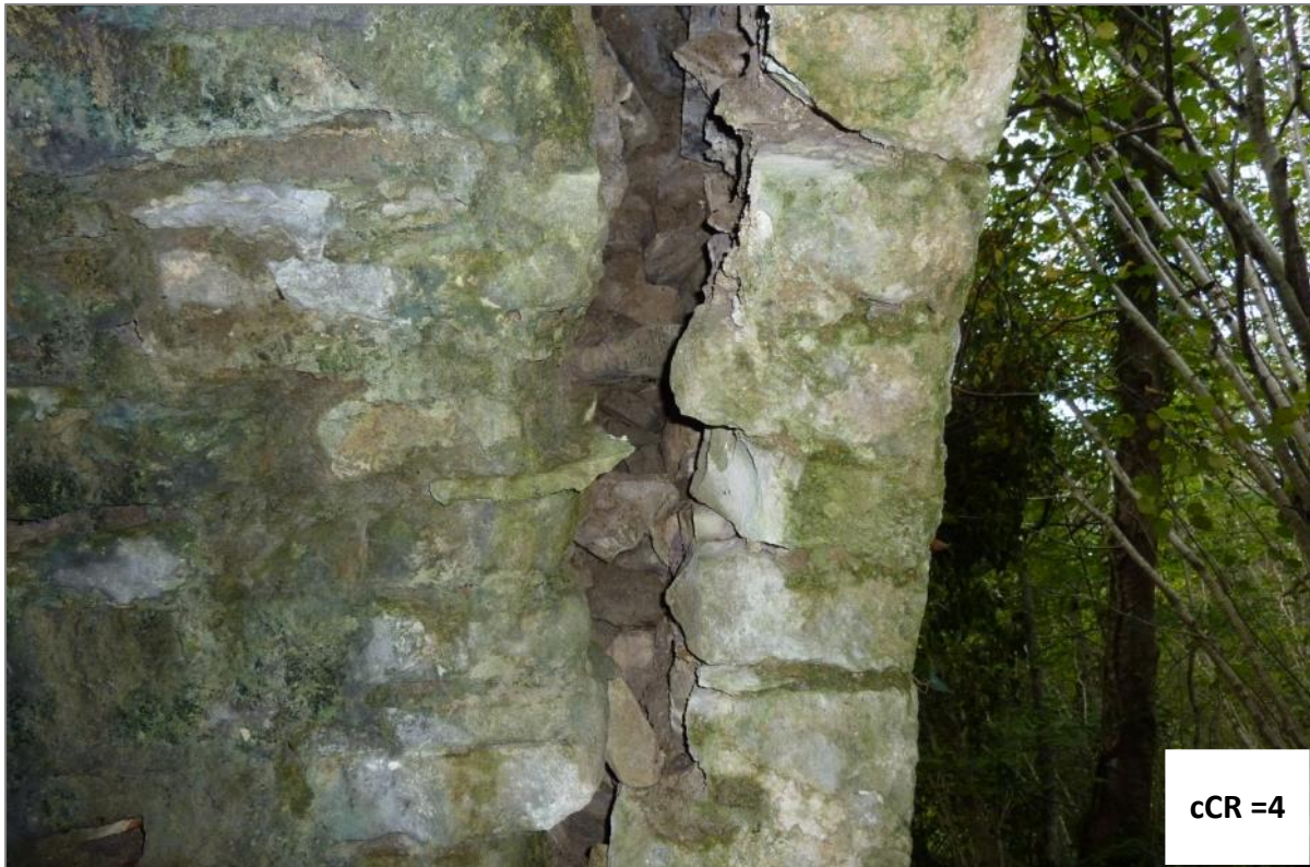
Figure A.26 – External Ring Isolation from Arch Barrel
