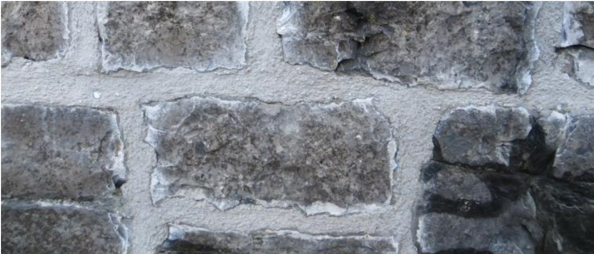
Figure 7.3 – Appropriate Lime Pointing
