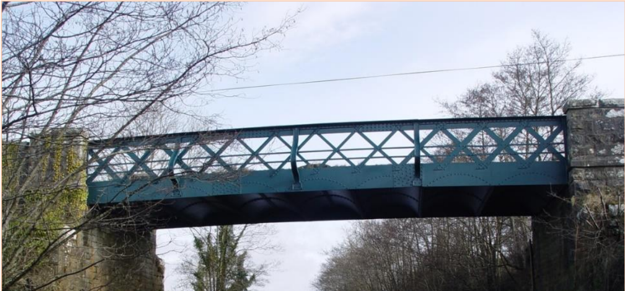
Wrought iron lattice girder 1881
