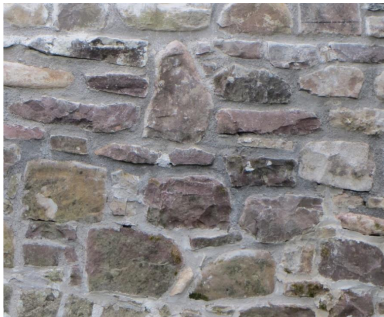
Figure 7.8 – Poor Quality Random-rubble Repair Work
