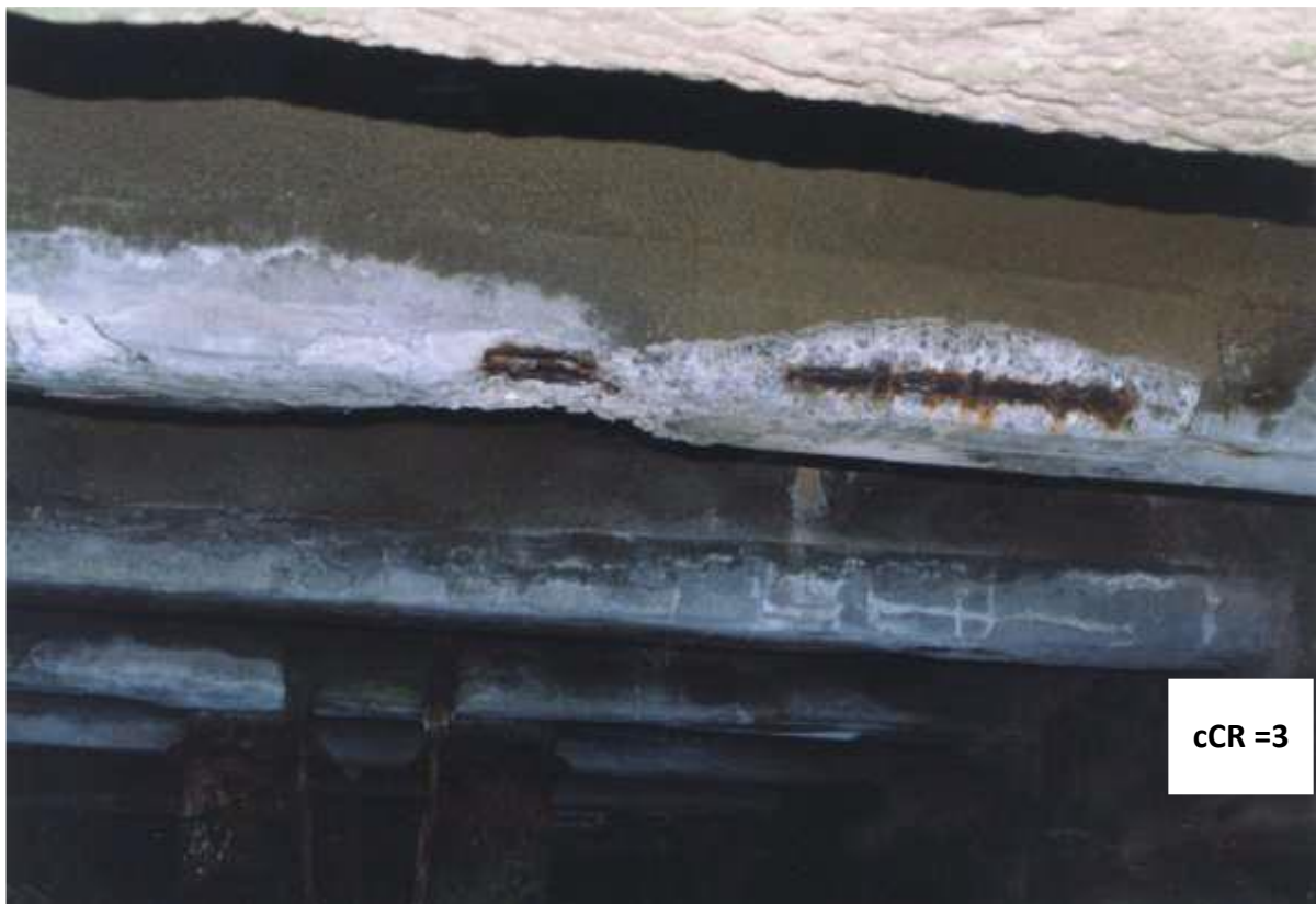
Figure A.29 – Main Reinforcement Rusting in Main Beam
