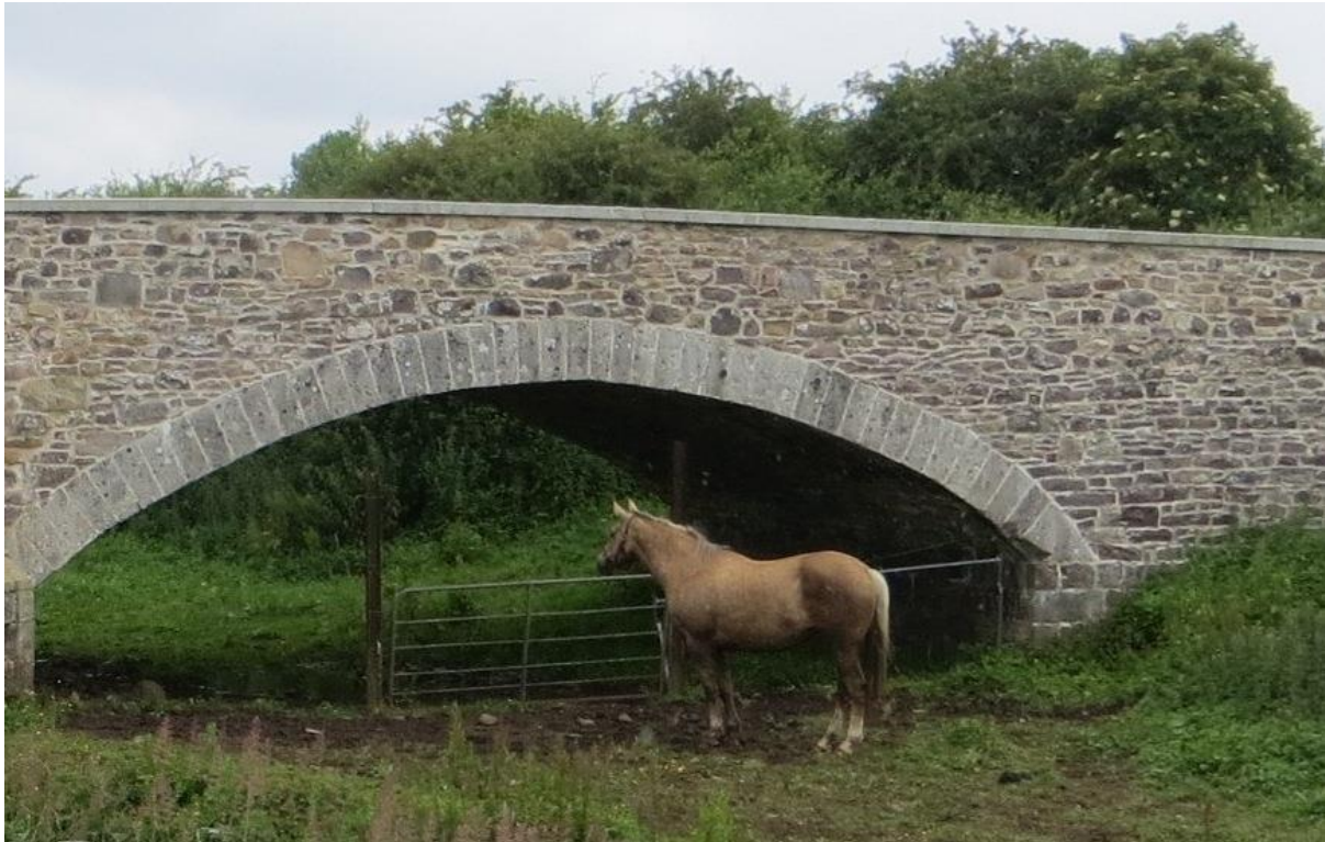
Figure 7.7 – Acceptable Random-rubble Repair Work
