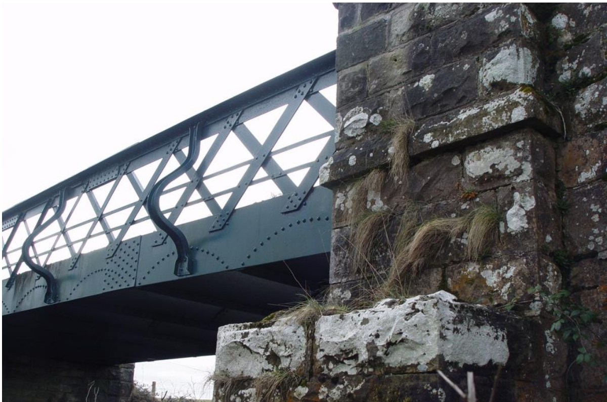
Figure 7.10 – Wrought Iron Bridge
