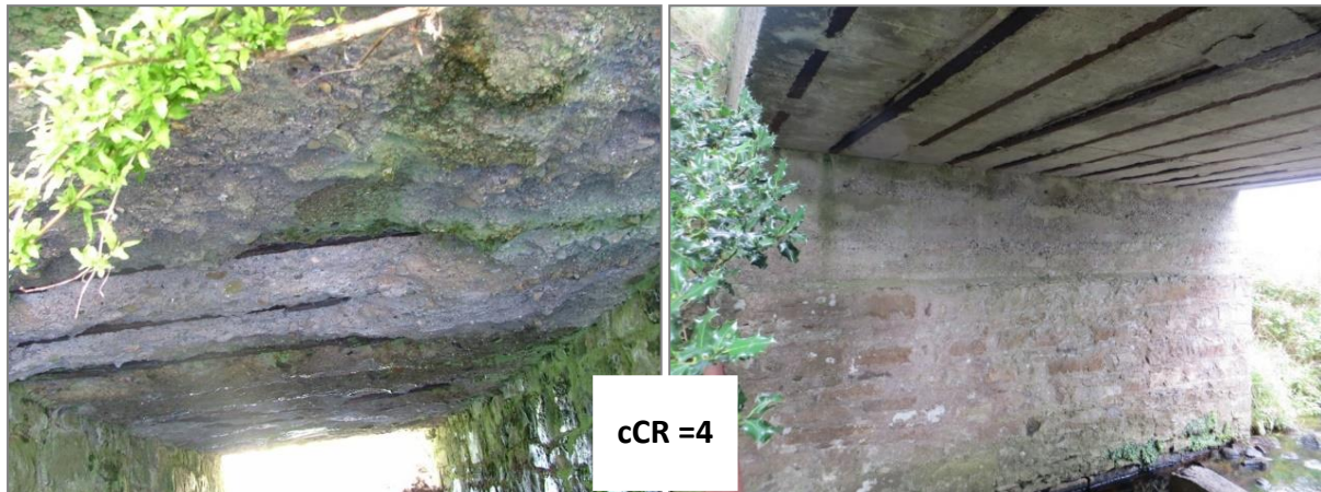
Figure A.32 – Compromised Flanges
