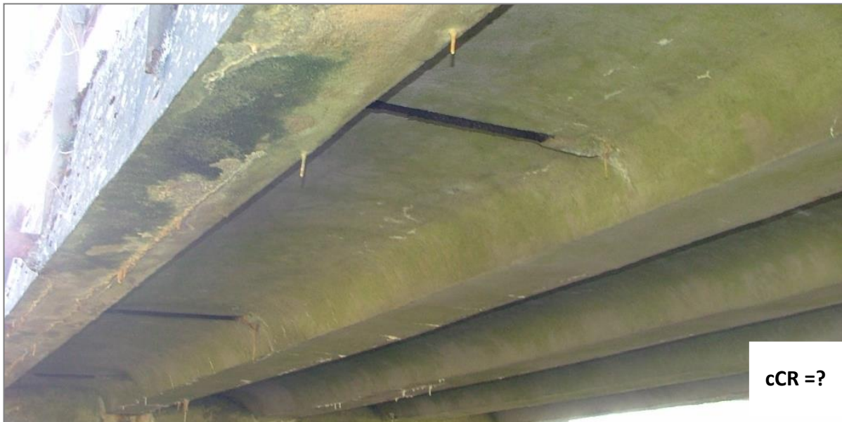
Figure A.27 – Cracks in Soffit
