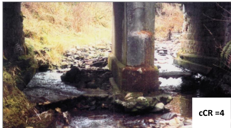
Figure A.35 – Bed Protection Failure
