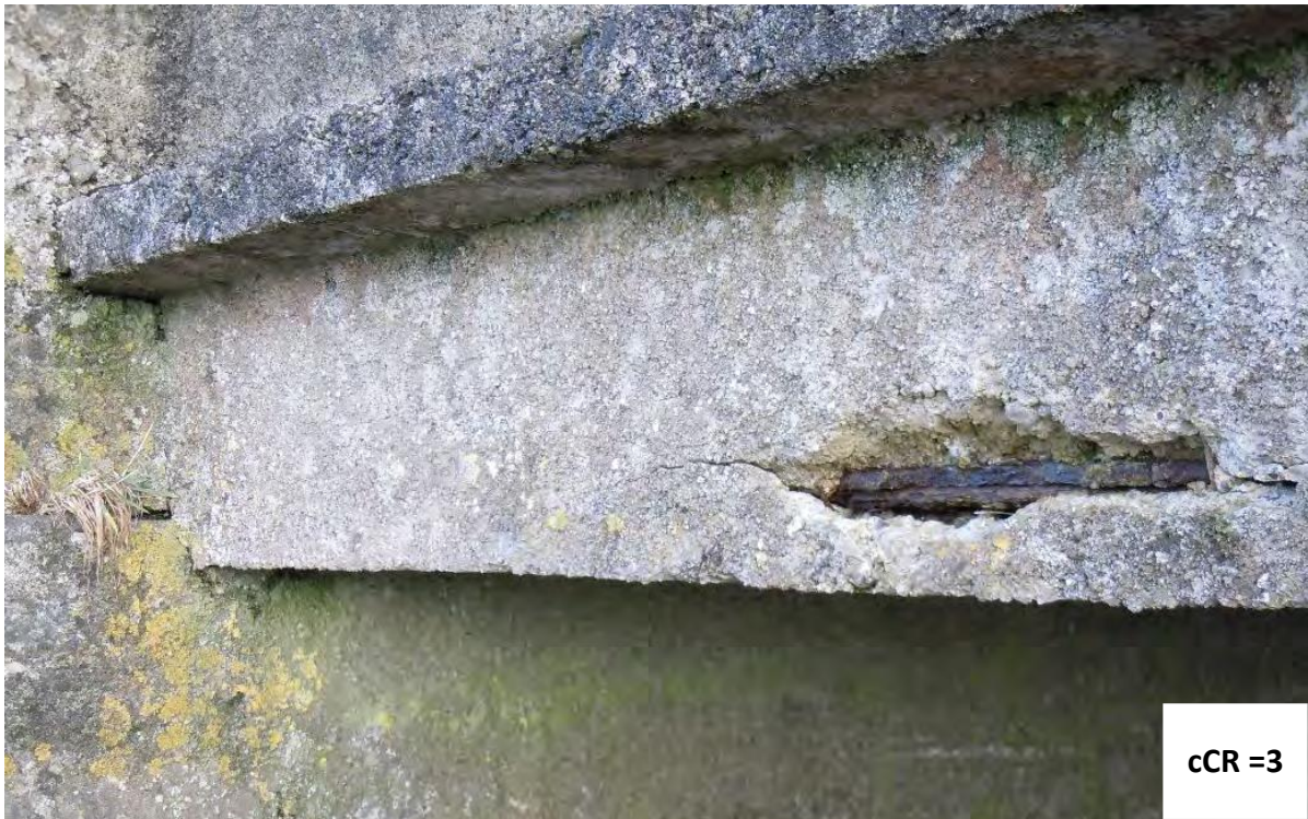
Figure A.30 – Exposed Steel Flange
