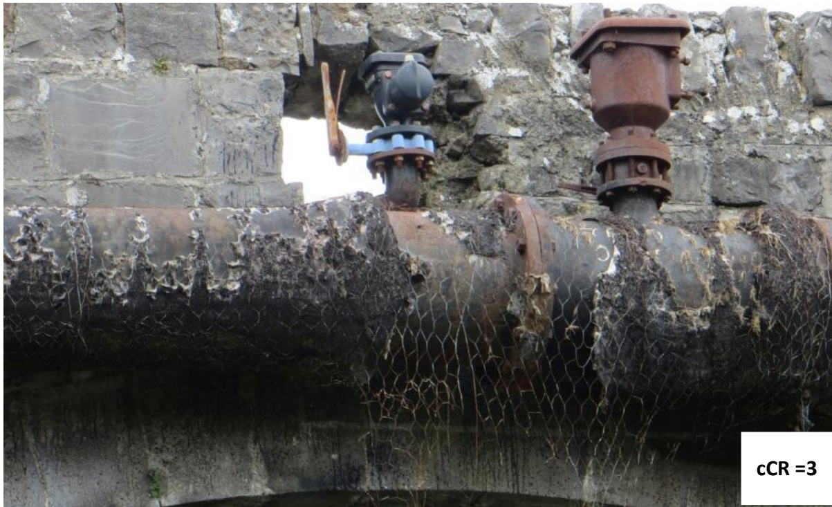
Figure A.45 – Inconsiderate treatment of Protected Bridge by service designers and installers.
