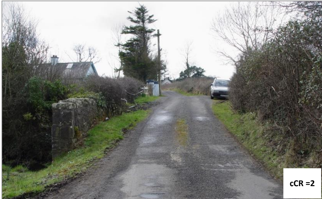
Figure A.3 – Grass Verges and Hedge Growth in Verge and Parapet
