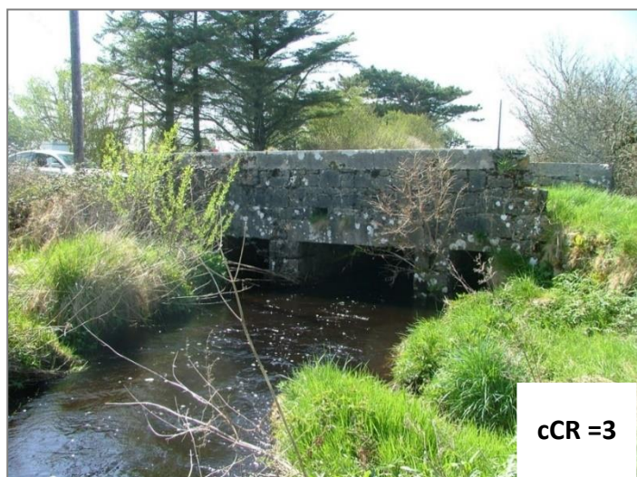
Figure A.31 – Compromised Concrete Slab Deck
