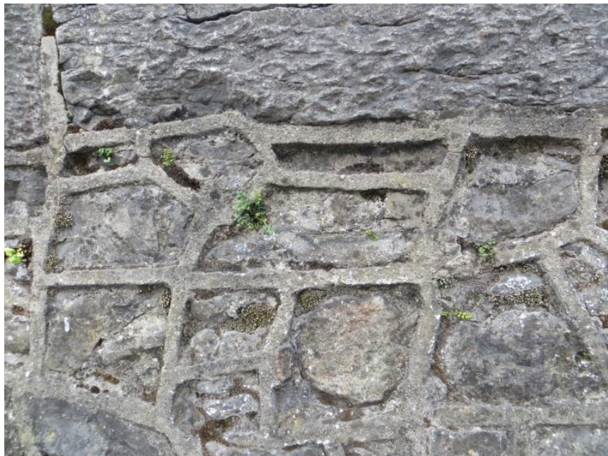
Figure 7.4 – Inappropriate opc 'strap' Pointing
