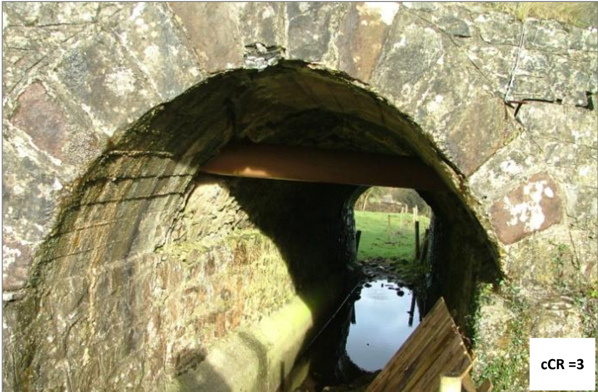
Figure A.43 – Services Causing Damage
