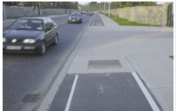
Incomplete marking of cycletrack at vehicle access
