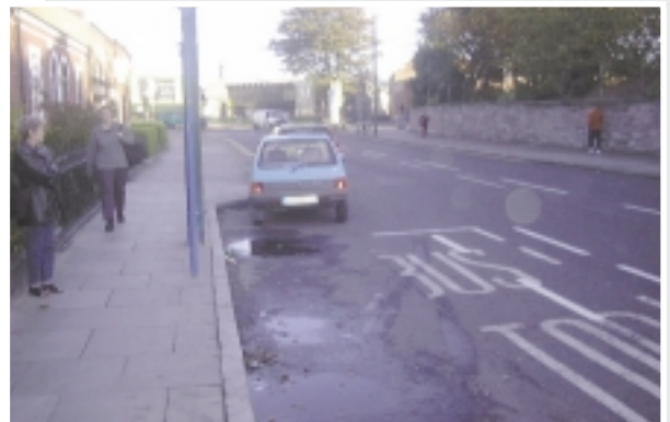
Example of poor design
