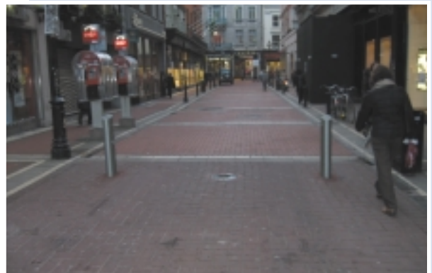
Rising bollard to restrict access
