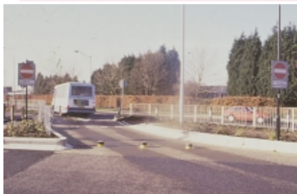
Rising bollard at bus only entry
