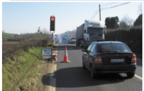
Temporary traffic signal control
