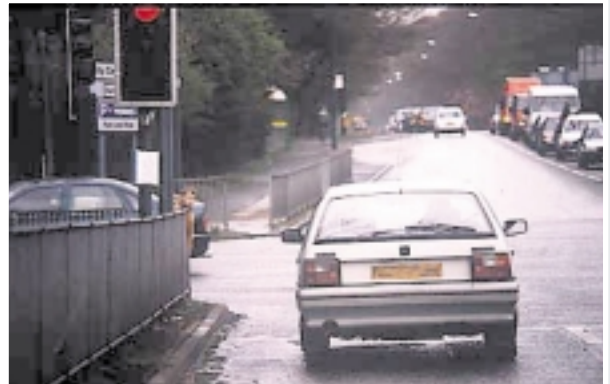
Guard Rail blocks visibility
