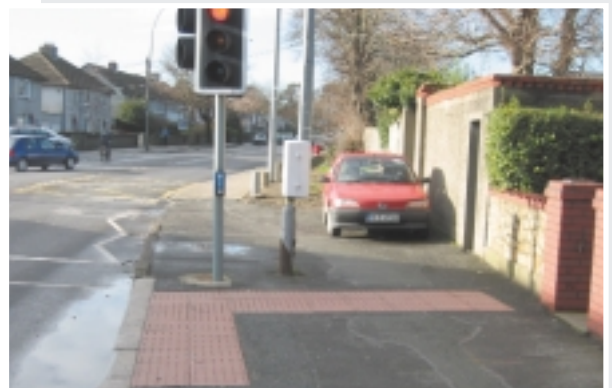
Tactile paving slabs
