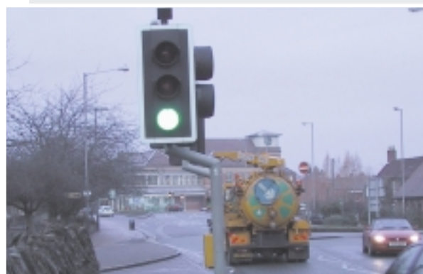
Cranked signal poles allow push buttons to be sited close to the crossing and provide clearance from passing vehicles without obstructing the footway
